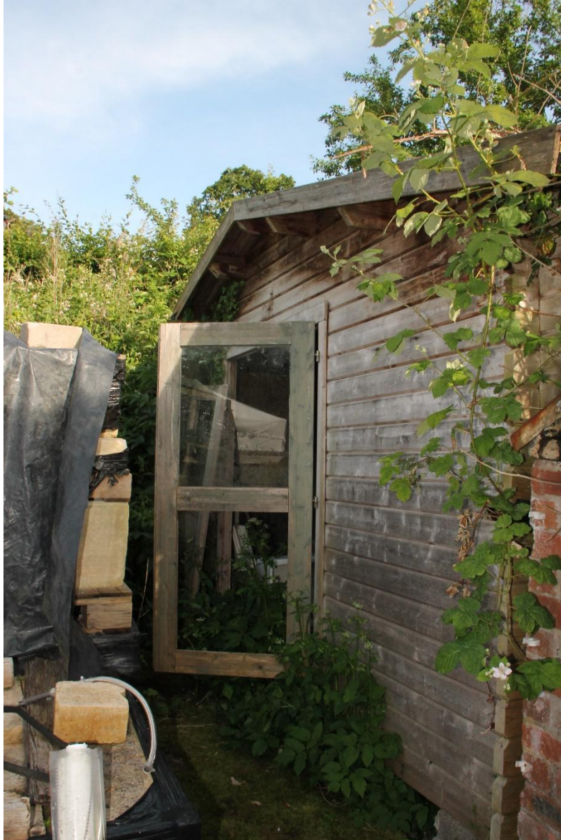
Photograph 5: showing a view of Building 3
