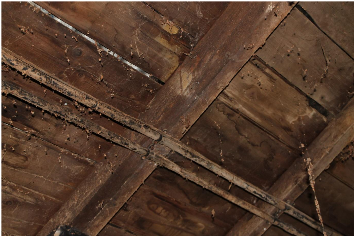
Photograph 4: showing a view of the internal roof of Building 2
