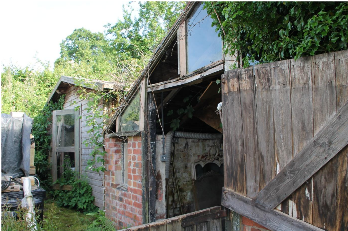
Photograph 3: showing a view of Building 2
