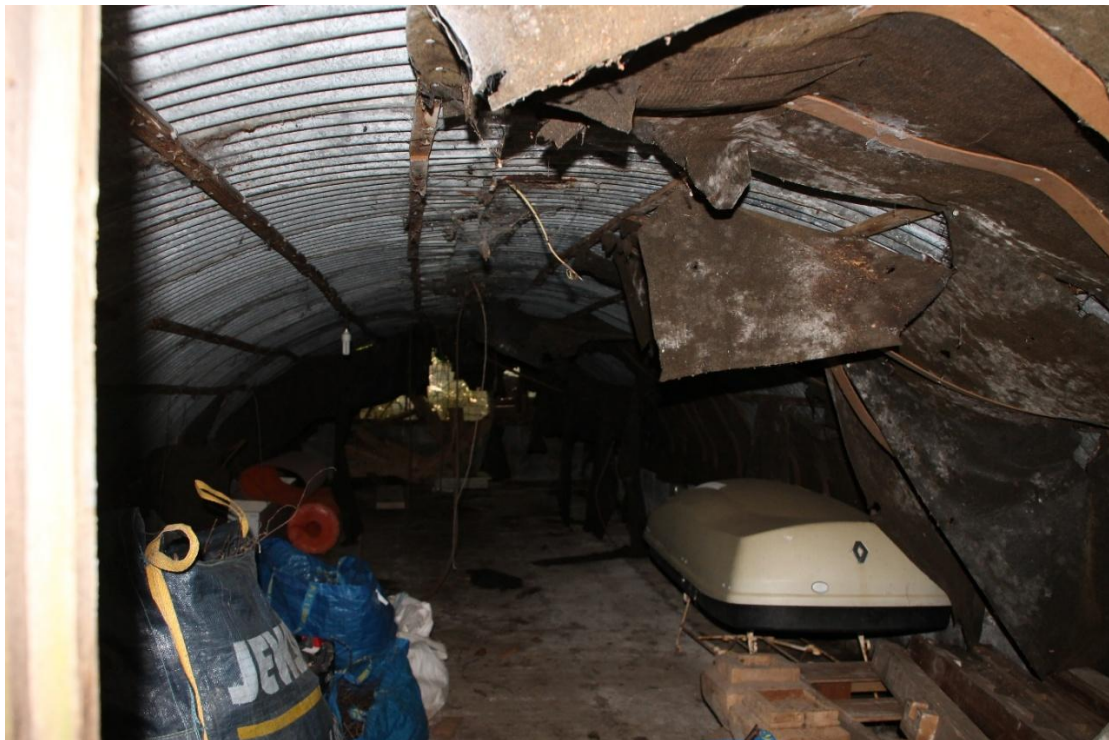
Photograph 2: showing a view of inside of Building 1
