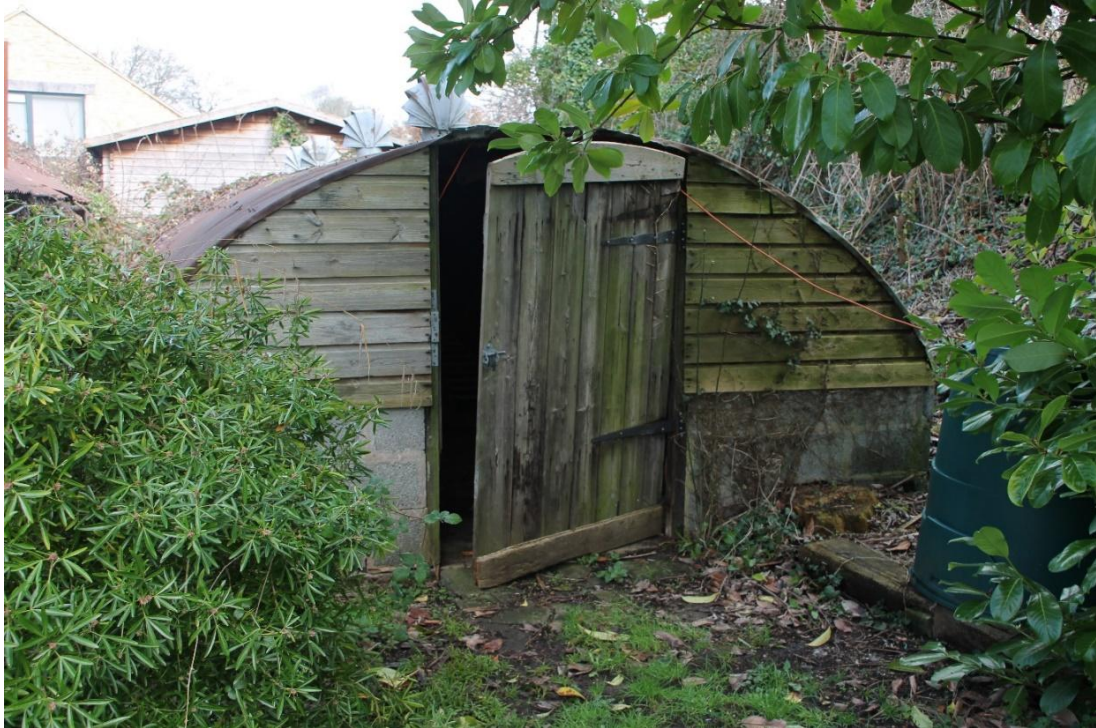
Photograph 1: showing a view of Building 1
