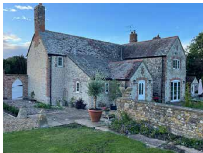
Fig 6 Combination of lean to, gable and porch added in 1987.
