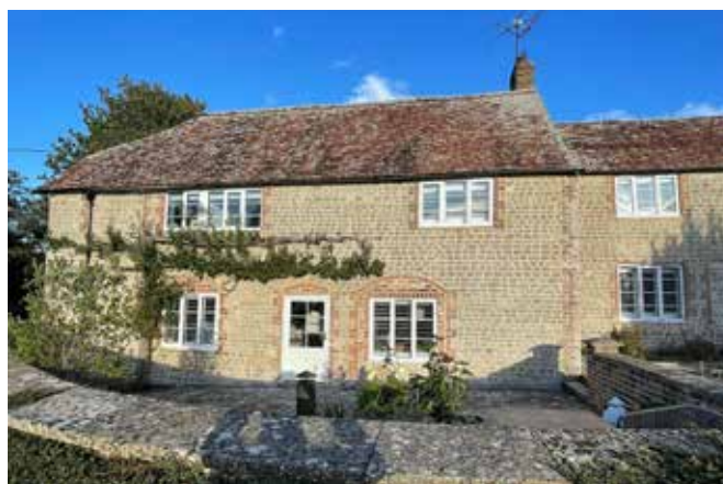
Fig 7 West elevation showing conjoined windows on first floor to be reinstated. Note door has been reinstated PL/2025/04445
