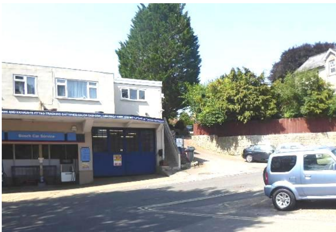
Fig 5.1.1: Ground slopes around the site
