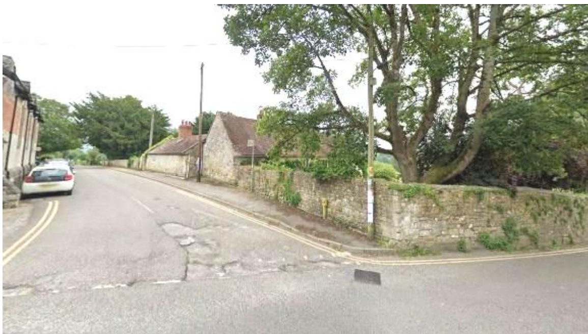
Fig 5.1.9: Gaston Manor and its boundary wall, as seen from the forecourt of Tisbury Motors
