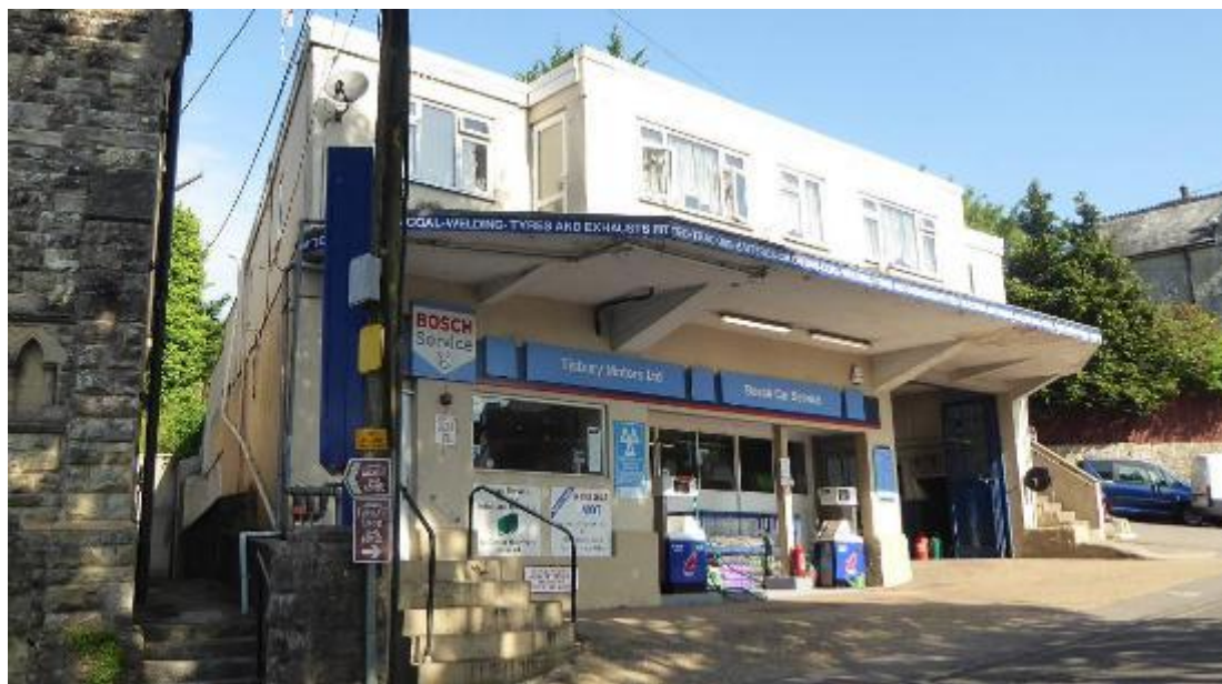
Fig: Tisbury Motors from the southeast
