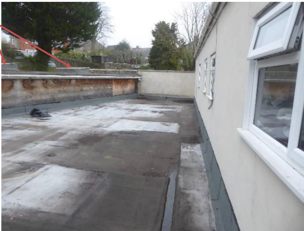
Fig 2.3.4: Roof terrace at the rear (west) of the flat
