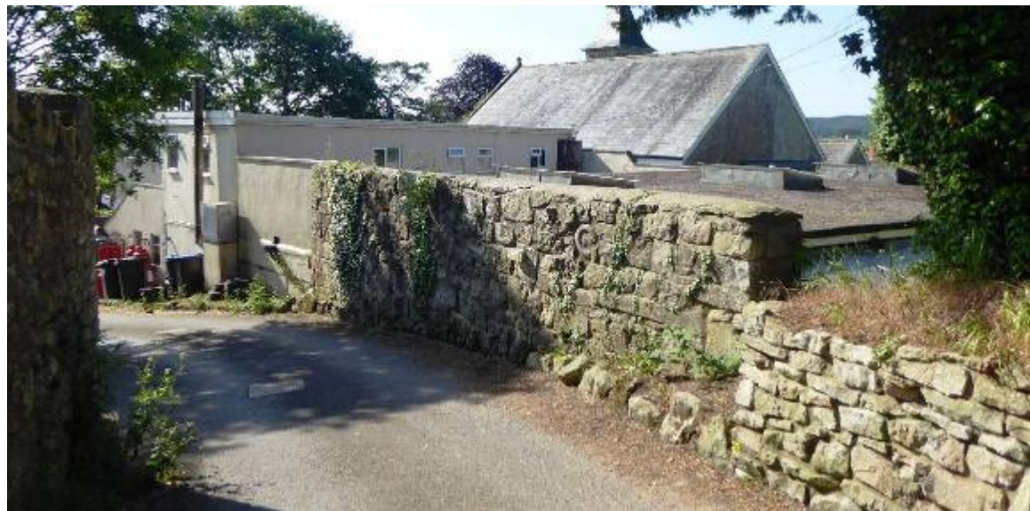
Fig 2.2.3: The rear of the garage, with 20 th walls to the access lane
