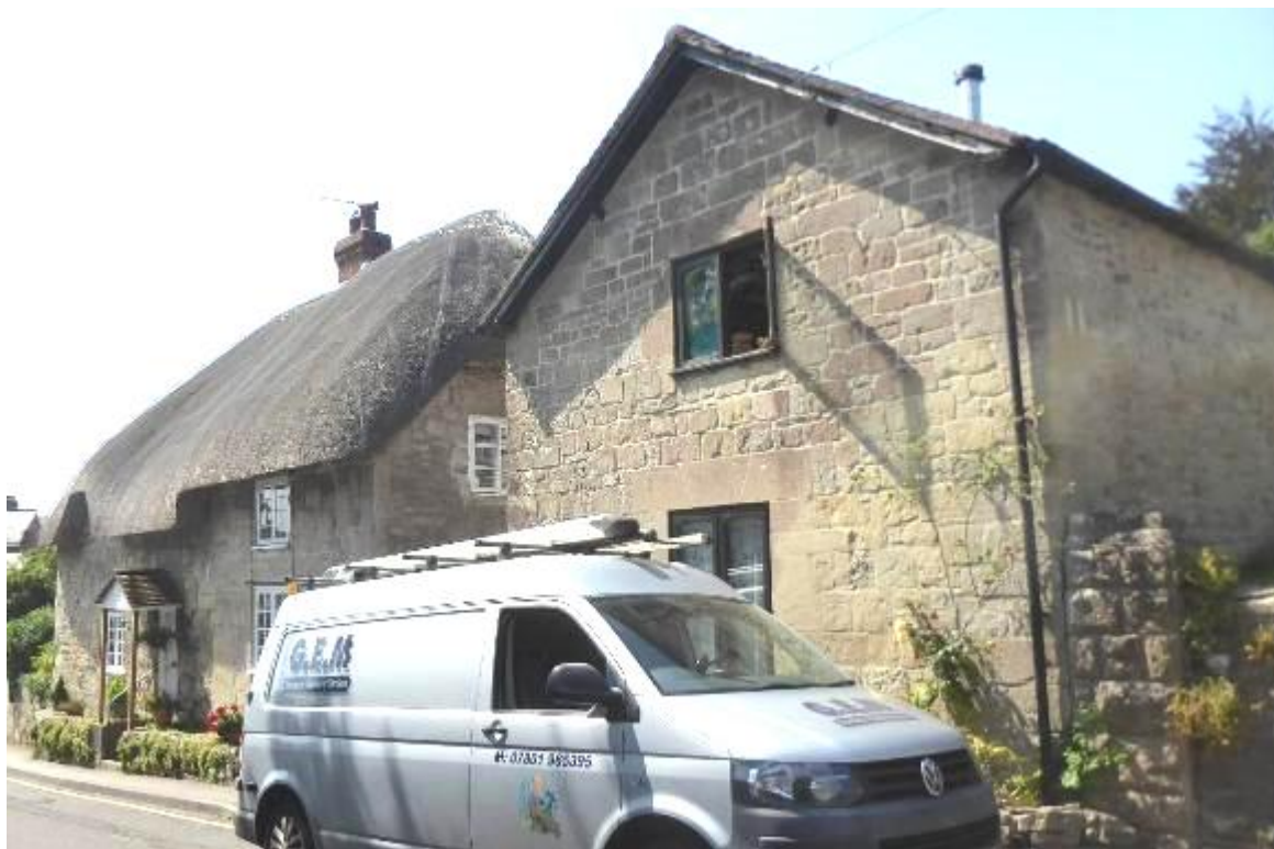
Fig 5.1.3: Residential dwellings to the south of the chapel
