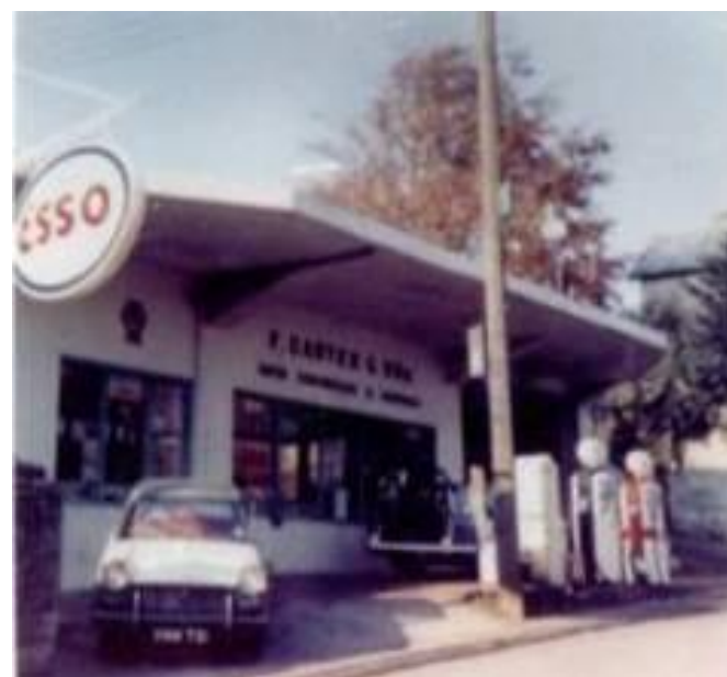
Fig 3.2.2: The garage in the 1950s
