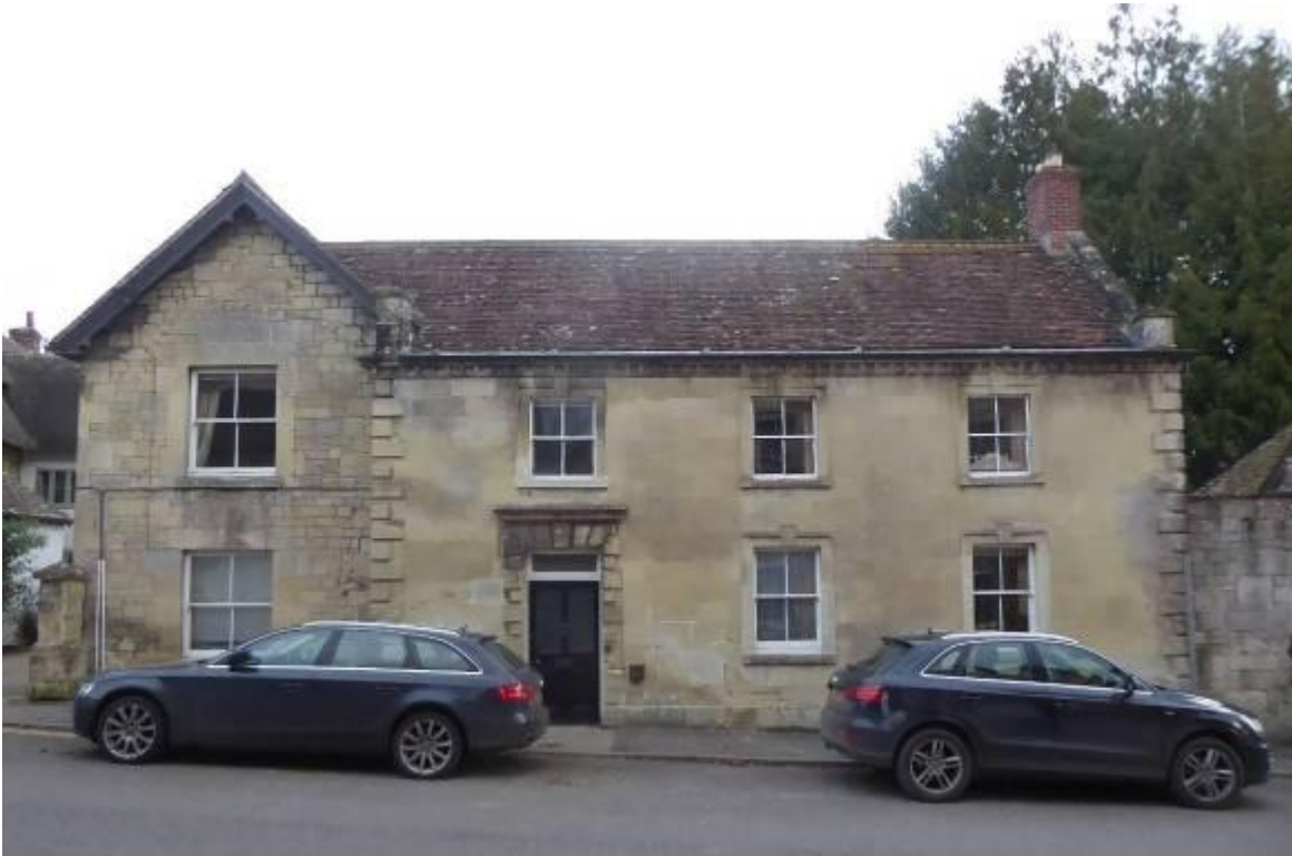
Picture 18: Ashlar facade on the east side of the High Street
