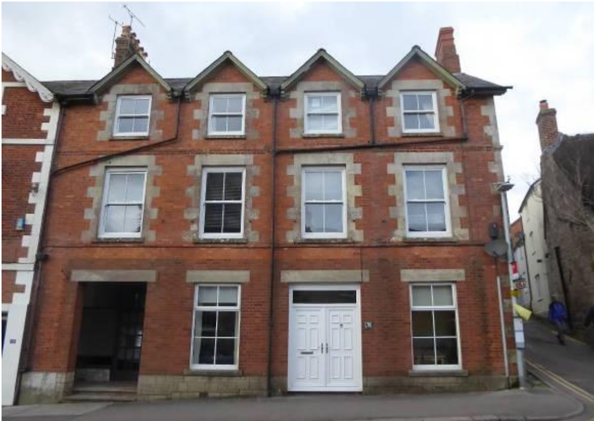
Picture 16: Terrace running north of Tisbury Motors continued
