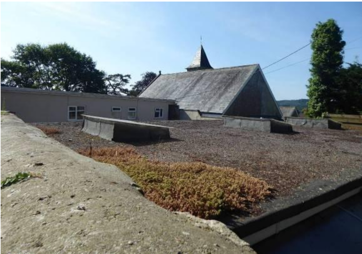
Picture 6: View across Tisbury Motors roof looking southeast
