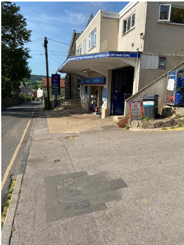
Front elevation looking south, view of station forecourt and fuel tanks
