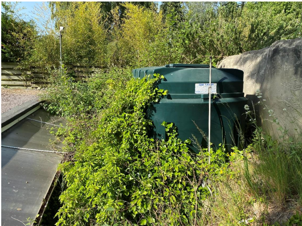
Oil tank at top of retaining wall – middle of the site
