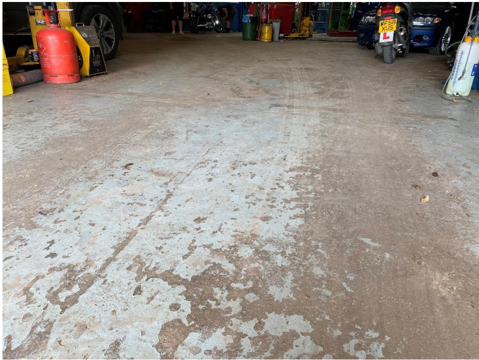
Existing slab within workshop
