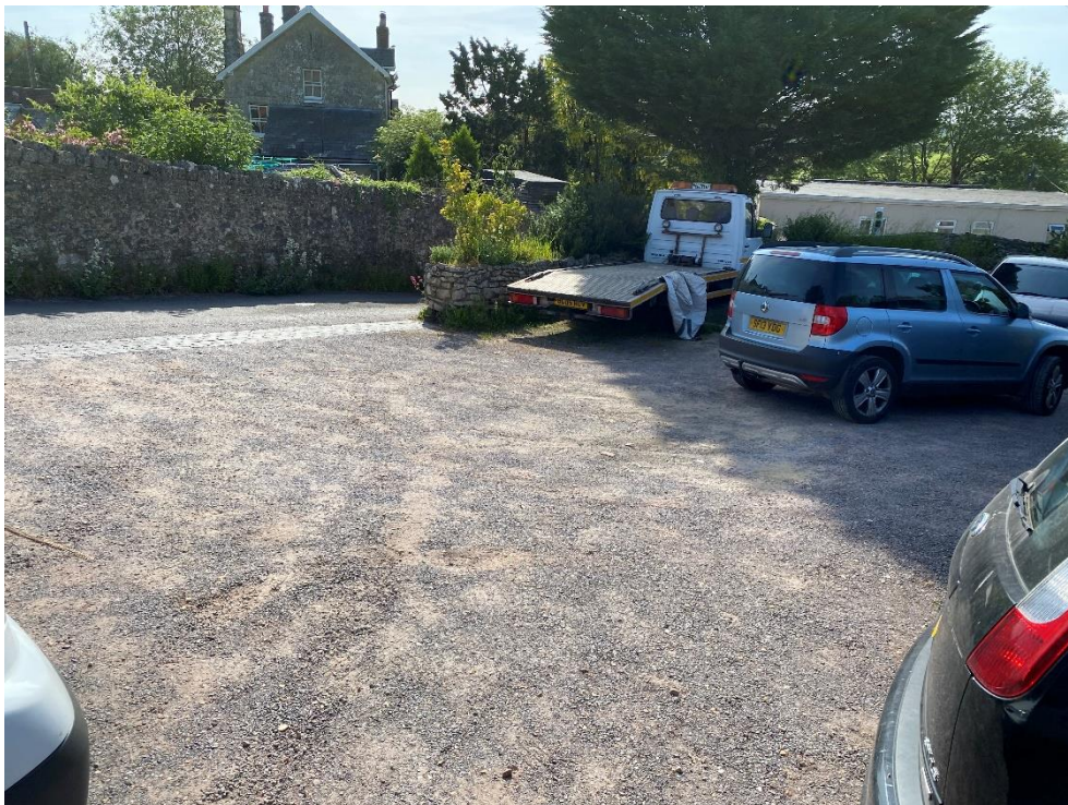
Gravel car parking surfacing
