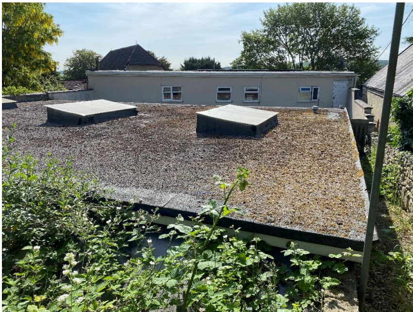
Single storey extension to rear of 2 storey main building
