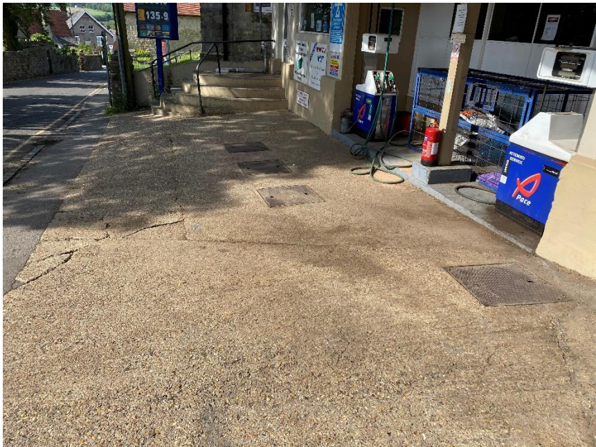
Front elevation looking south, view of station forecourt and fuel tanks
