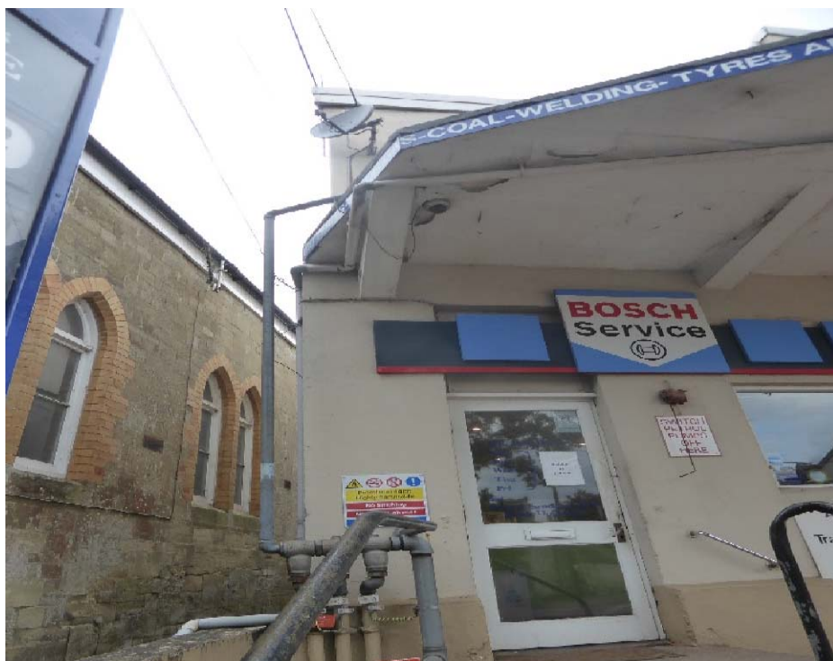
Existing Canopy Drainage Outlet and Additional Roof Downpipe on Southern Side of Building
