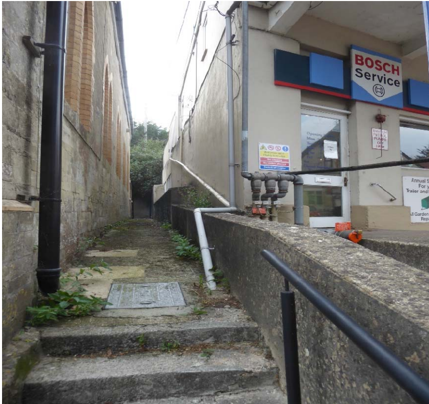
Downpipe From Site Entering an Existing Private Combined Inspection Chamber adjacent to the Neighbouring Church
