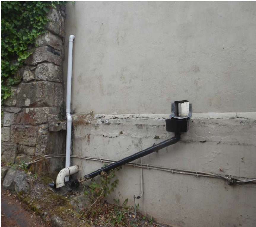
Combined Gully Adjacent to North Wall
