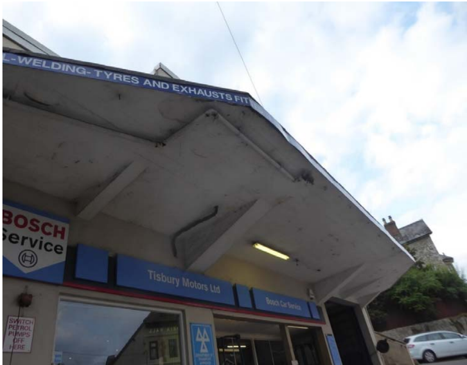
Existing Roof Drainage Outlet Through Canopy
