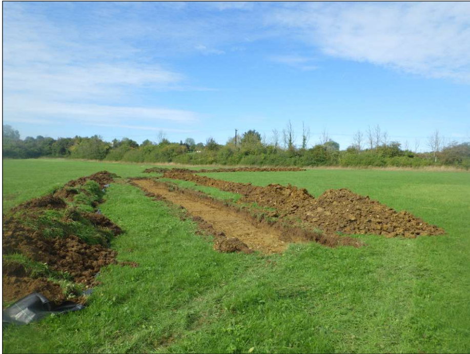
Plate 1: Western parcel of land, with Trench 2 in the foreground and Trench 1 beyond, looking northwest
