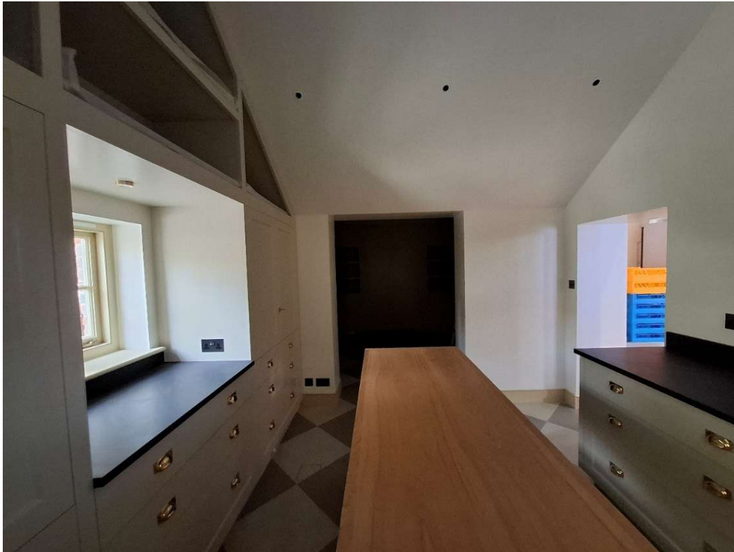
Figure 5 New doorway shown on G04 side - after woks completed
