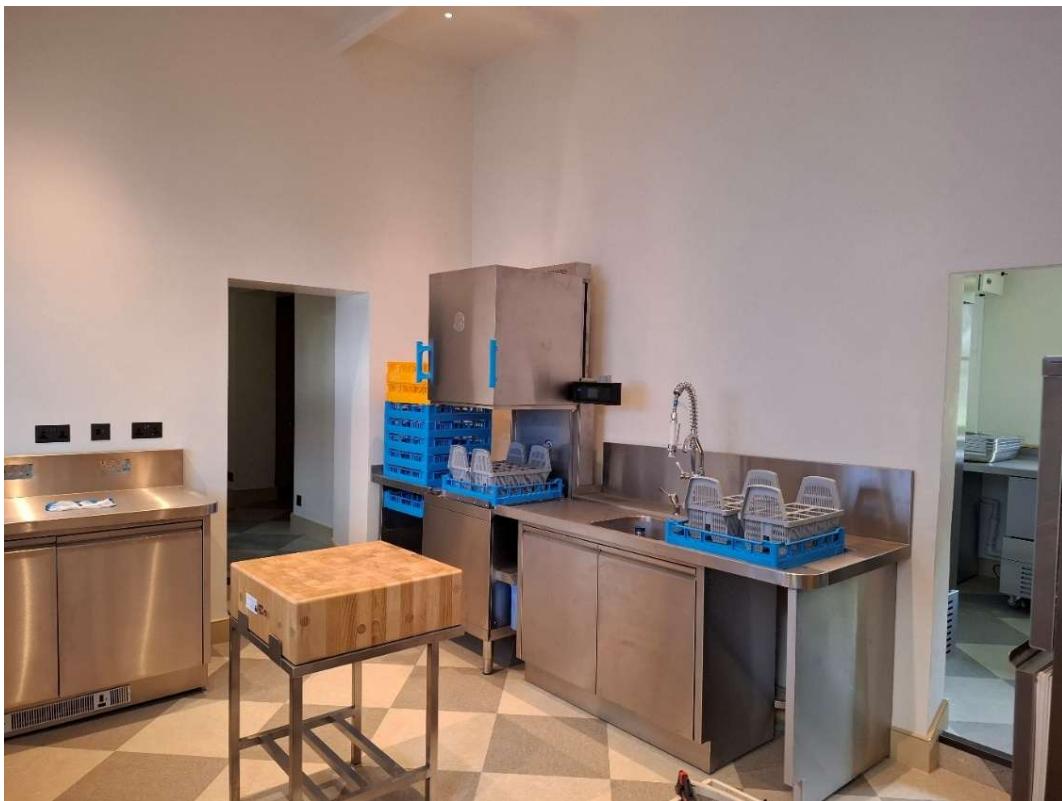
Figure 6 New doorway shown on G01 side - woks completed
