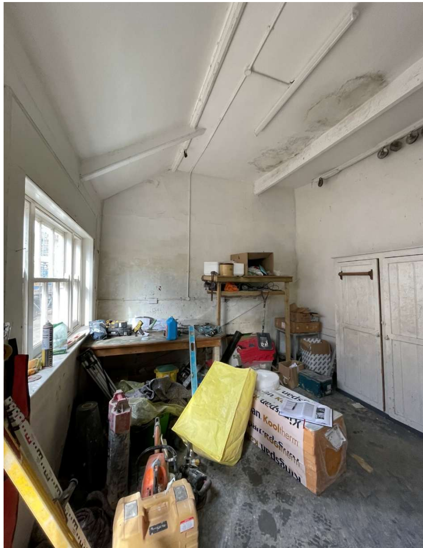
Figure 2 Wall separating (A1)G04 and (A1)G01- G01 side - before refurbishment works commenced
