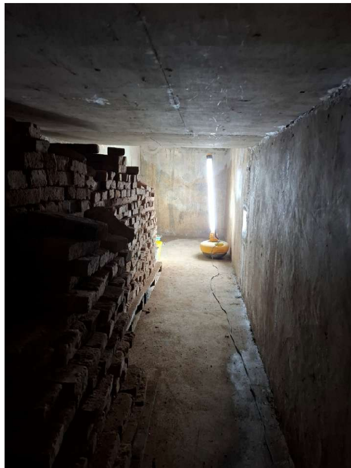
Figure 3 Image shows existing structures with newly cast lid - Picture taken looking towards the bottom of the tunnel
