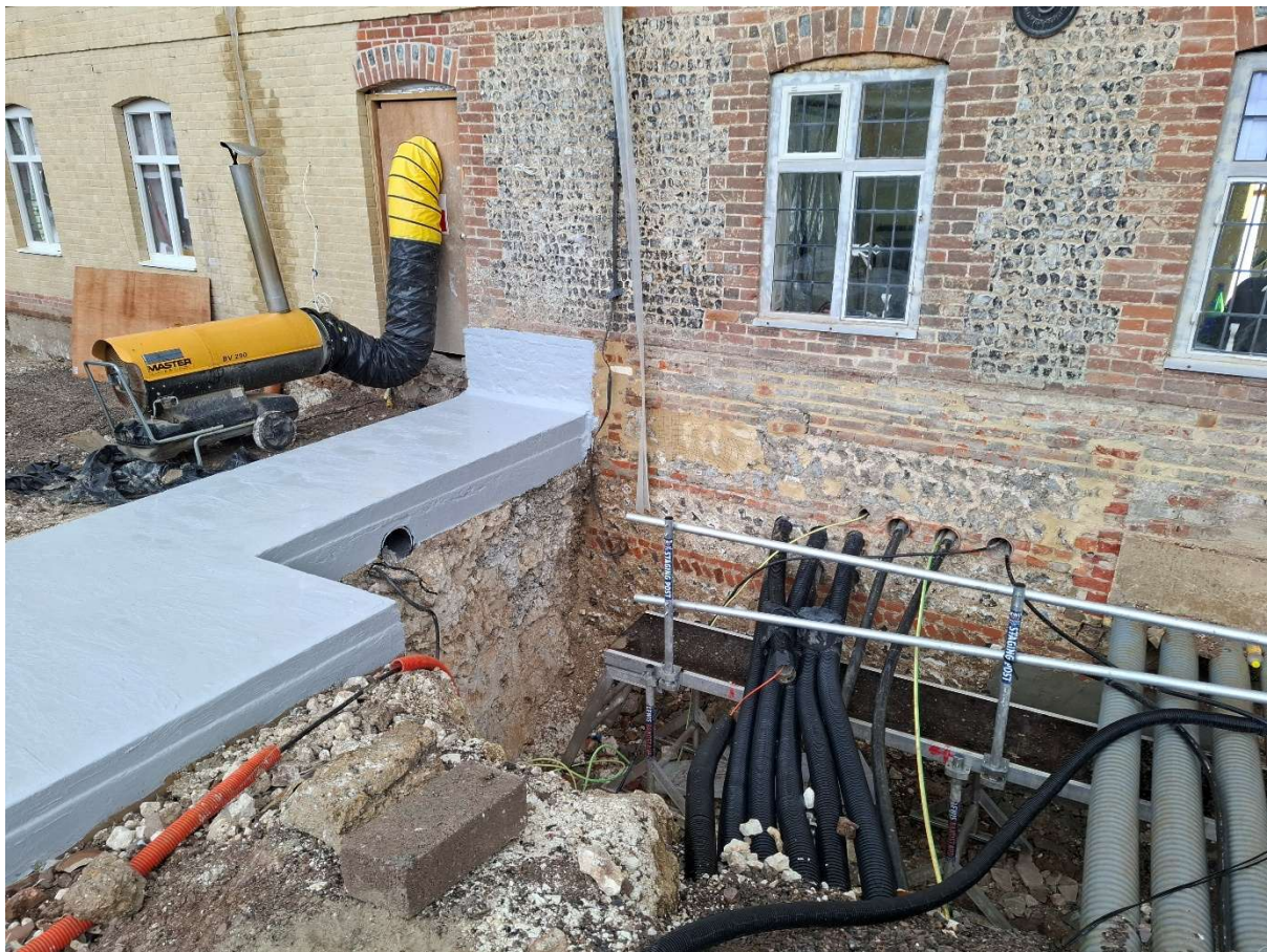
Figure 6 image shows existing and new lid while receiving waterproofing coating. Retained structures are also visible
