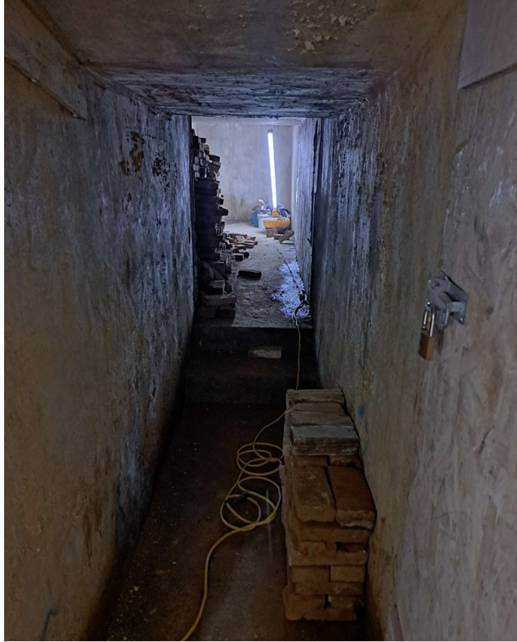
Figure 4 Image shows existing structures with newly cast lid - Picture taken from access point within House's basement
