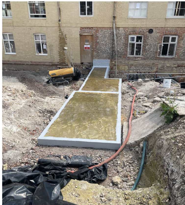
Figure 5 image shows existing and new lid while receiving waterproofing coating
