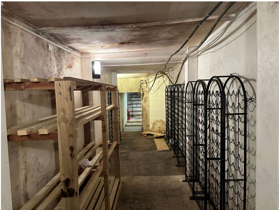
Figure 1 Image shows conditions of existing modern linings before refurbished works commenced
