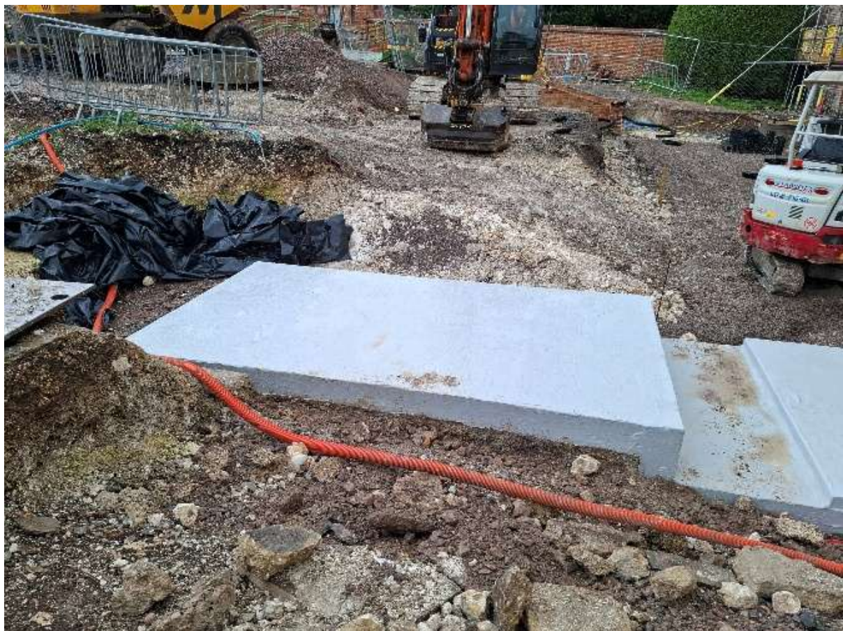
Figure 7 image shows existing and new lid after receiving waterproofing coating
