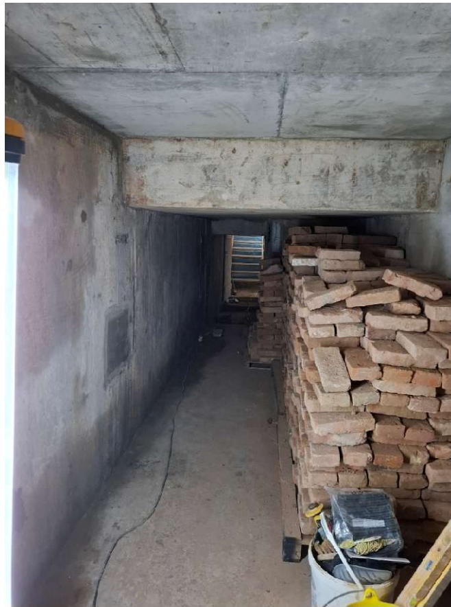
Figure 2 Image shows existing structures with newly cast lid - Picture taken from the bottom of the tunnel looking towards access from the House's basement
