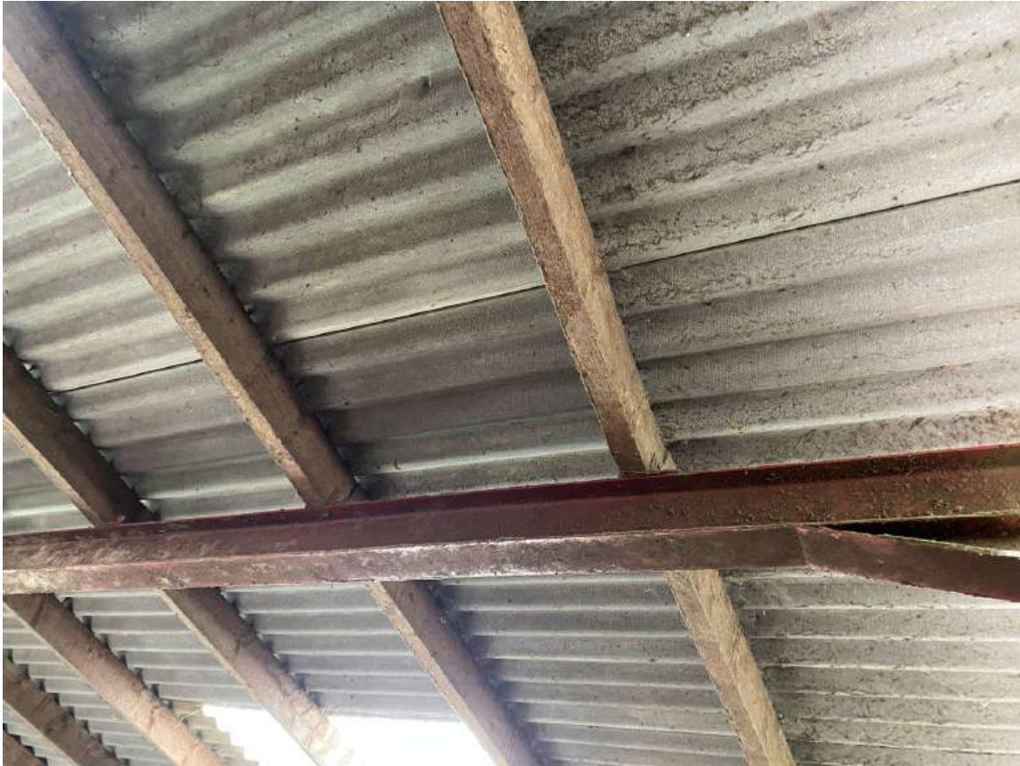
Figure 1.12– Principal rafter and purlin connection
