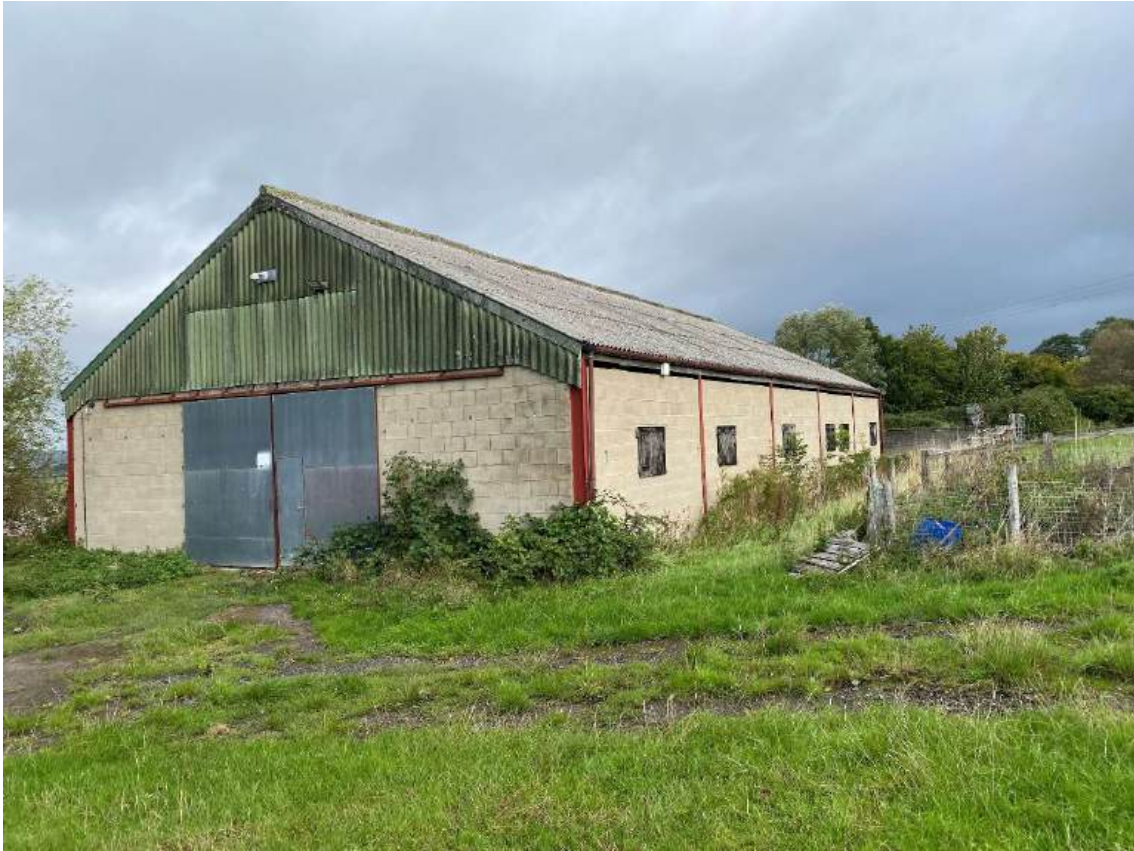
Figure 1.5 – Rear Elevation next field
