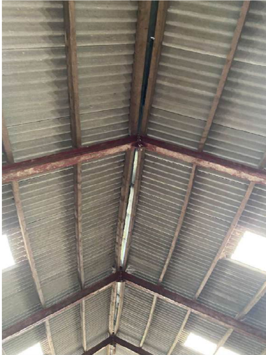
Figure 1.10 – Underside of roof ridge
