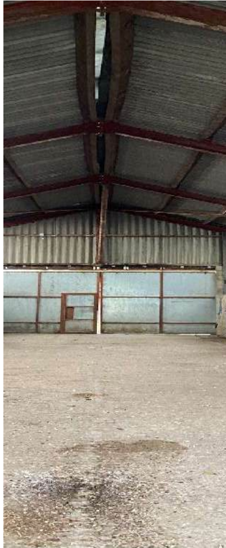
Figure 1.6 Internal roof structure
