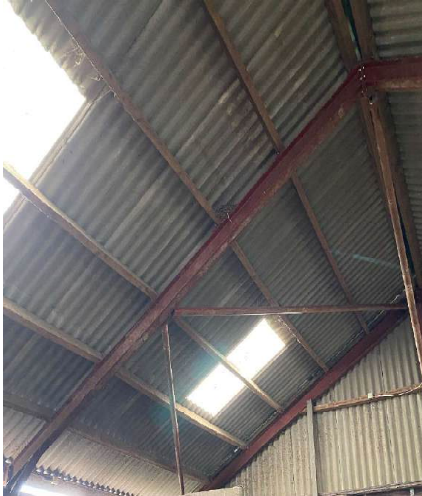
Figure 1.7– Portal Frame bracing
