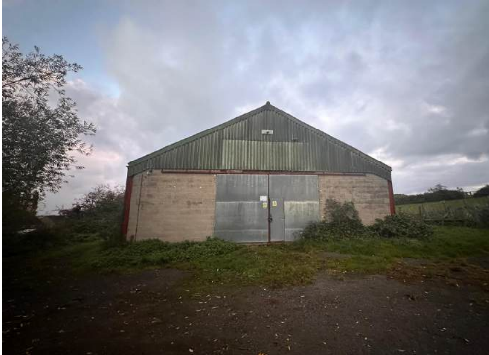
Figure 1.1 (Barn at Lifely Farm, West Ashton, Trowbridge)
