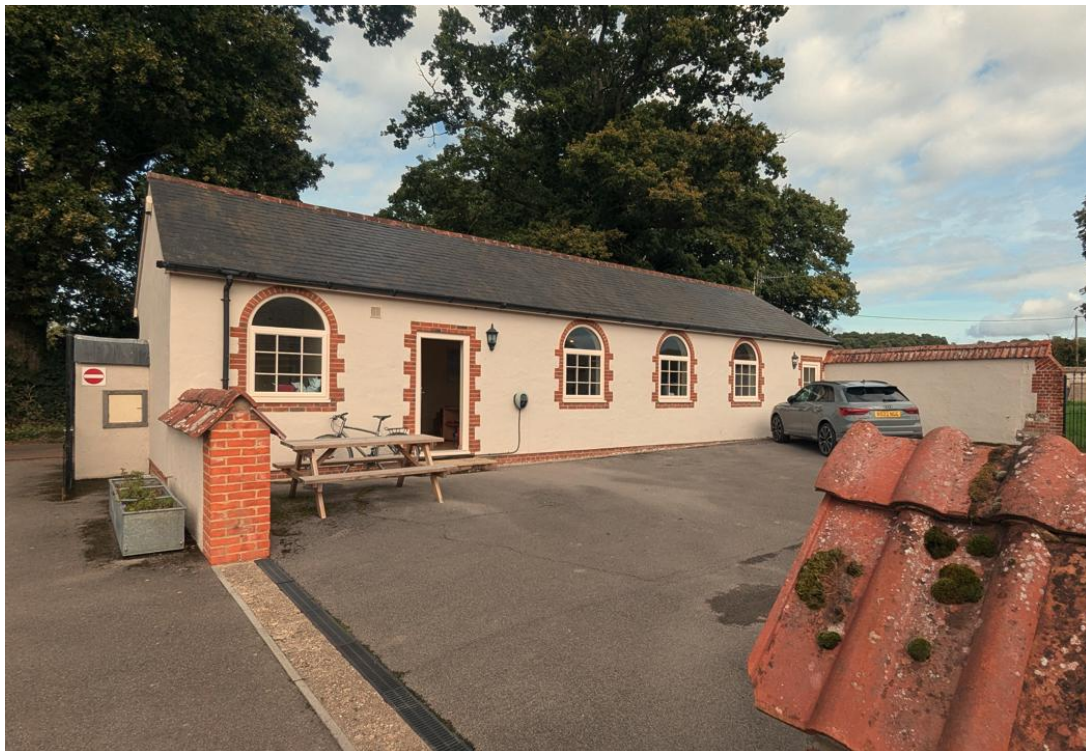
Figure 2 - Front elevation of Building 2 with parking in front
