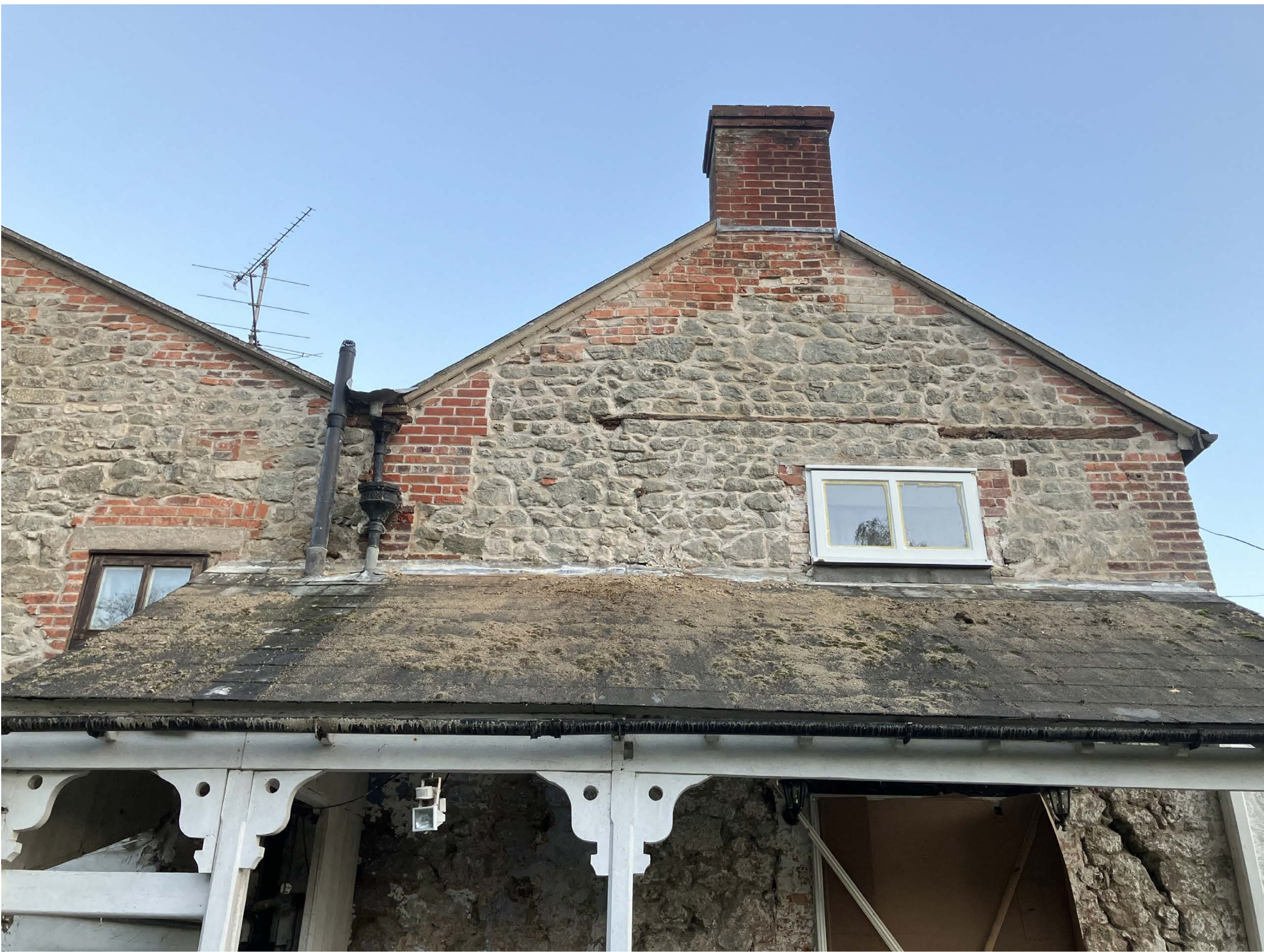
Images show existing pointing on rear wall. All new pointing will be mixed on-site to match the colour and appearance of he existing mortar. Pointing method/style between bricks and stone will match existing on-site.
