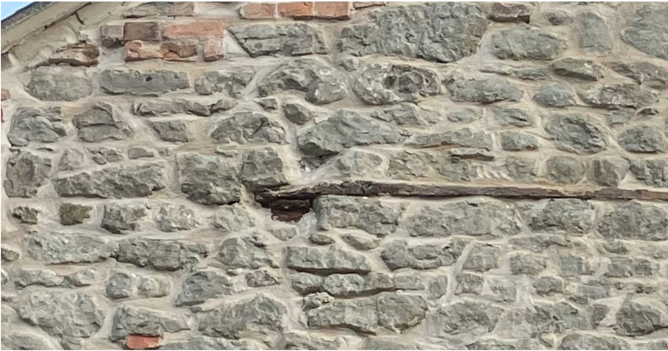
Images show existing pointing on rear wall. All new pointing will be mixed on-site to match the colour and appearance of he existing mortar. Pointing method/style between bricks and stone will match existing on-site.
