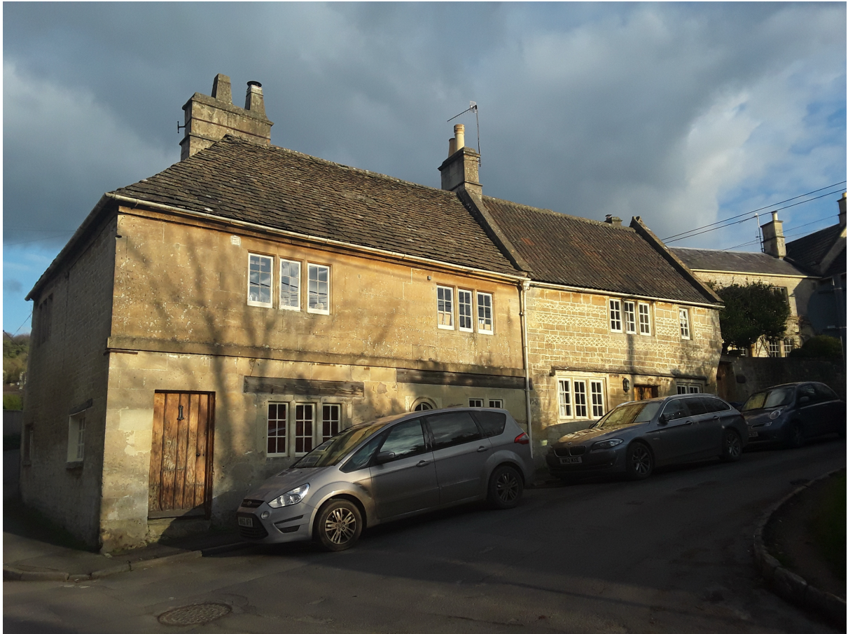
existing photograph of front elevation (Laker, J., Historic England, 2018)
