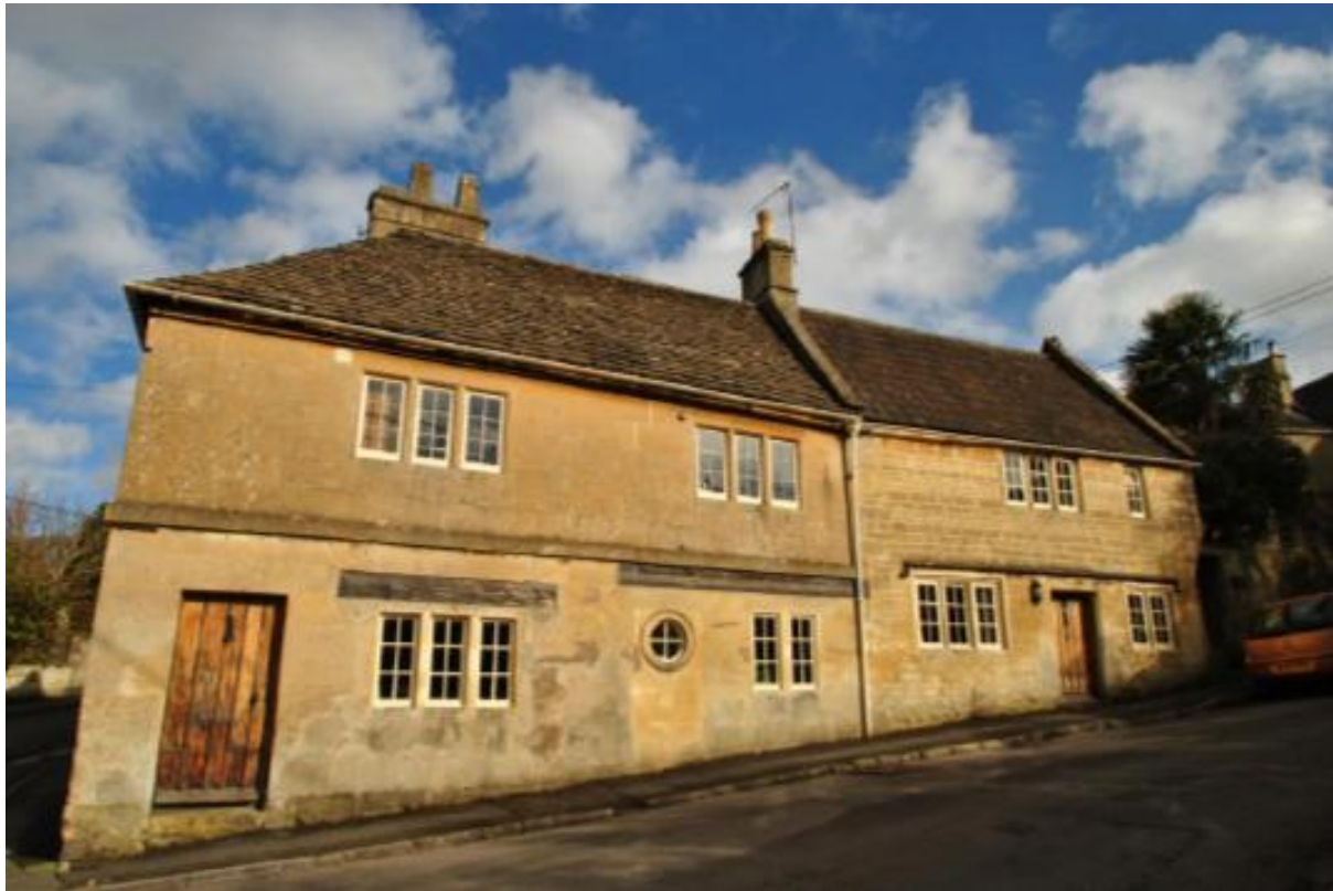
Photograph 1: showing a view of the building
