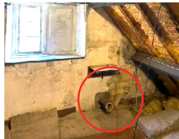
Soil pipe in north gable
