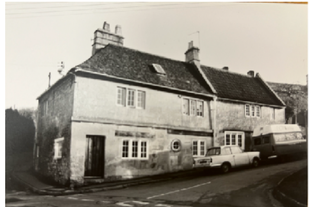
Rooflight on the southerly roofline prior (removed 1987)
