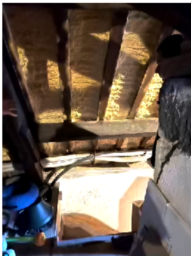
Access to attic
