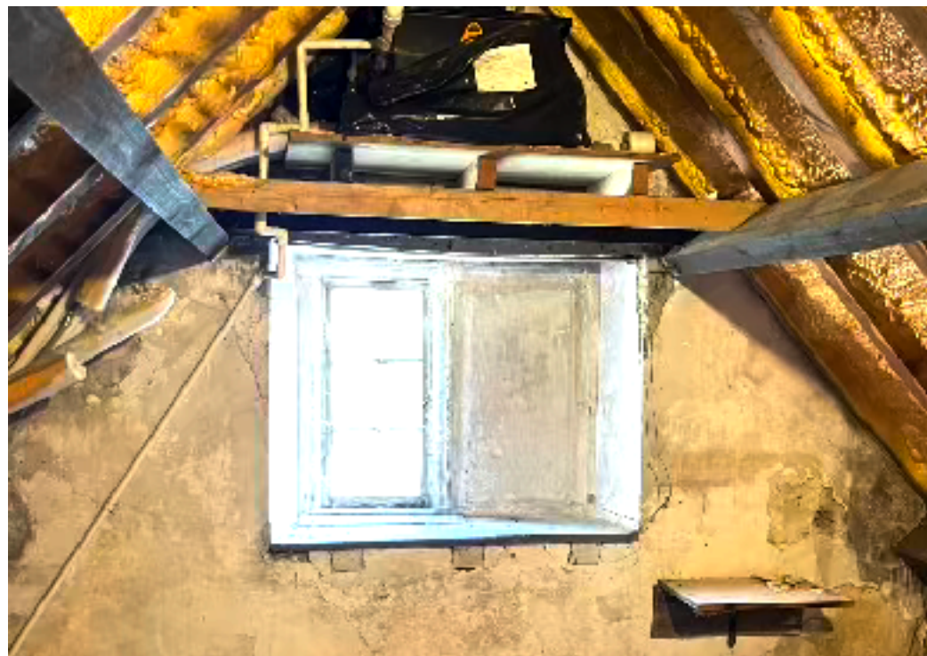
2 light window in attic on north gable
