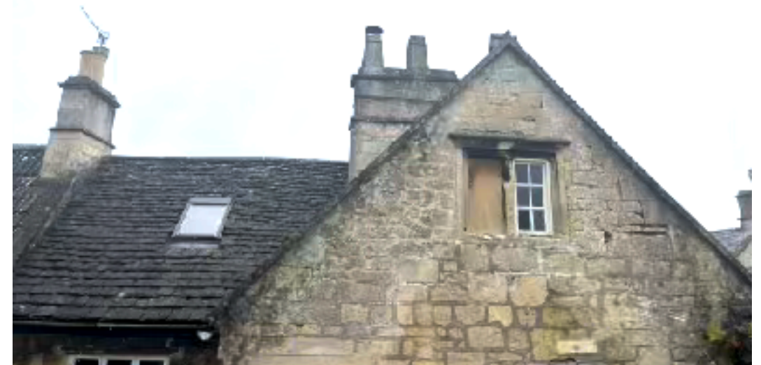
Former attic window, now partially blocked
