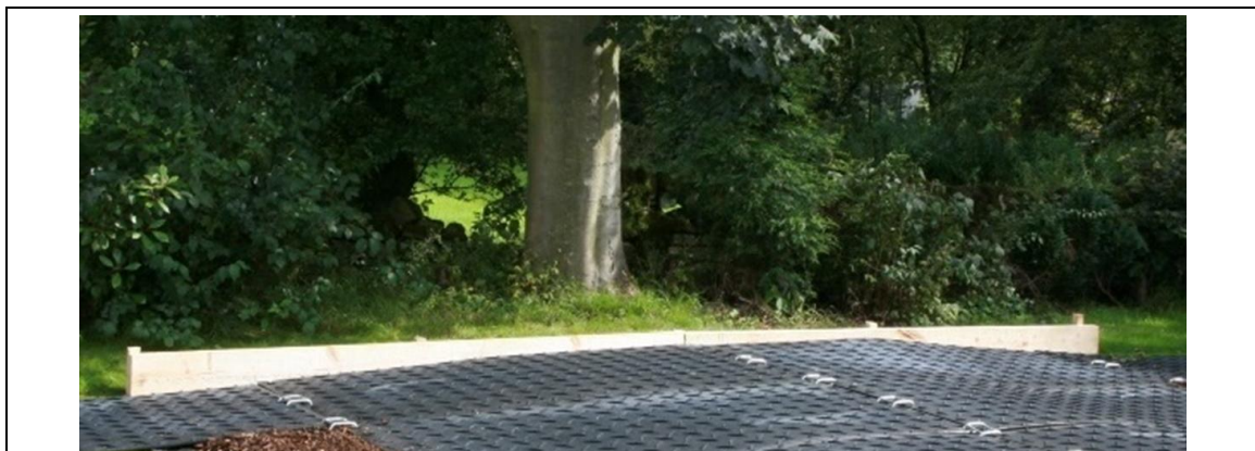
Figure 1: Example of proprietary, inter-linked ground protection boards used to protect RPAs.
