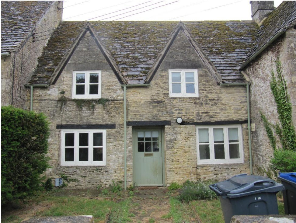
Main front façade of 7 Park Street Charlton
