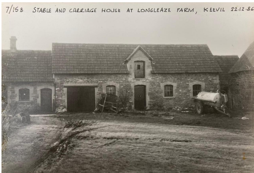
Figure 8 – This is the earliest picture of the stables held at the Wiltshire and Swindon History Centre. It was taken in 1986, prior to residential conversion. The windows had been recently installed by the previous owner, and replaced chicken wire
