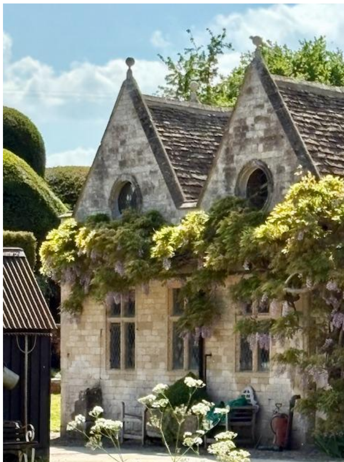
Figure 12 - Grade 2 Listed - the coach house and stables at Blagden House
