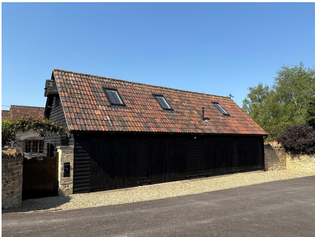
Figure 10 - Existing rooflights in garage
