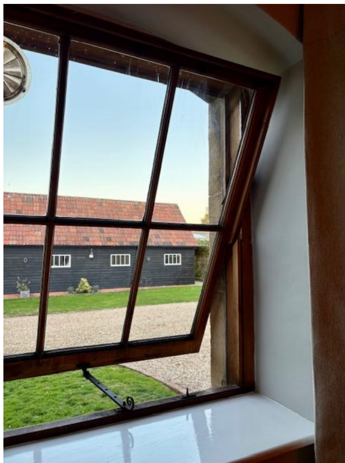
Figure 20 - Internal view of typical existing window
