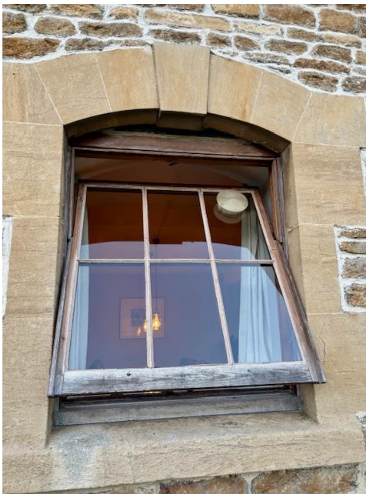
Figure 11 – Existing window, external view
