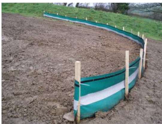
Fig 1. Example of silt barrier installation
