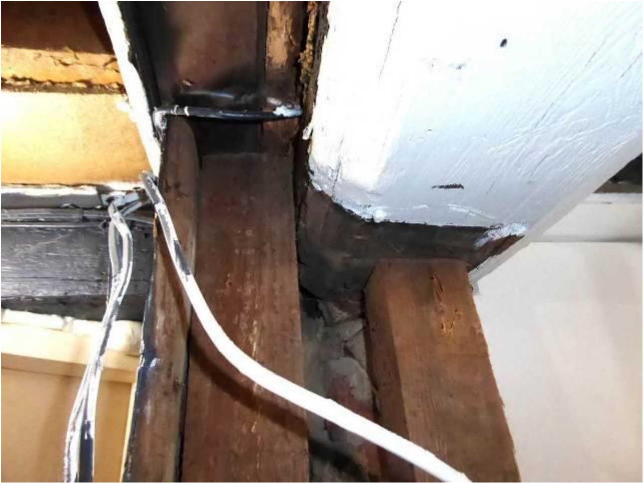
Modern end support post butted against brick pier
