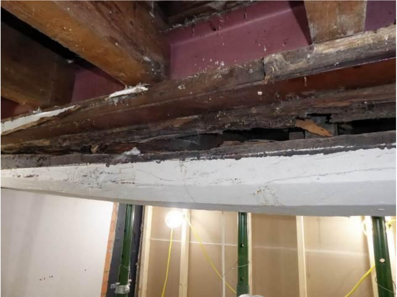
Beam over bar area
