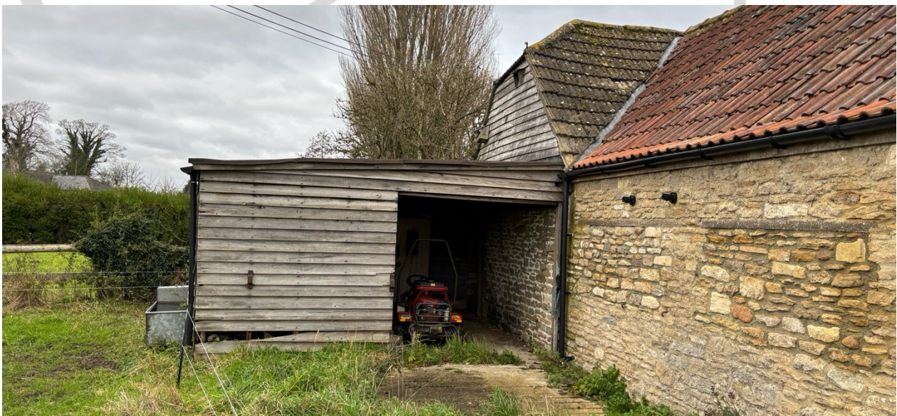
Image: South West and South East Elevation. Timber lean-to element.
