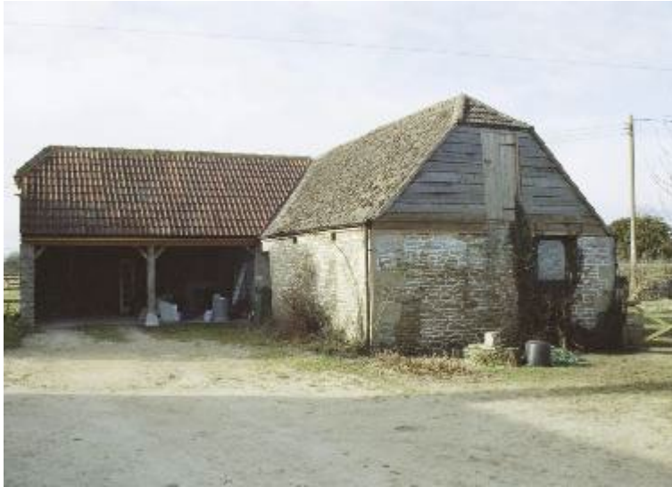
Plate 9: Photograph of the Grade II Listed Stables at Coggsell, 2006 (Historic England).
