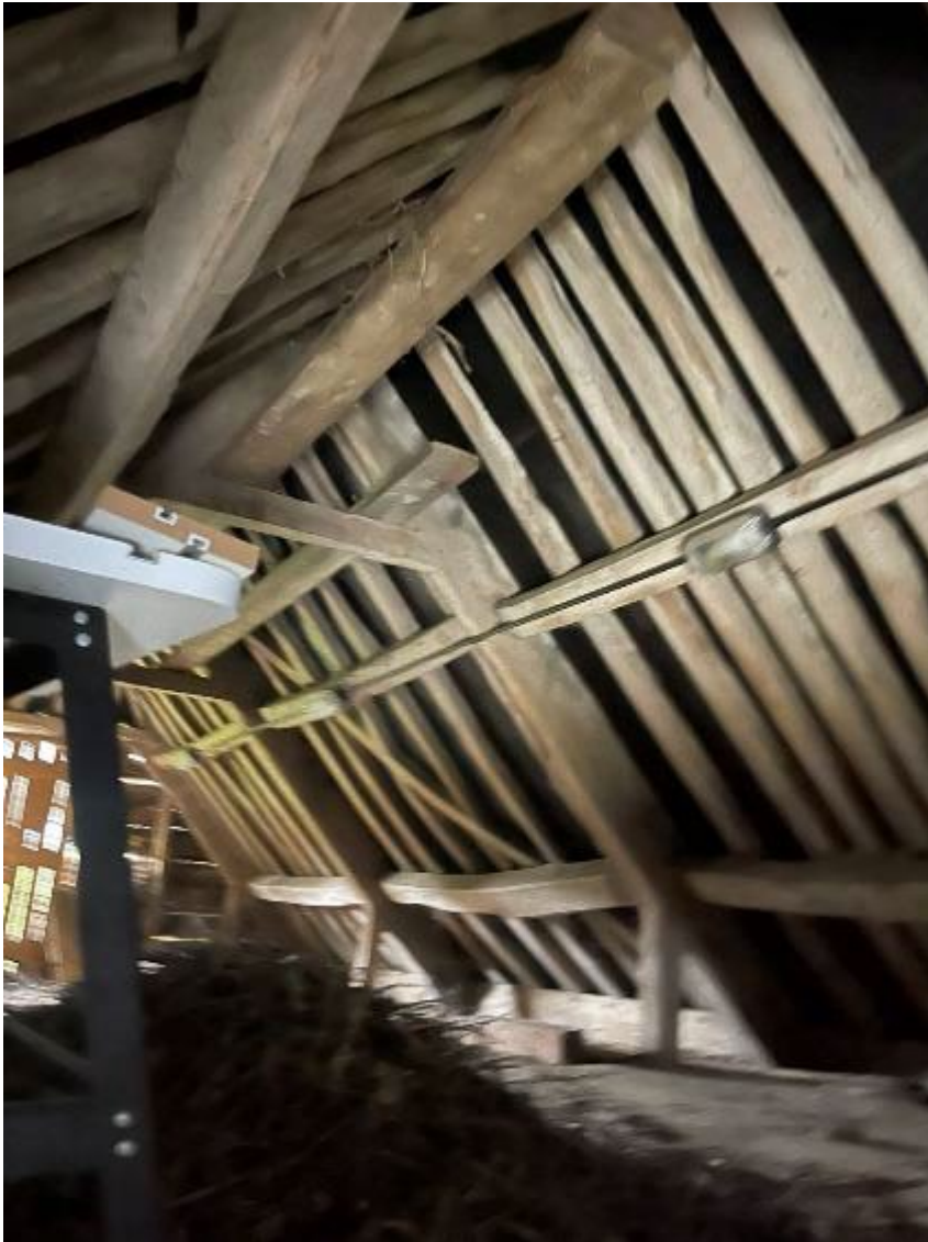
Plate 25: The historic roof structure of the loft space, including hand sawn timber beams.
