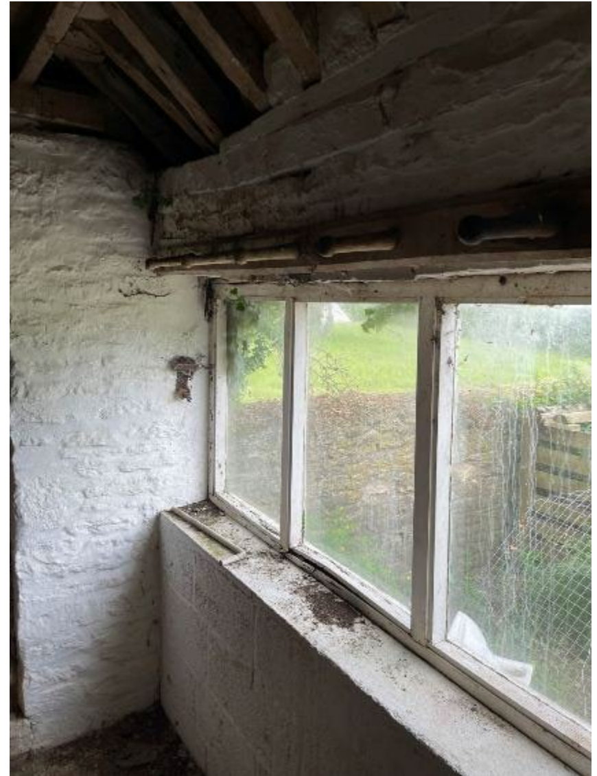
Plate 18: The inserted window with timber pegs above, and concrete block wall below, within the south-western compartment.
