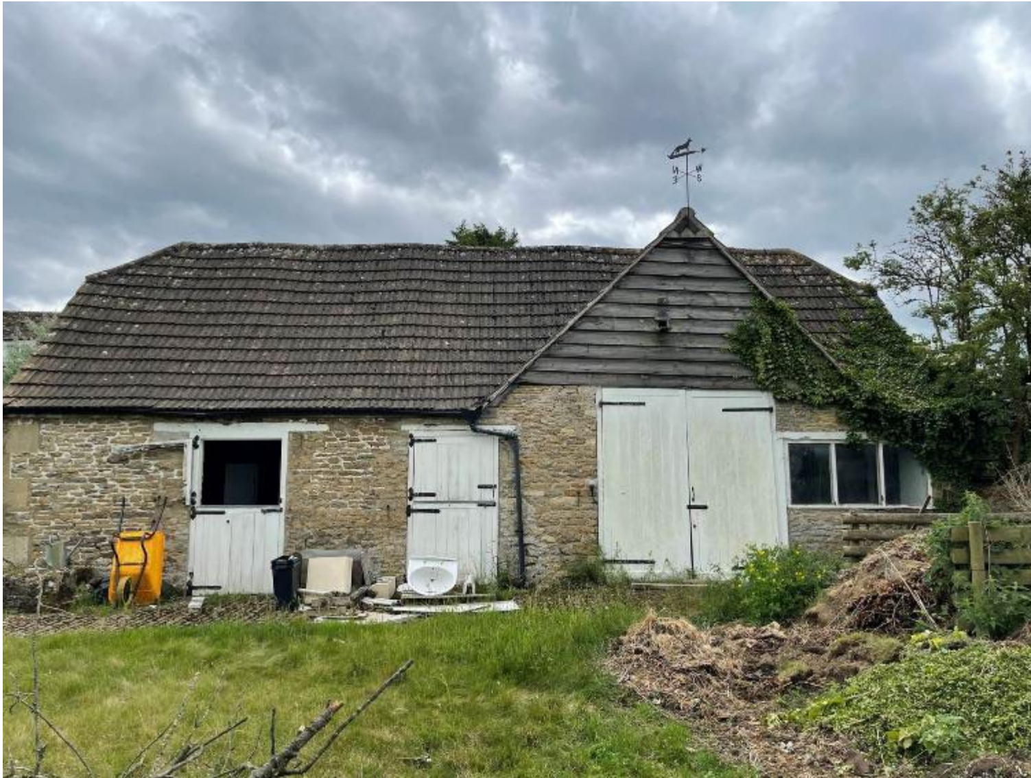
Plate 13: The principal north-western elevation of the Grade II Listed Stables at Coggsell.
