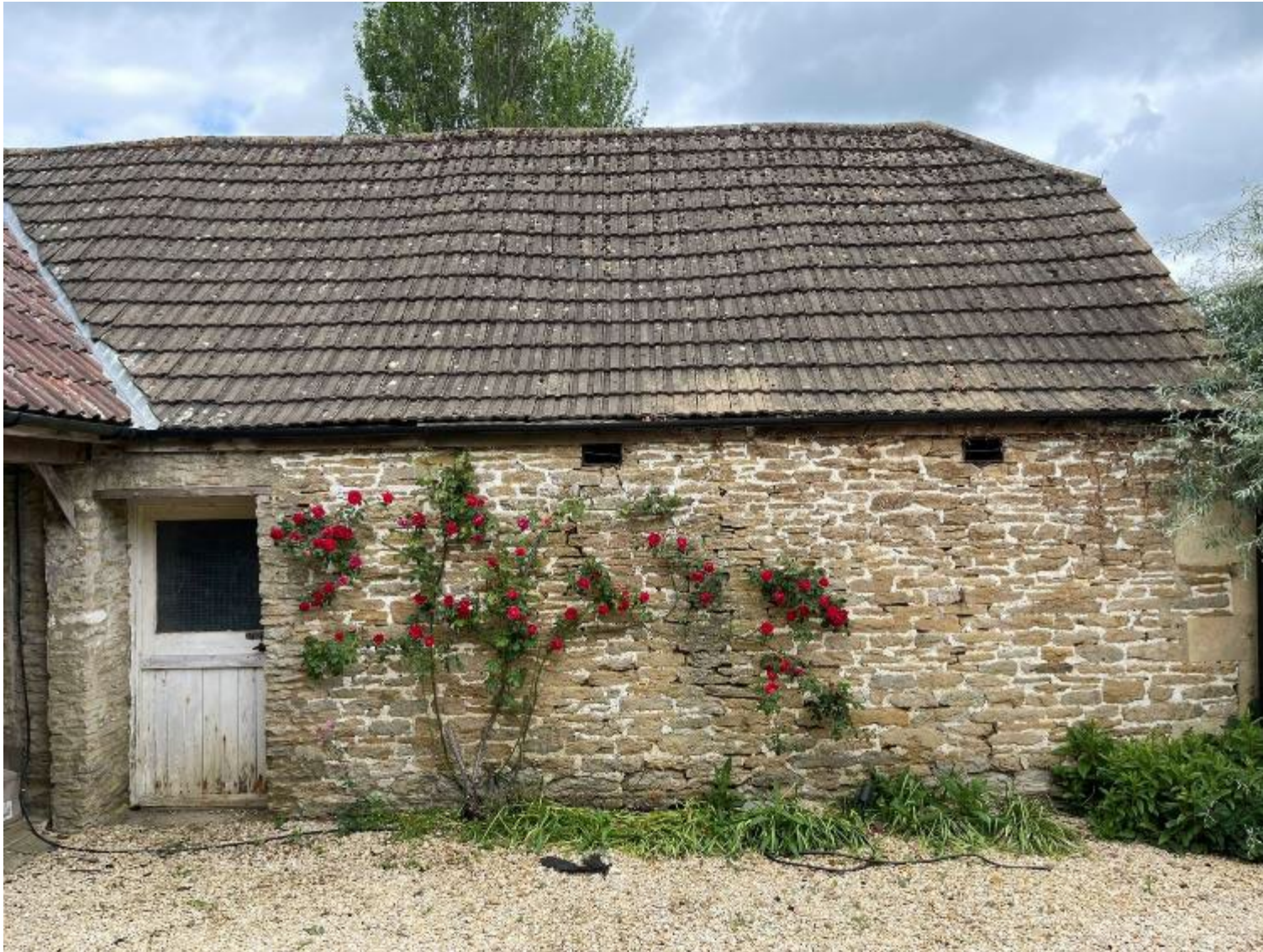
Plate 16: The south-eastern elevation of the Stables at Coggsell.
