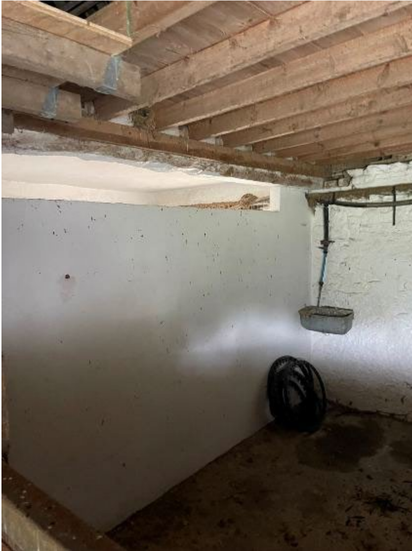
Plate 19: The modern partition wall and modern machine cut timber ceiling structure of the south-western compartment.
