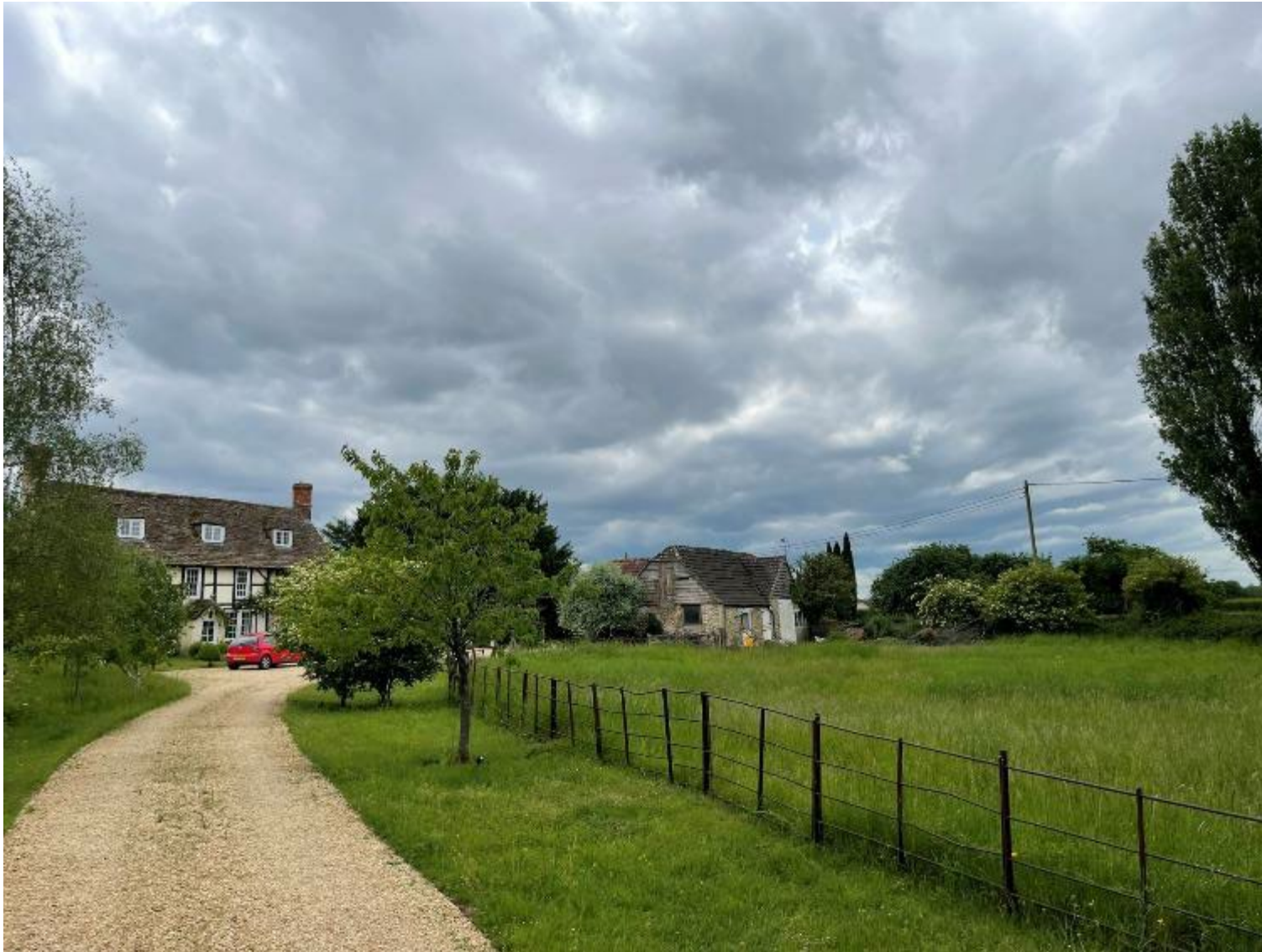
Plate 27: View along the gravel access track, towards the Grade II Listed Stables at Coggsell, and the associated Grade II Listed Coggsell.
