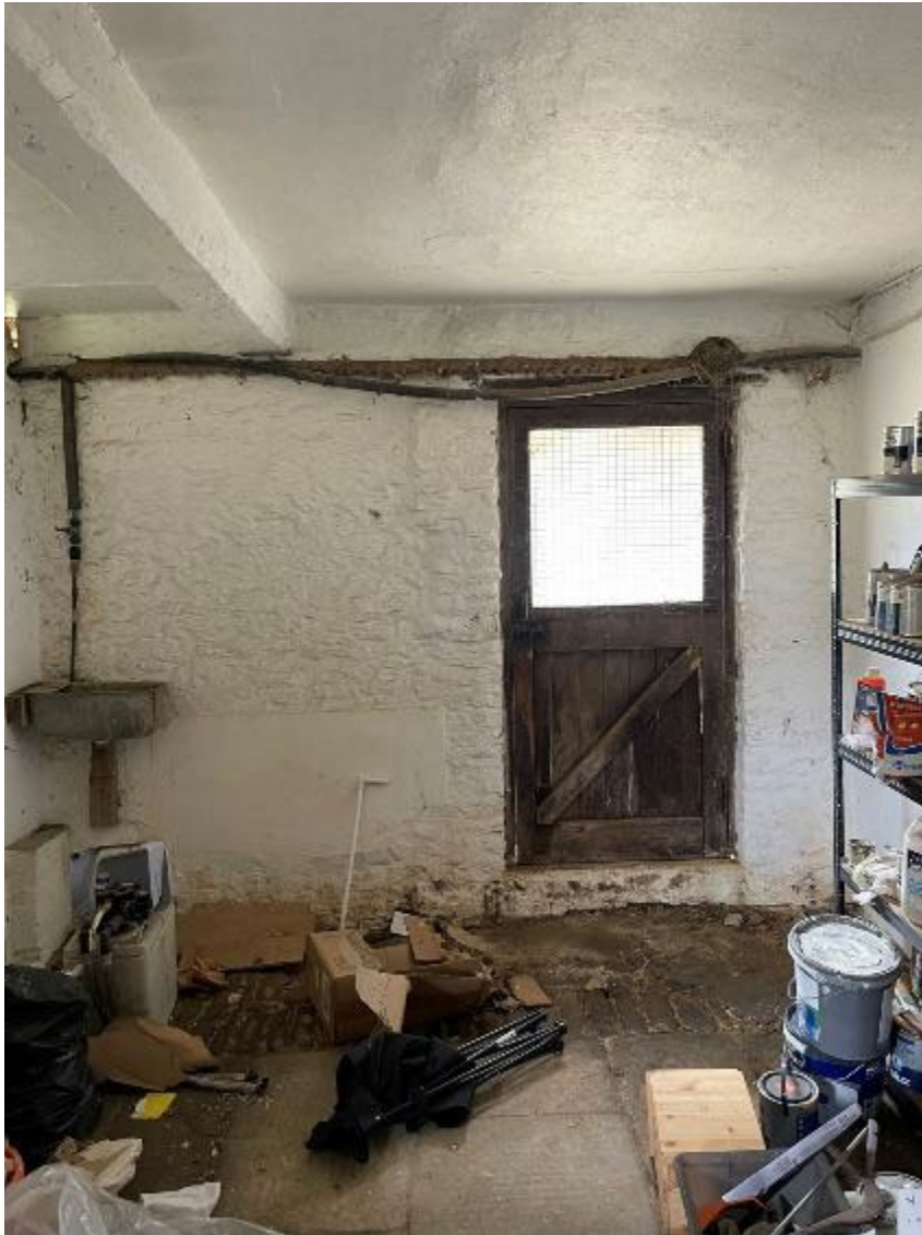
Plate 21: View south-eastwards within the central compartment, showing the flagstone floor, section of cobbled stones, and exposed timber beam.
