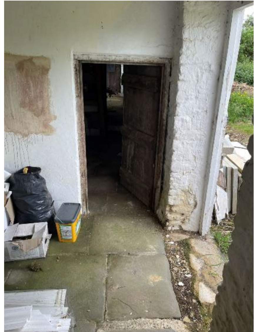
Plate 24: View south-westwards within the north-easter compartment, showing the historic flagstone floor, as well as the ledged timber plank door, set within a modern partition wall.
