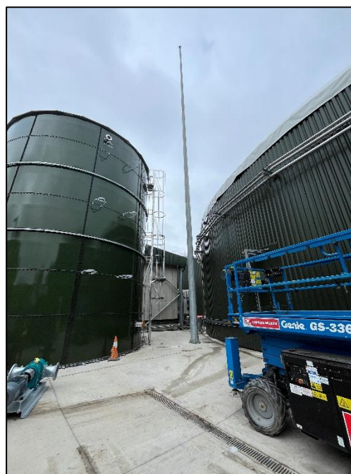
Figure 16: Telescopic Mast
