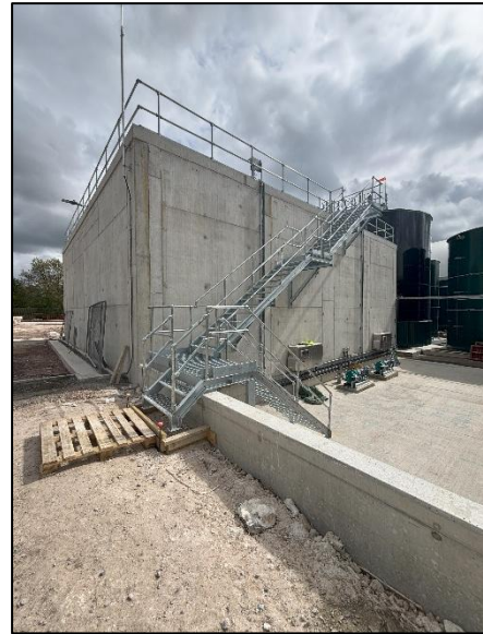
Figure 20: HVI Conductor to Building
