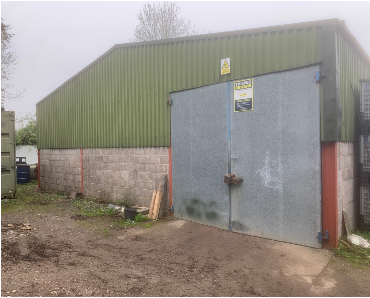
Photo of the south elevation of the barn
