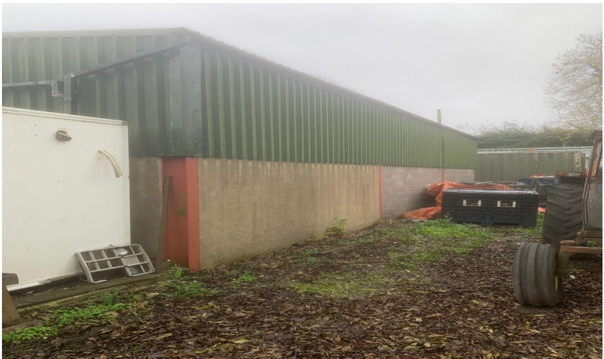
Photo of West elevation of the barn
