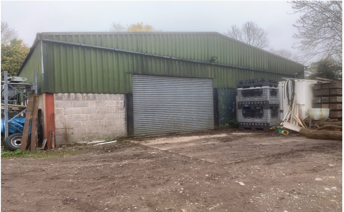
Photo of north elevation of the barn
