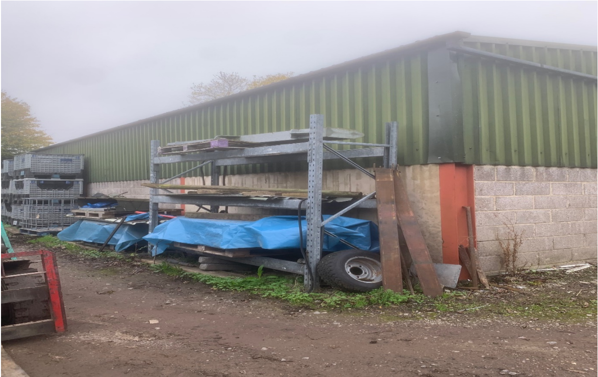
Photo of East elevation of the barn
