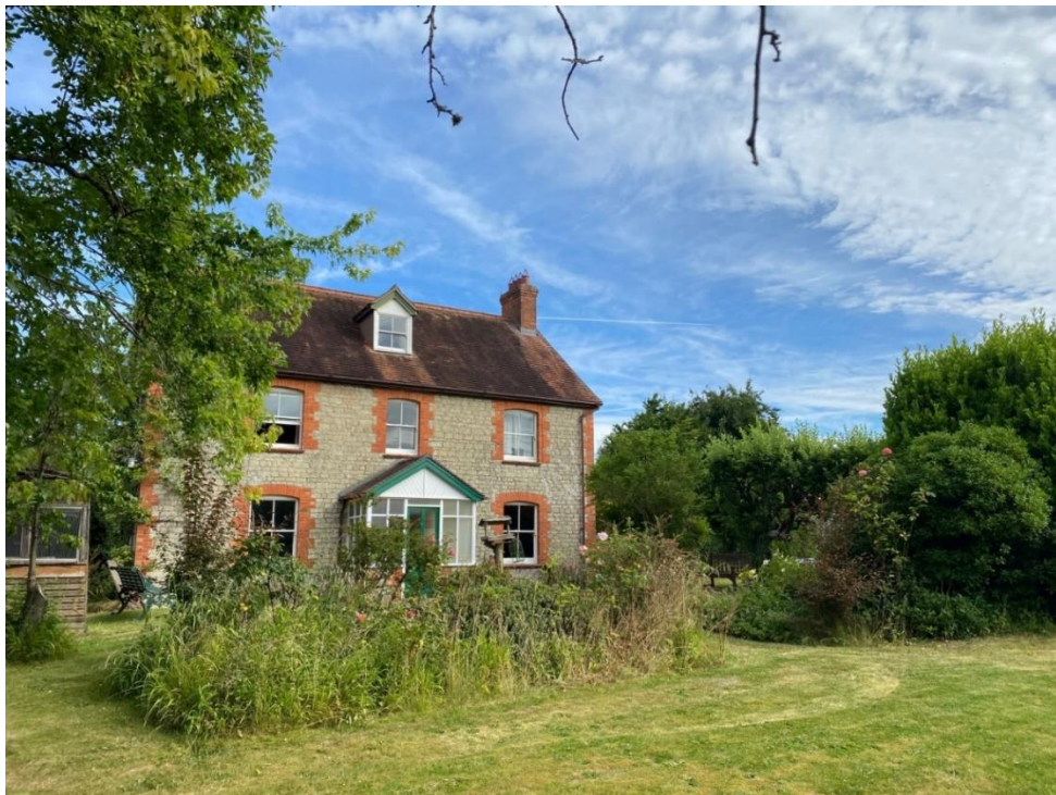
Figure 2: Southern elevation of Elmsleigh
