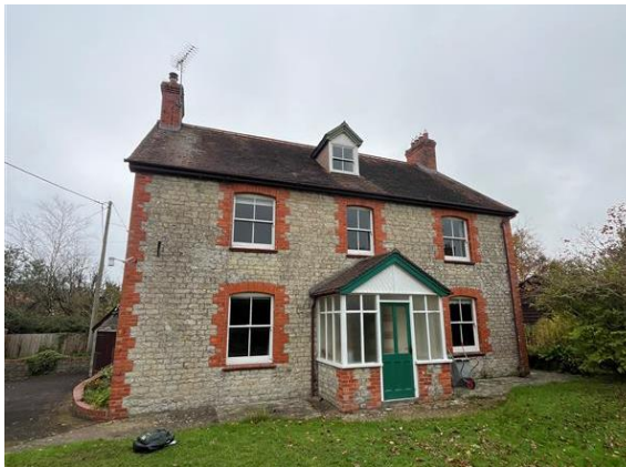
Photo 1: Elmsleigh main house.
