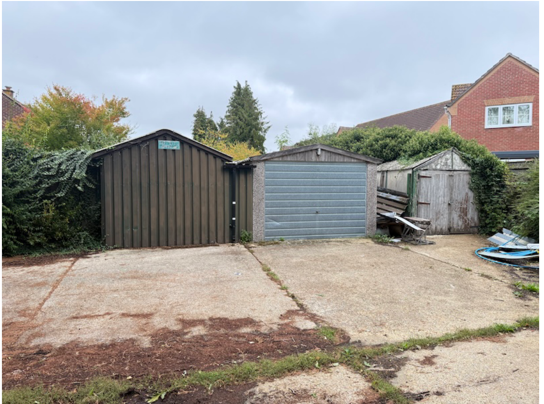
Figure 7 – View of Garages from Shared Road
