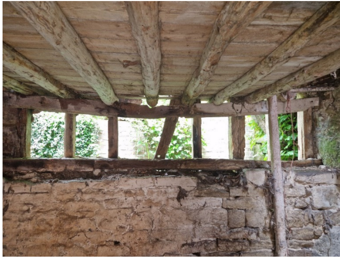
Existing floor joists supported on oak frame
