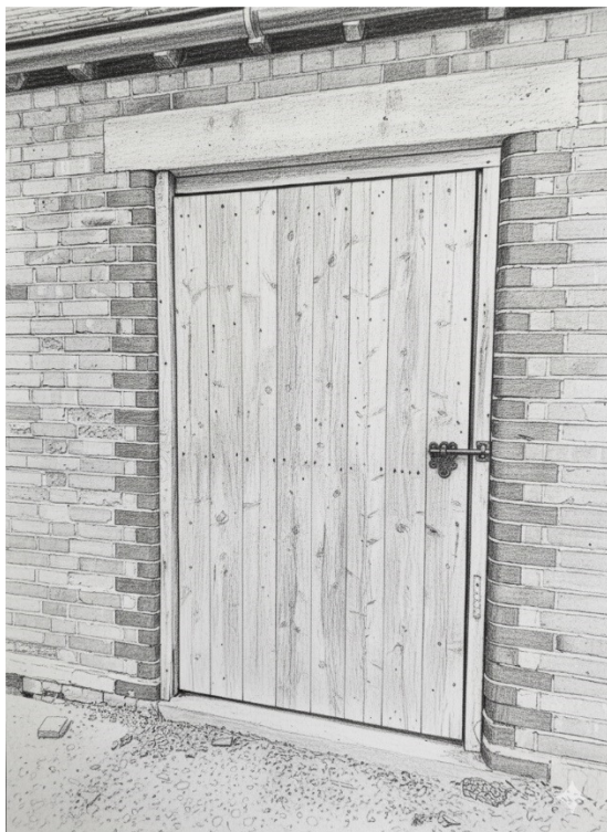
Simple plank doors to outbuilding
