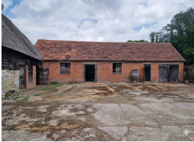
Existing yard and Outbuildings
