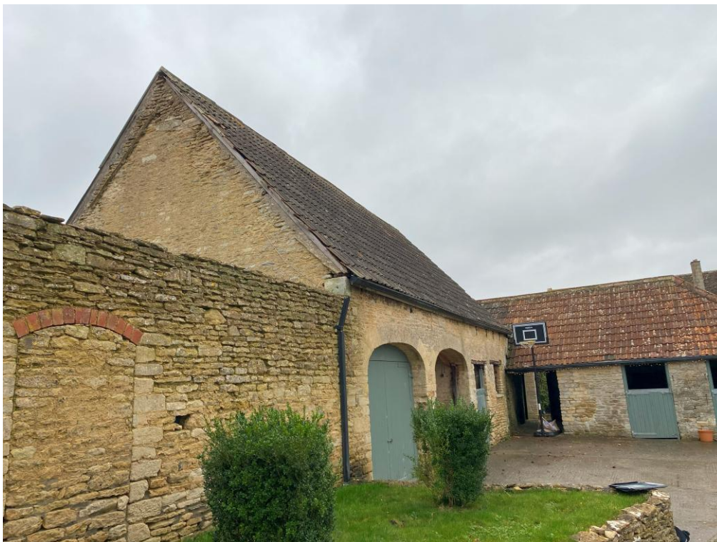
Photograph 17. B5 and B6 – southern and eastern elevations, respectively
