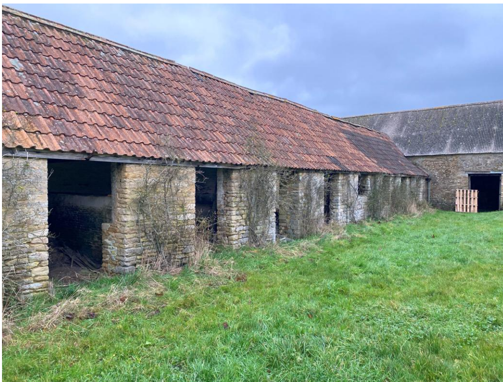
Photograph 22. B10 – southern elevation
