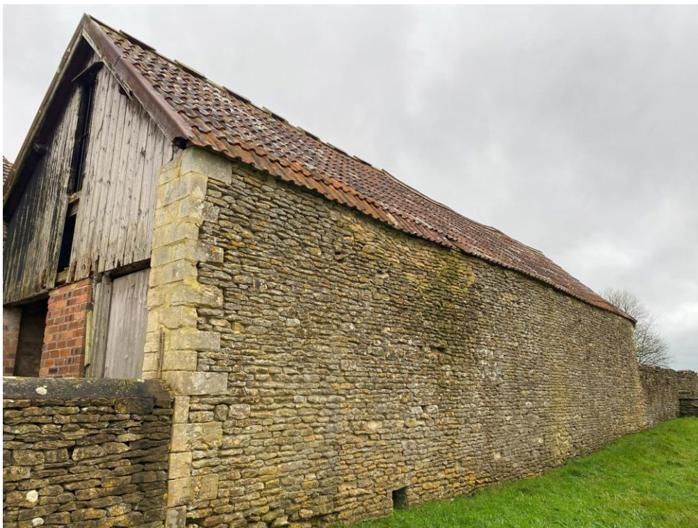
Photograph 5. B2 – northern elevation
