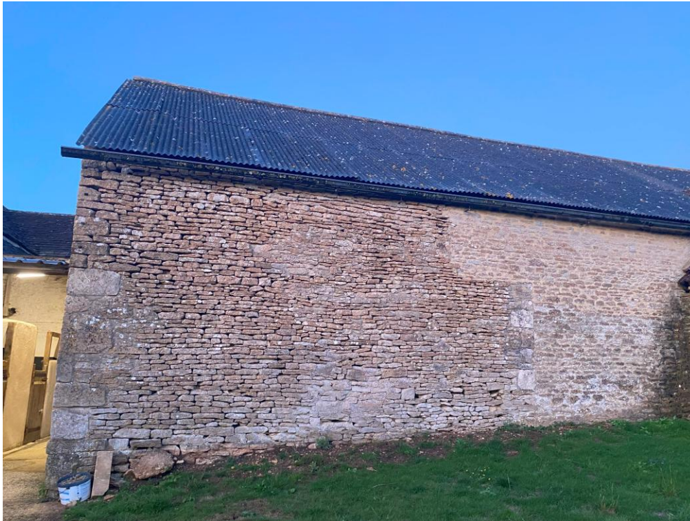
Photograph 20. B7 – western elevation
