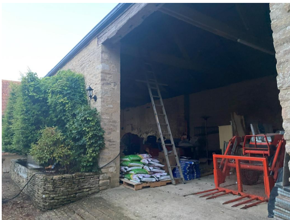
Photograph 19. B7 – eastern elevation/interior
