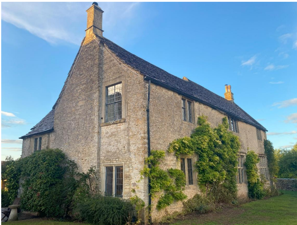
Photograph 23. B10 – southern and western elevations
