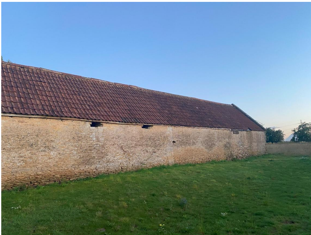
Photograph 21. B10 – northern elevation
