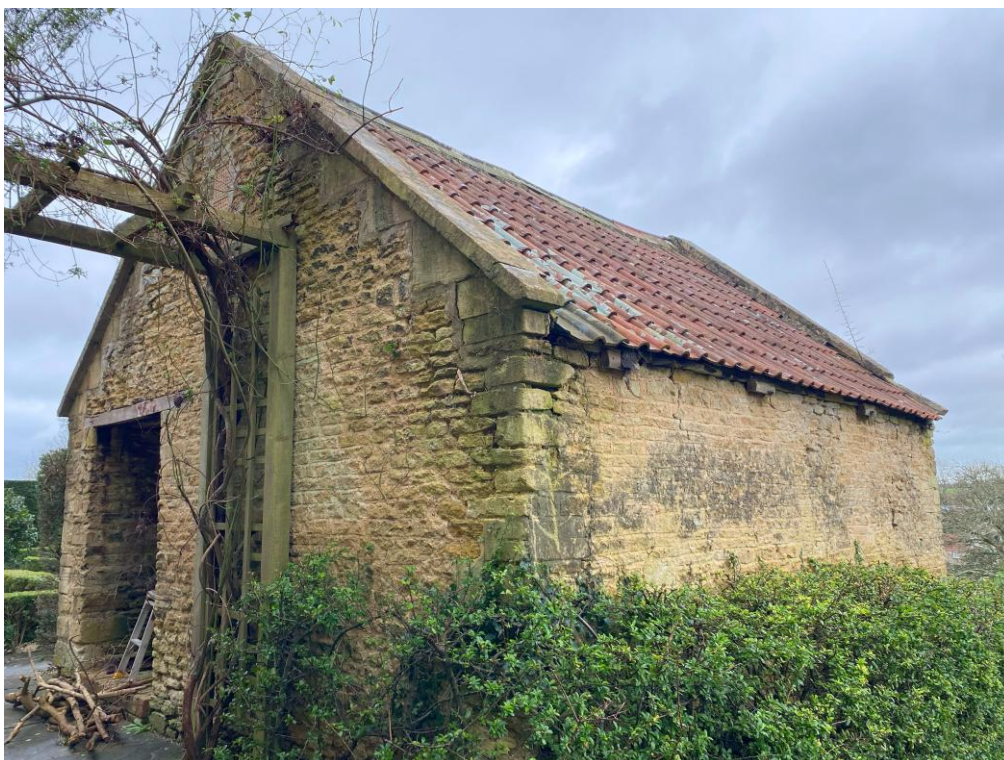
Photograph 4. B1 – eastern and southern elevations
