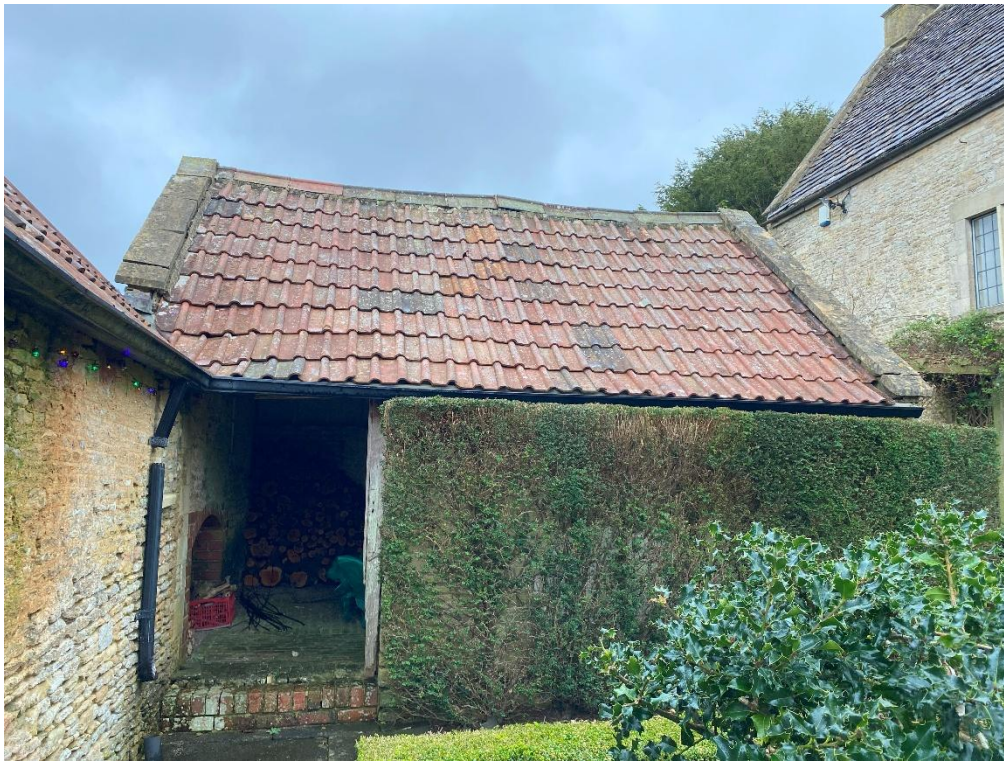
Photograph 3. B1 – western elevation
