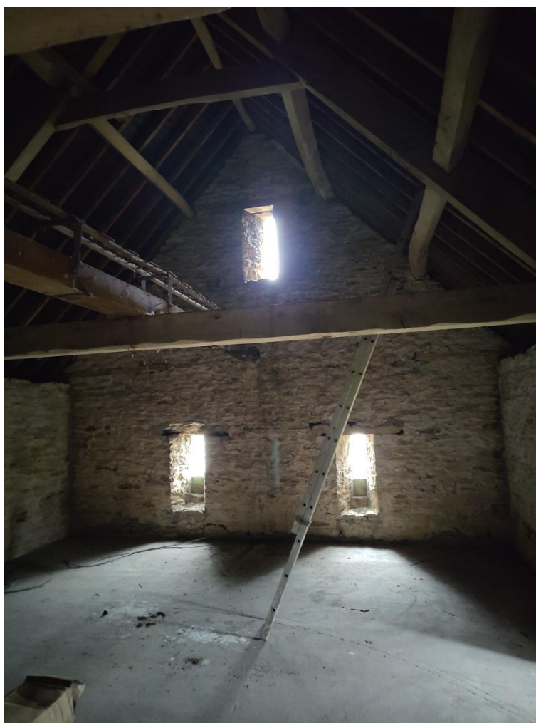
Photograph 15. B4 – upper interior
