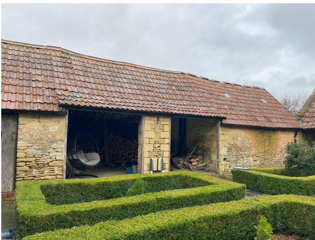
Photograph 7. B2 – southern elevation
