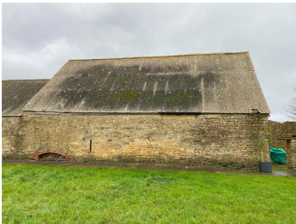
Photograph 18. B6 – western elevation
