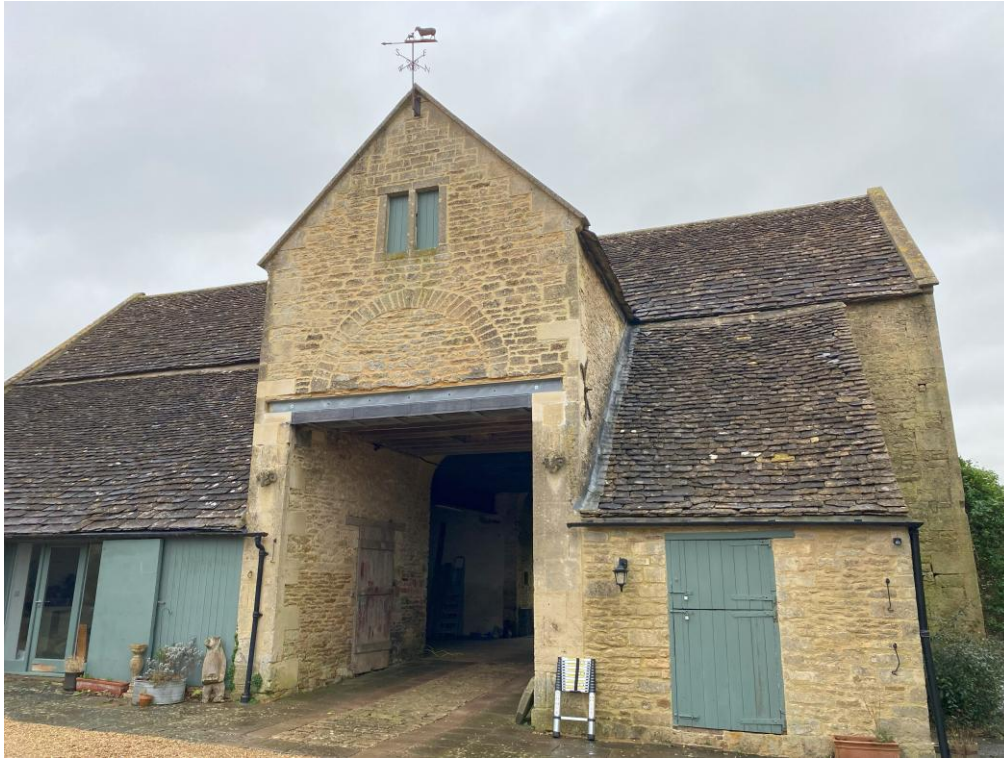
Photograph 12. B4 – southern elevation
