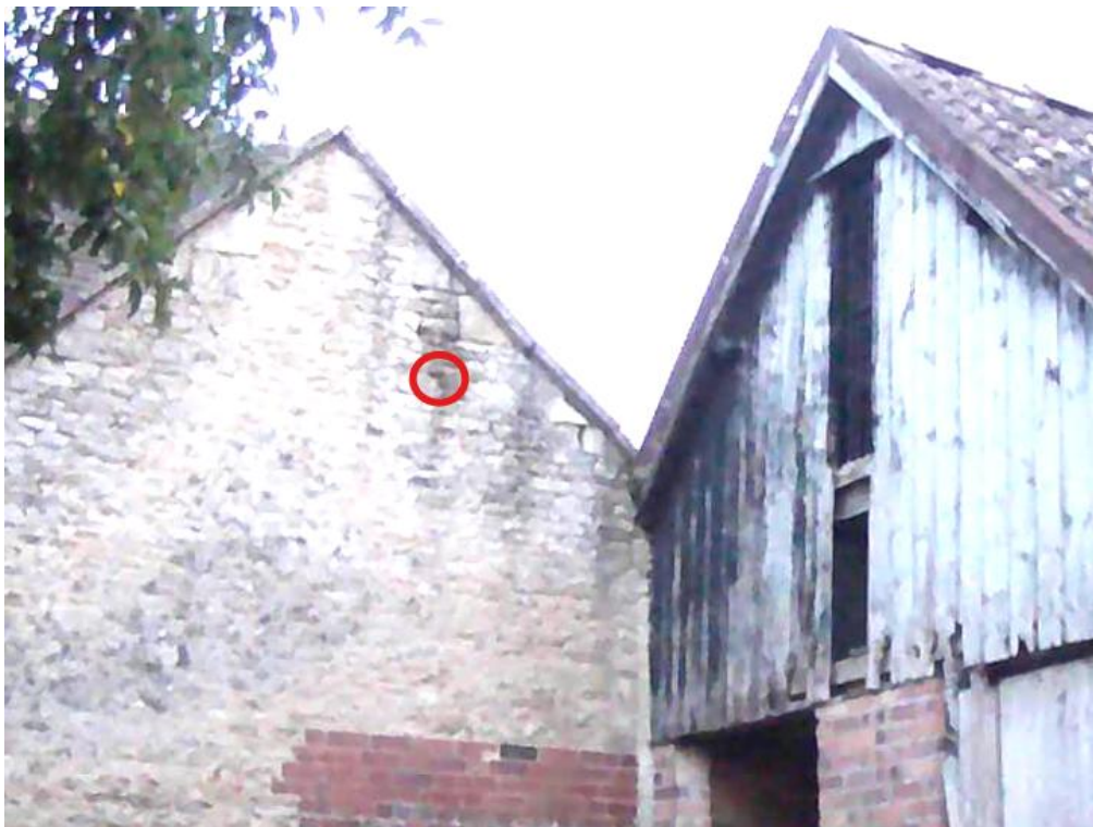
Figure 4: R1 – Soprano pipistrelle roost access point
