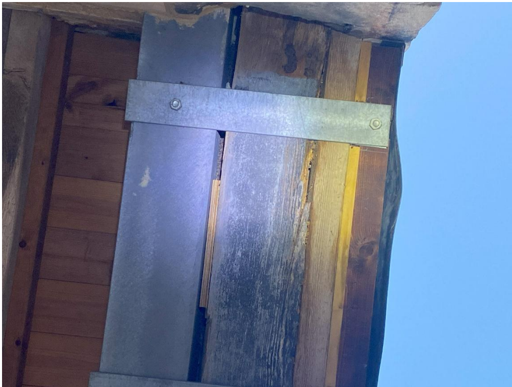
Photograph 3. Lintel above doorway in B4
