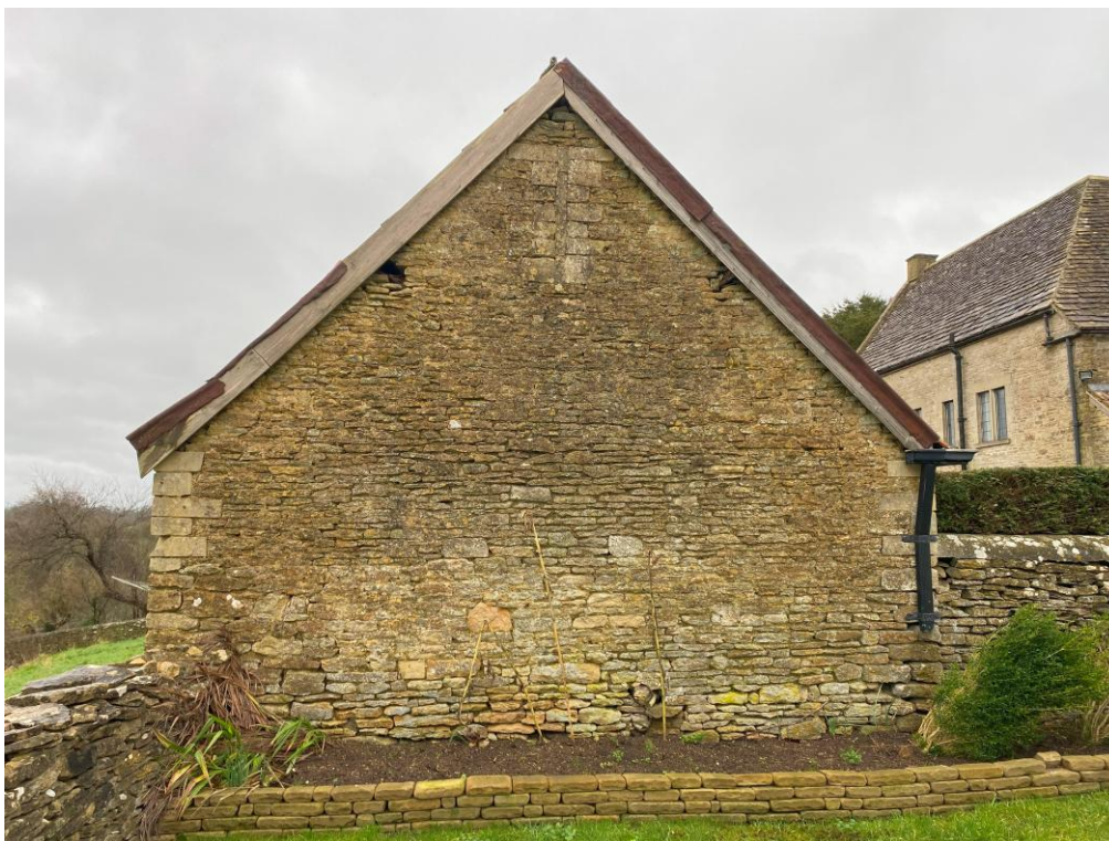
Photograph 8. B2 – western elevation
