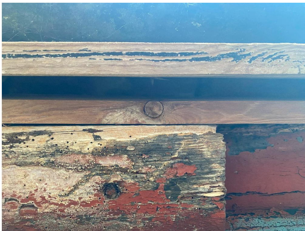
Photograph 4. Lintel above doorway in B5
