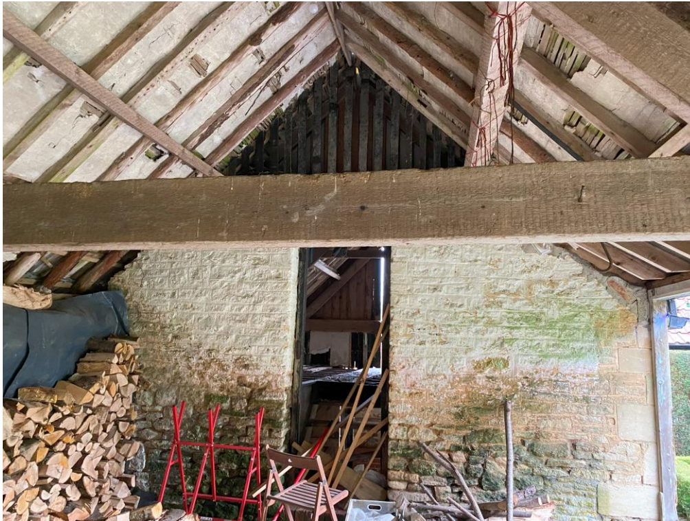
Photograph 10. B2b – interior facing east
