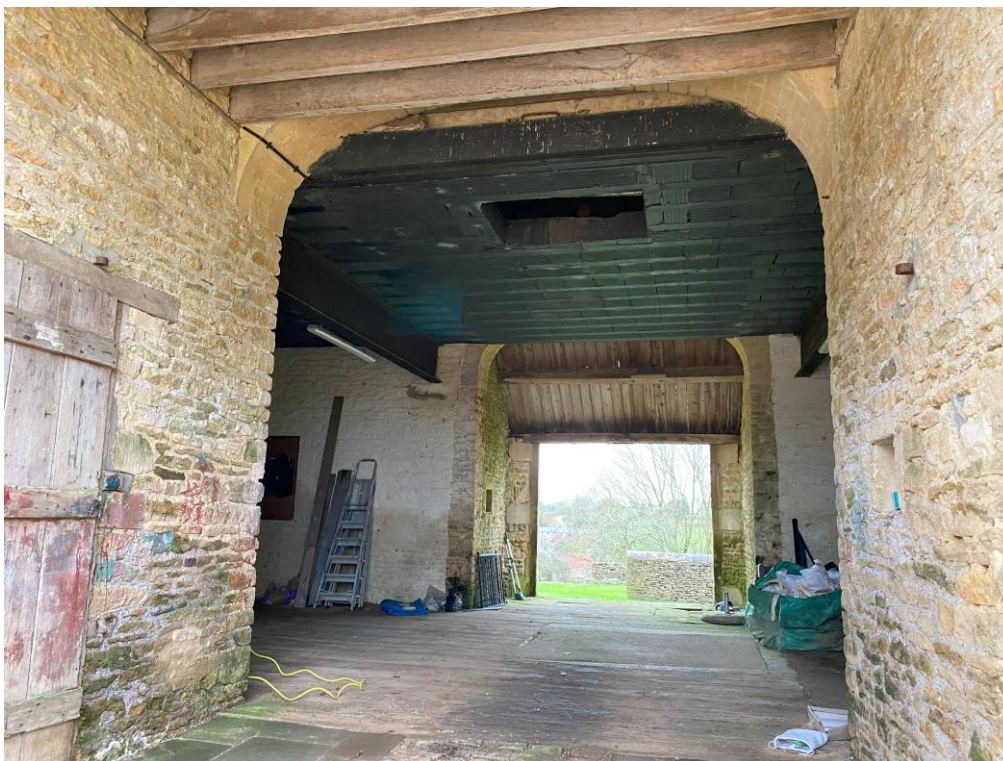
Photograph 14. B4 – lower interior
