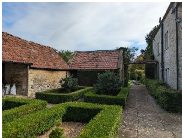
8. View towards 1920 outbuilding and link location
