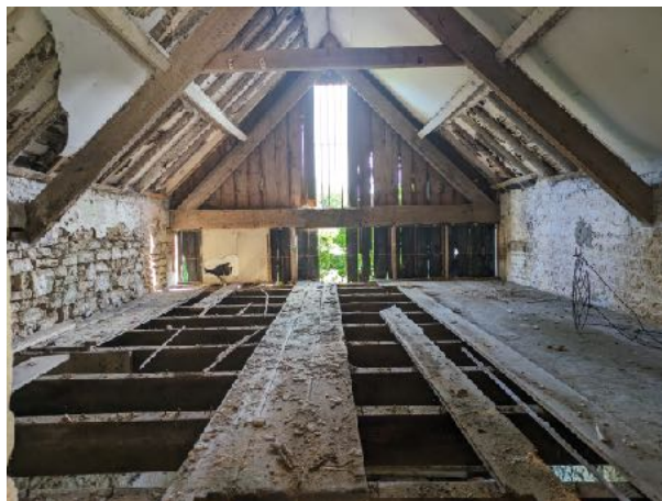
11. Mezzanine level of north end of outbuilding
