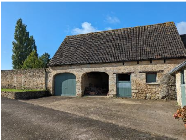
27. Office barn and attached cart shed
