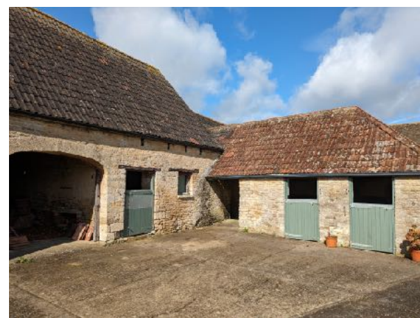
29. The stable building, southern elevation
