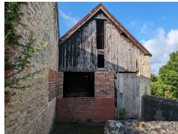
9. Timber gable at north end and pigsty
