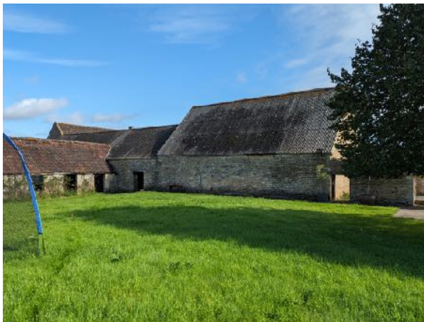
28. Rear of Office barn
