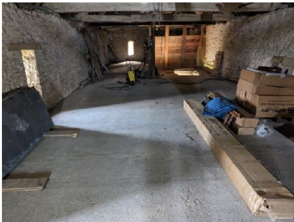
19 Main Barn; concrete first floor looking east
