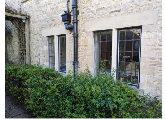
3. The north utility windows c.C20 insertions in location of link
