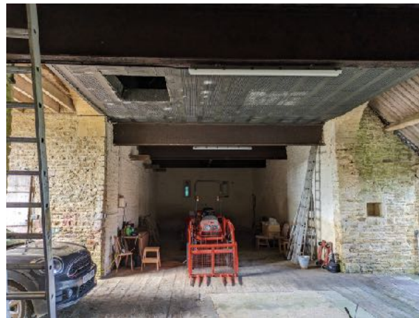
20. The Main Barn; threshing floor under concrete first floor
