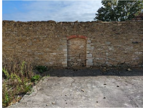
34. Blocked door in east elevation of cart shed
