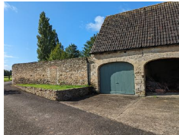
32. The eastern elevation of cart shed
