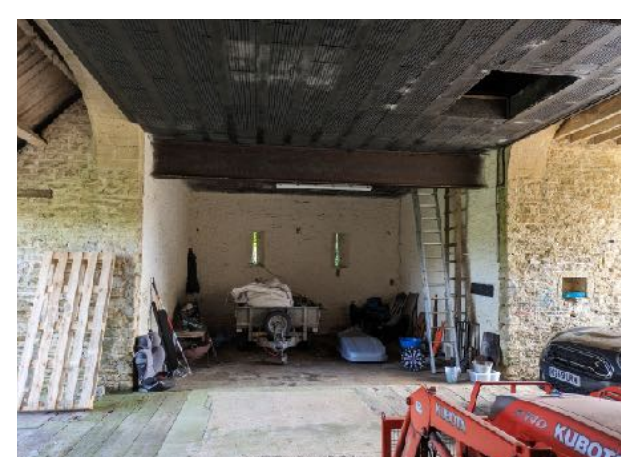
21. Looking east in Main Barn
