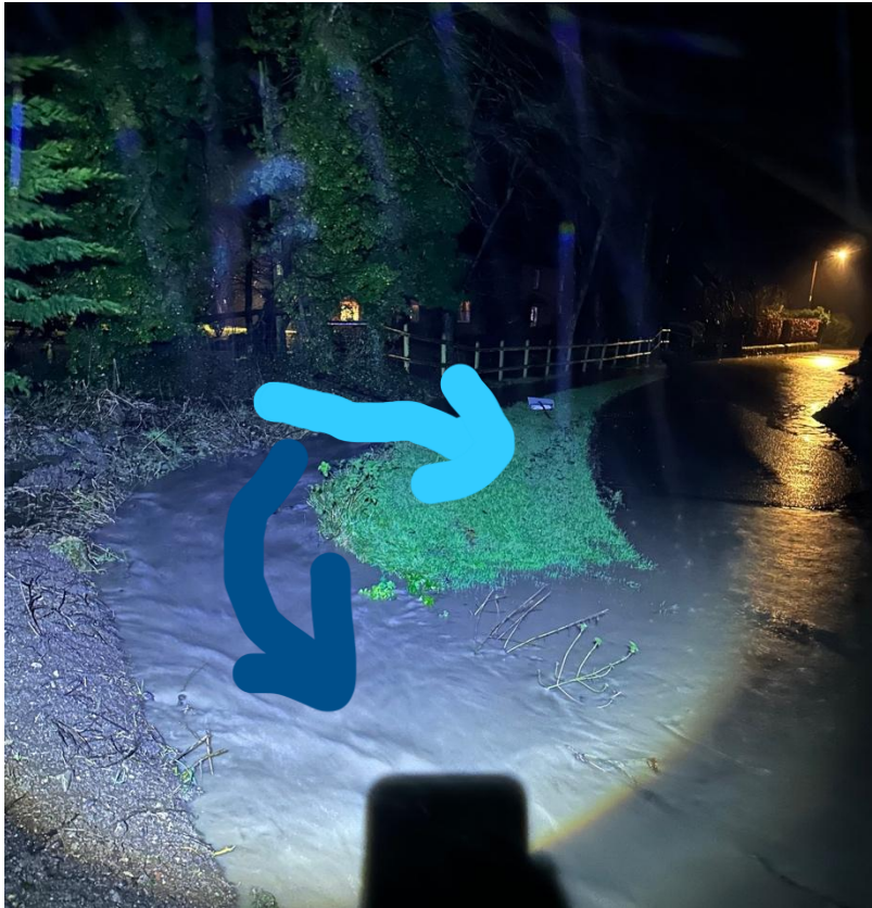
Water exiting the Gog via the drainage channel due to being unable to pass under the culvert. 4 th January 2024.
