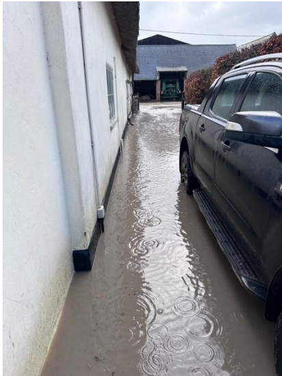
28 th March. Water flowing off the lane in Allington and into the driveway along our house prior to re entering the Gog below the culvert.
