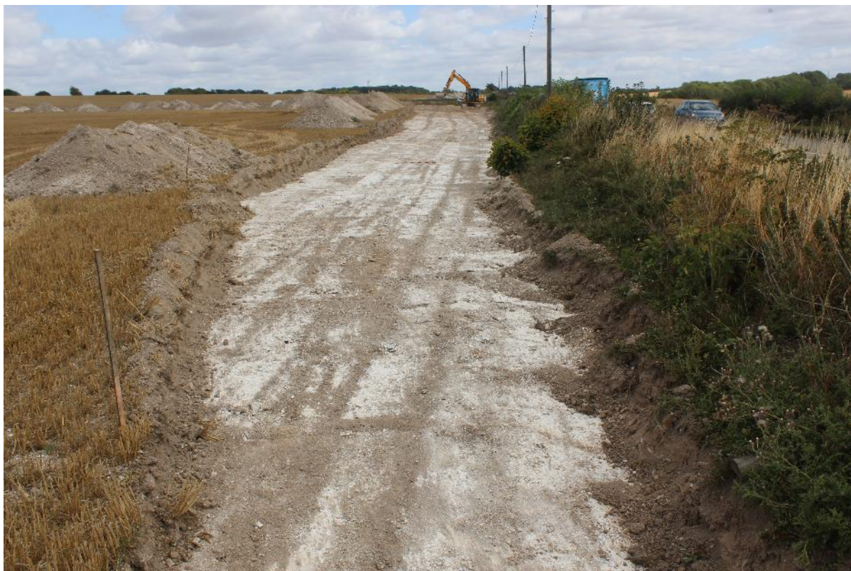
Plate 1 – Overview of Southwest stripped area, taken looking northeast with a 1m scale.
