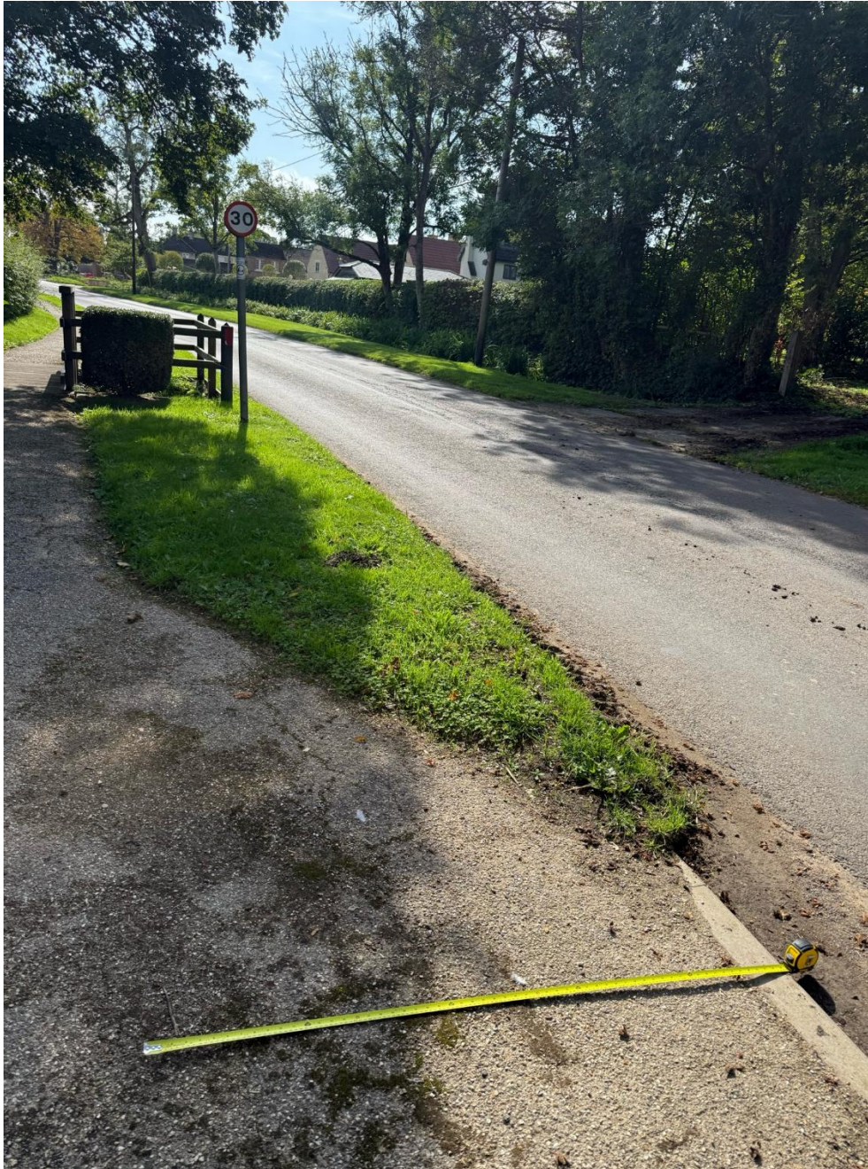
Figure 2.2: Culvert post and rail fence - view taken 1.5m back at location of proposed crossing point
