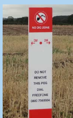
When the pipeline route has been located it will be marked with location pegs.
