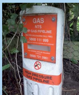
National Gas marker post
