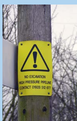
Pole warning marker
