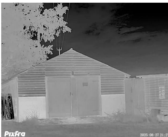
Figure 2: Still from infra-red camera facing the northern elevation.
