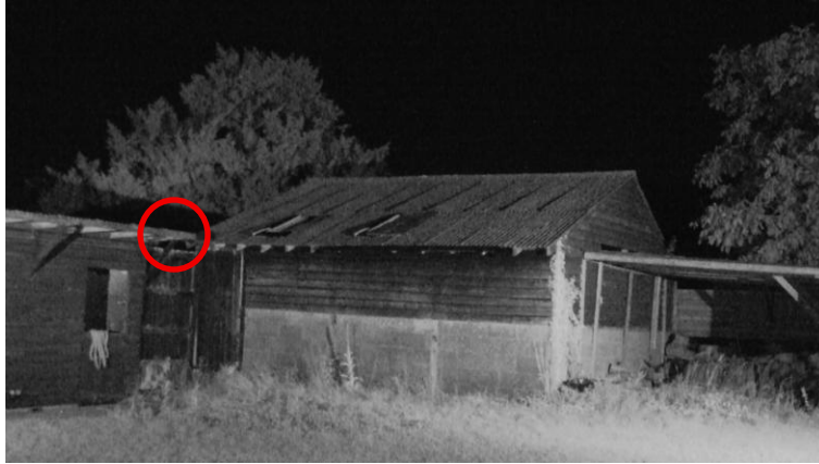
Figure 3: Common pipistrelle roost location in Barn B.
