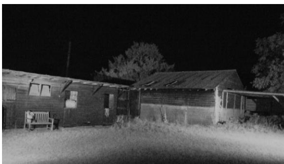
Figure 1: Still from infra-red camera facing the southern and eastern elevations.
