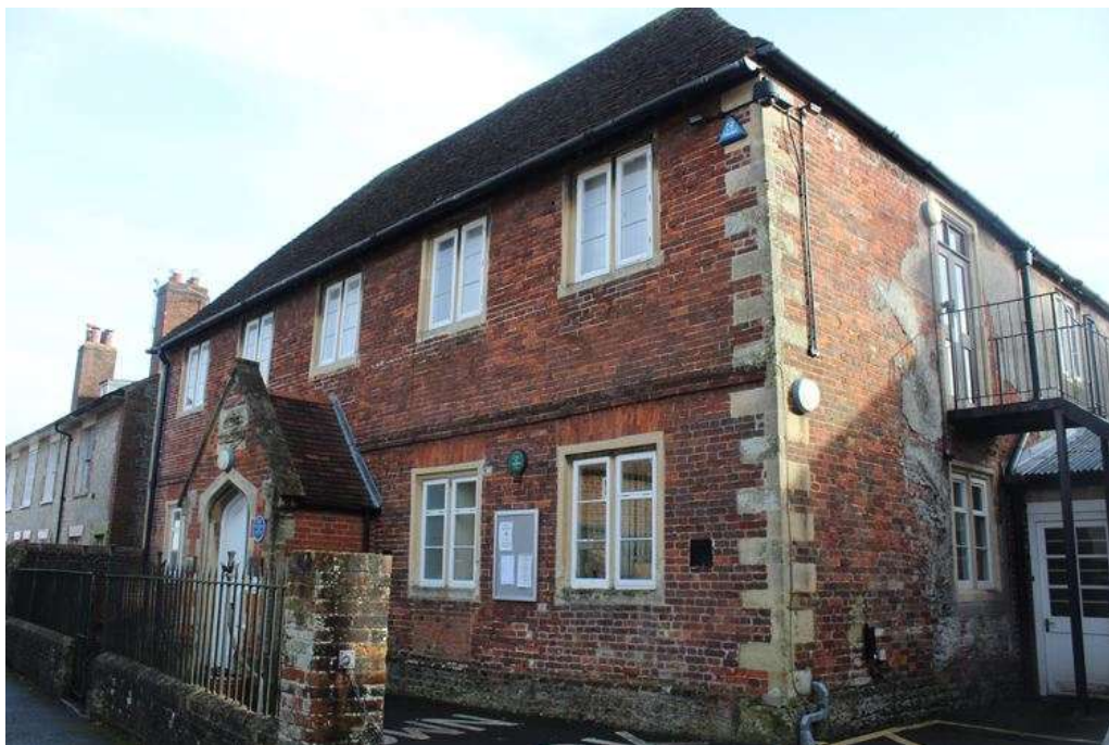
Fig 1 – Front elevation of building to North Row
