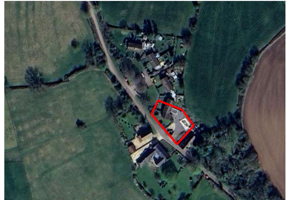
Figure 3 Site view (Google Maps)
