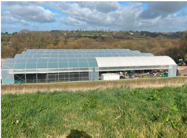
Photograph 8 – View the top of the field bank looking down at the planning approved poly tunnel
