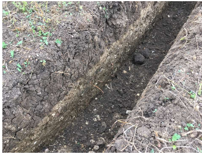
Photograph 5 – Trial trench to identify if there is any builders waste to a depth of around 1m.
