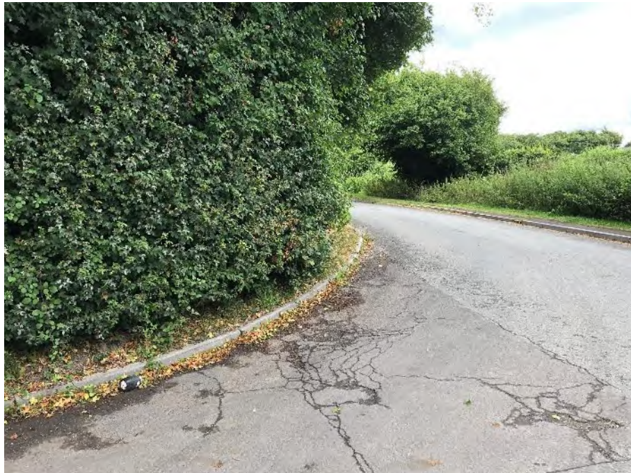
Photograph 3.1: Visibility looking left from existing site access
