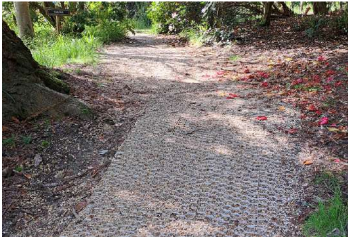
Gravel-filled cellular confinement system at Leonardslee
