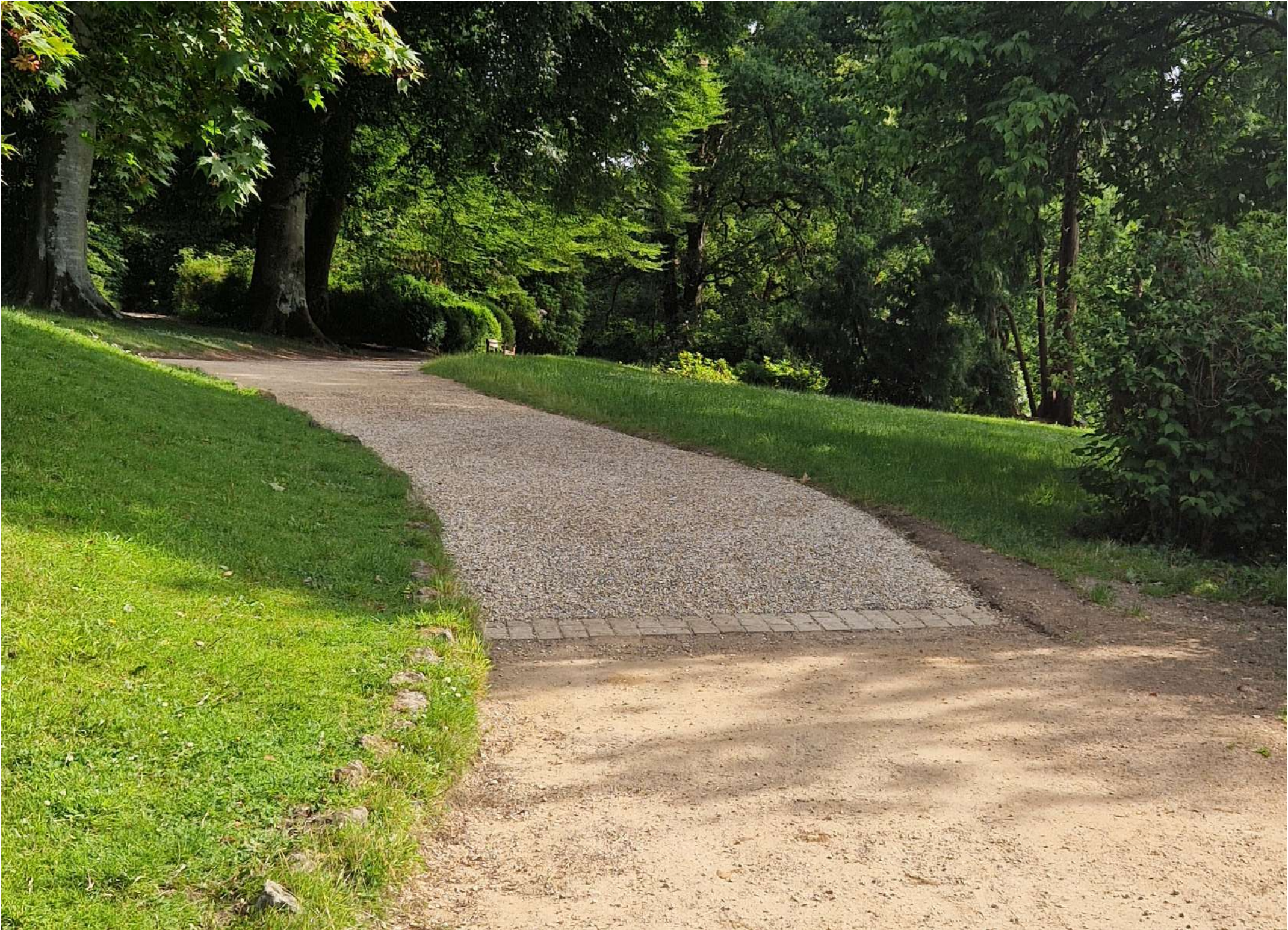
Figure 54. Site Photo - first sample section of path adjacent to the Gothic Cottage, June 2025
