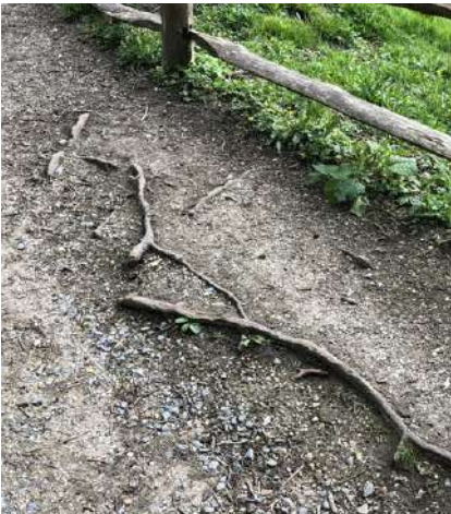
Exposed tree roots
