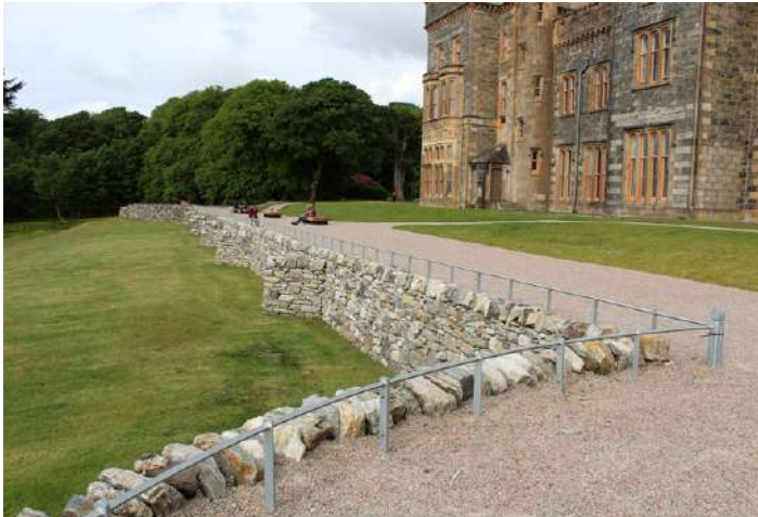
Crushed aggregate at Lewes Castle
