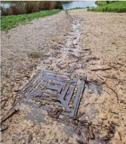
Blocked drains
