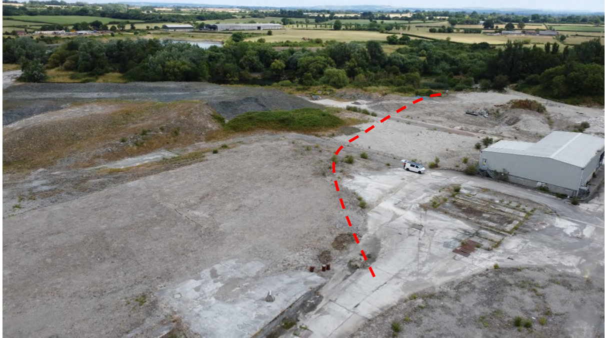
Plate 1 showing the site looking north east and approximate route of the works
