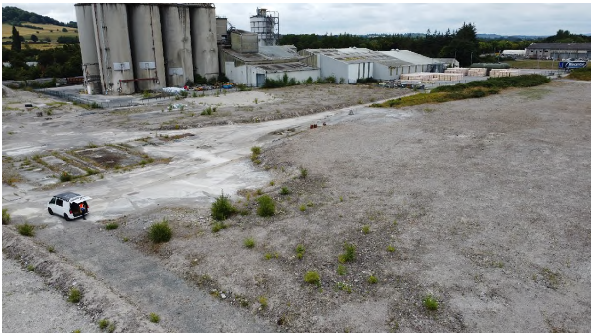
Plate 4 showing the bare ground of crushed concrete sealed surface zero rated in BNG criteria
