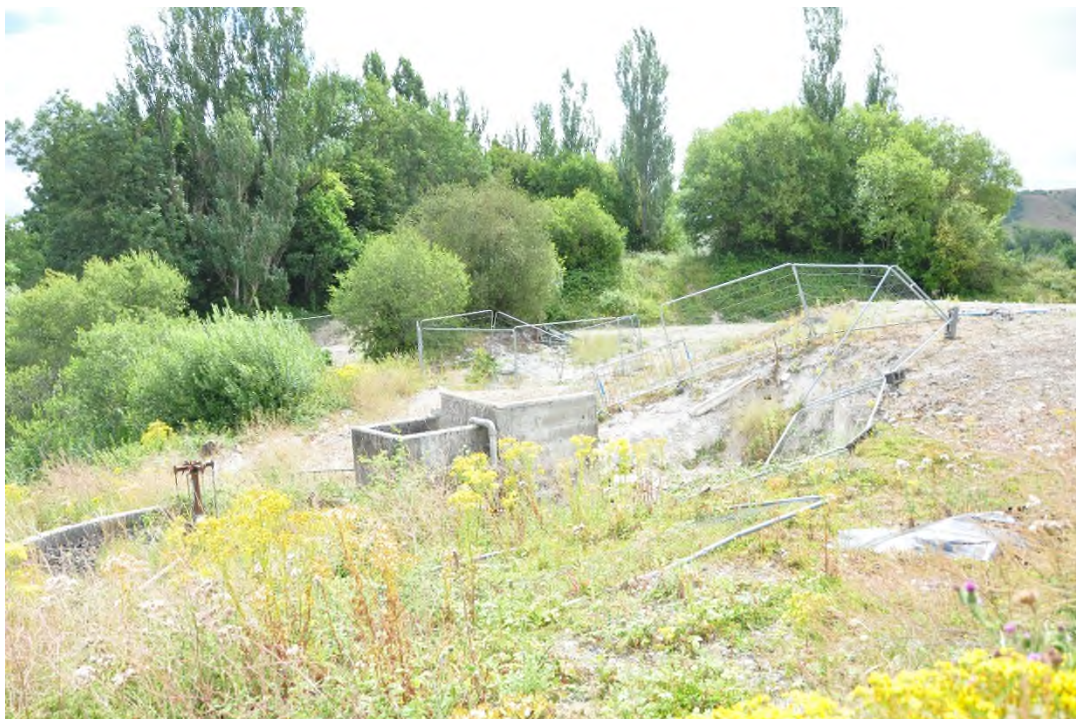
Plate 10 area of the proposed works at the STW
