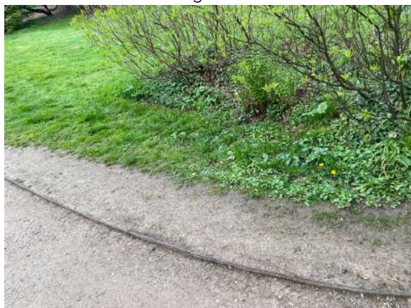
Plate 1: Erosion due to high traffic levels
