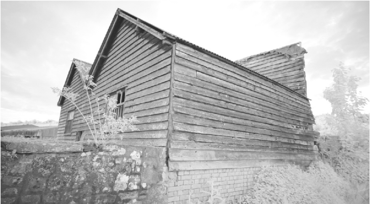
Figure 21 - Camera 2 Northwest and southwest elevations of Outbuilding 6. Start of survey 12/05/2025
