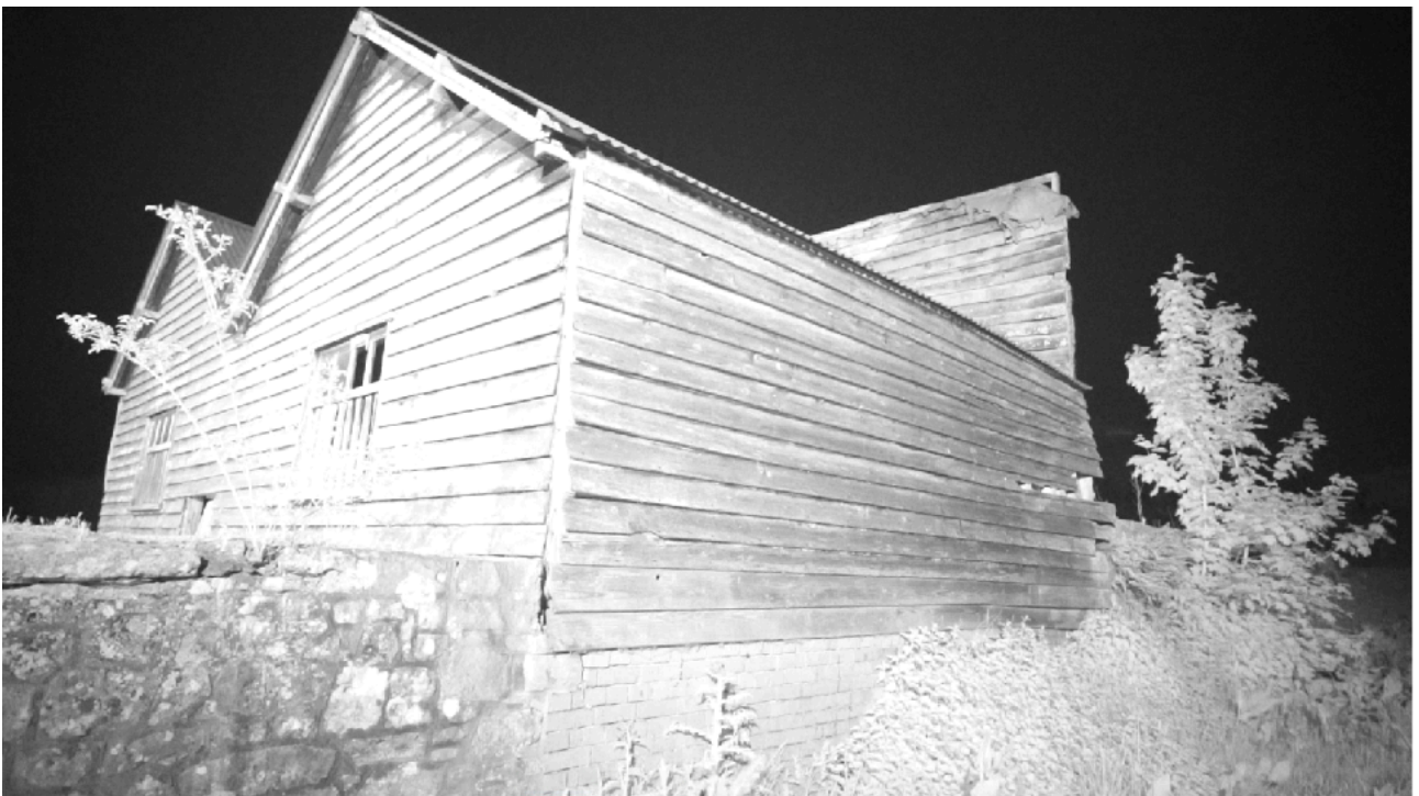
Figure 22 - Camera 2 Northwest and southwest elevations of Outbuilding 6. End of survey 12/05/2025
