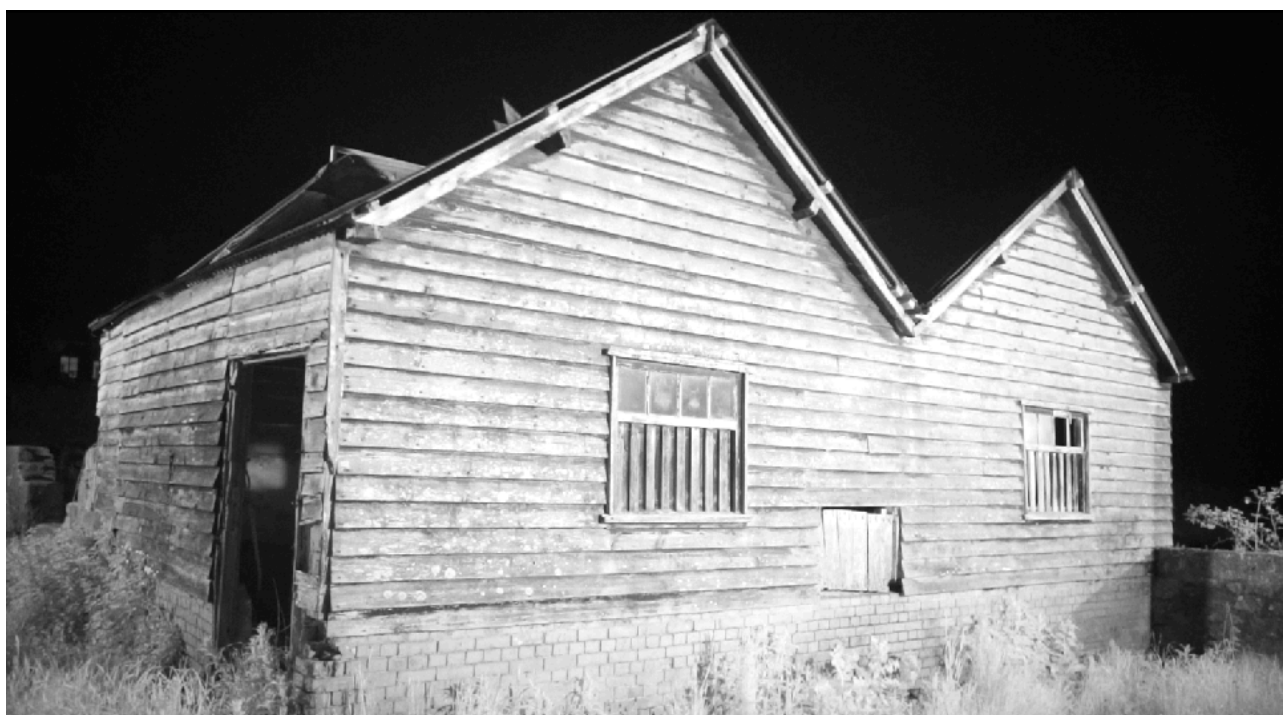
Figure 20 - Camera 1 Northeast and northwest elevations of Outbuilding 6. End of survey 12/05/2025
