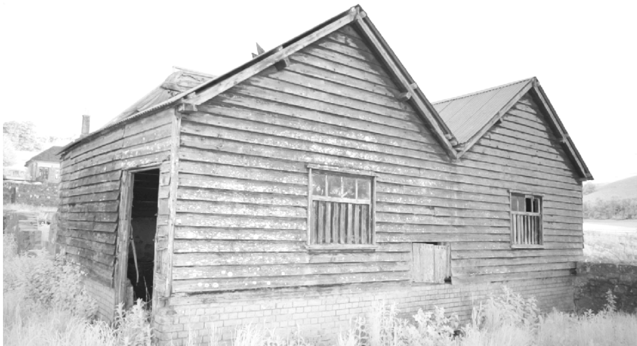
Figure 19 - Camera 1 Northeast and northwest elevations of Outbuilding 6. Start of survey 12/05/2025
