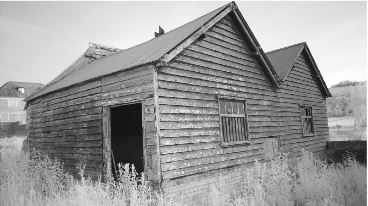
Figure 25 - Camera 1 Northeast and northwest elevations of Outbuilding 6. Start of survey 02/06/2025
