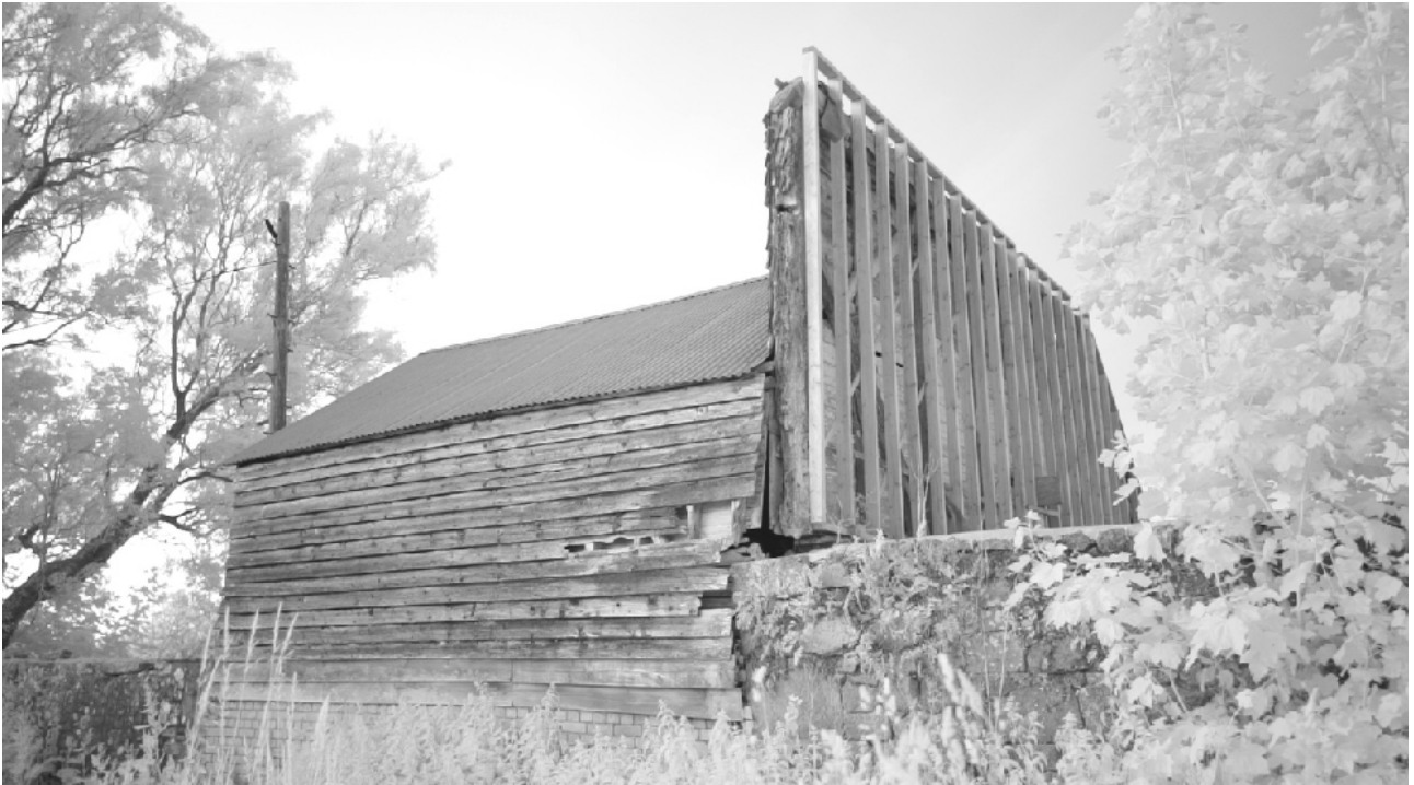
Figure 27 - Camera 2 Southwest and southeast elevations of Outbuilding 6. Start of survey 02/06/2025
