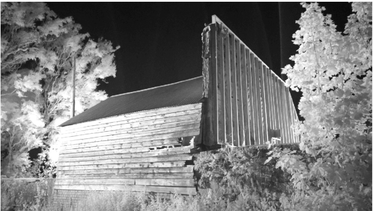
Figure 28 - Camera 2 Southwest and southeast elevations of Outbuilding 6. End of survey 02/06/2025
