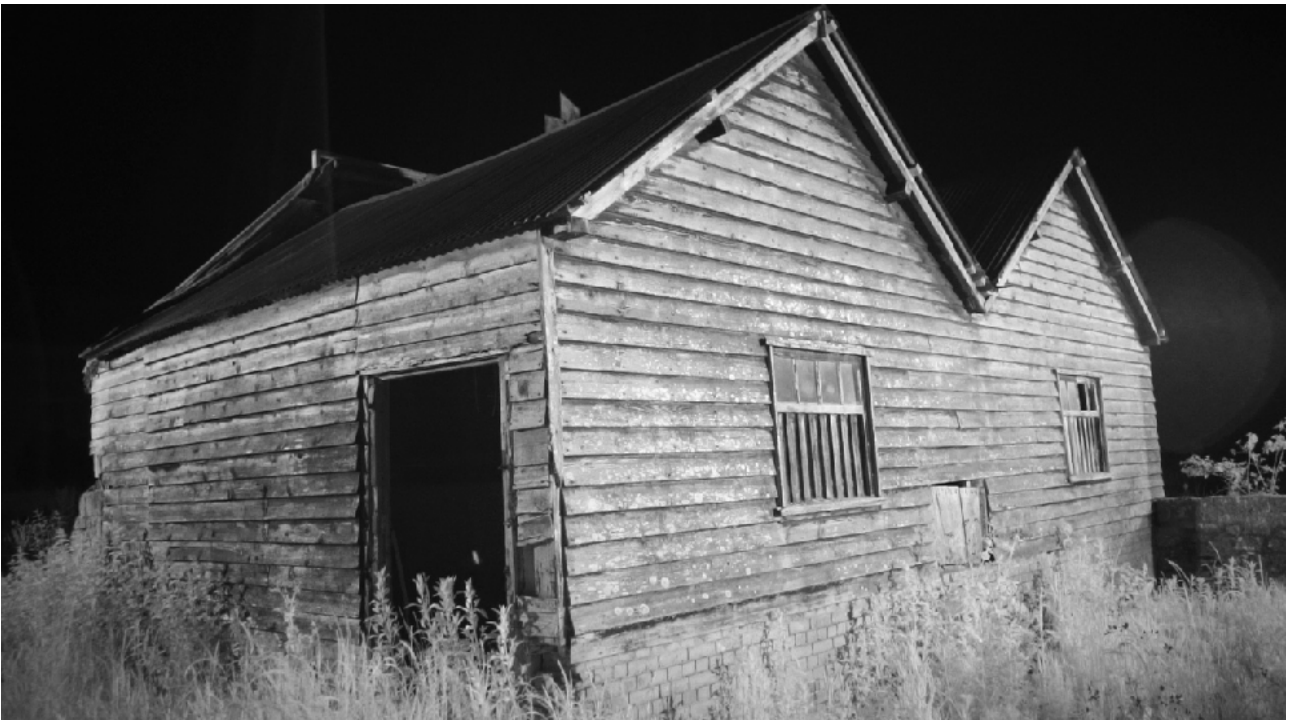
Figure 26 - Camera 1 Northeast and northwest elevations of Outbuilding 6. End of survey 02/06/2025
