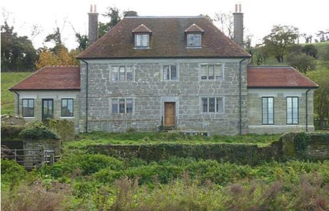
South front of Lower Bridmore Farmhouse
