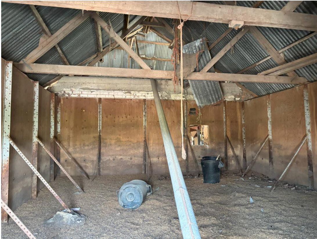
Interior of the north range of Barn 3 – internal boarded lining
