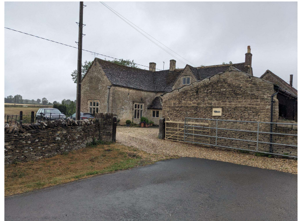
Access to Park Farm Dwelling
