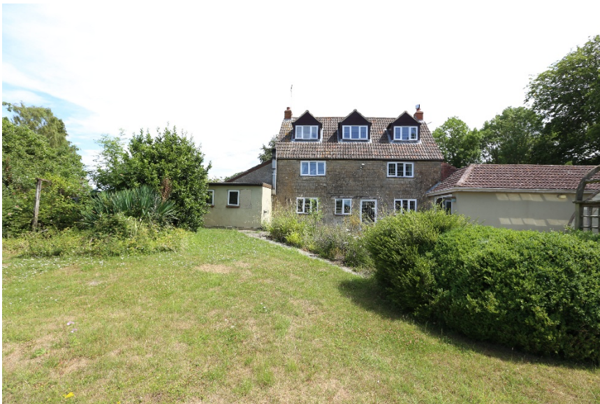
Bincknoll Cottage – View looking at the back of the property
