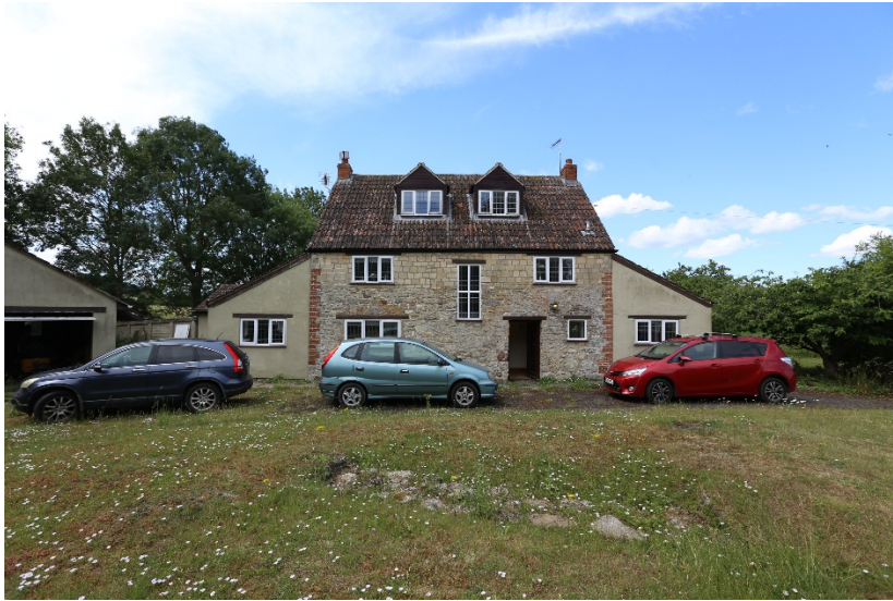
Bincknoll Cottage – View looking at the front of the property
