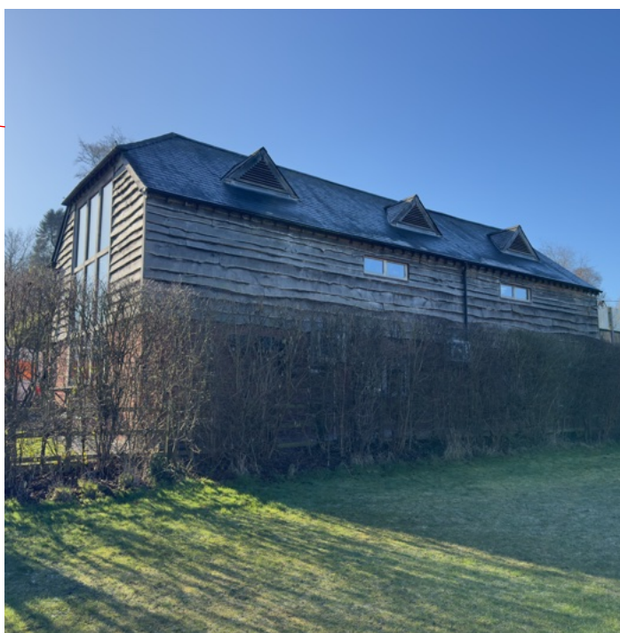
Figure 3 - The Farm Shops Northern elevation
