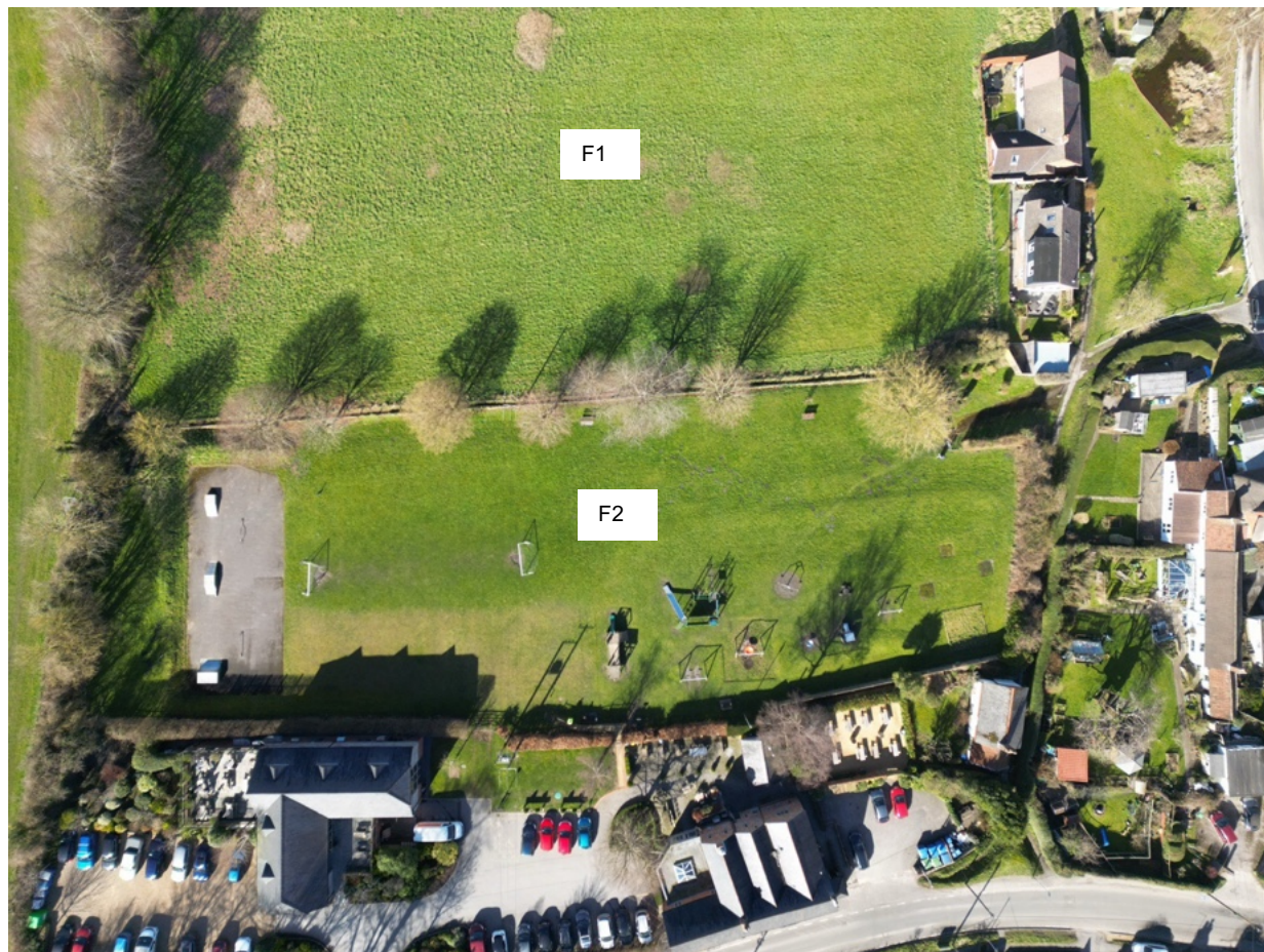
Figure 1: Aerial view of most of the Site
