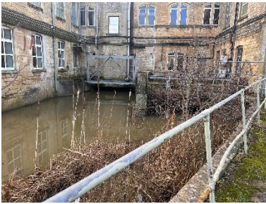
Figure 2-9: Sluices under building
