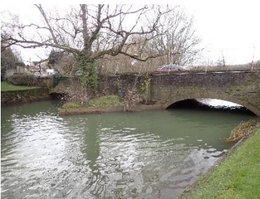
Figure 2-11: Weston Cut Bridge
