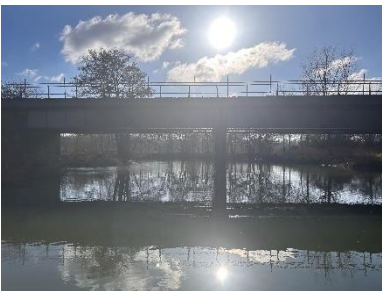
Figure 2-3: Railway Bridge Wessex Mainline
