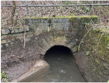
Figure 2-5: Culvert 0, Mason Arch Culvert
