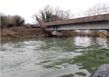
Figure 2-2: Railway Bridge Weymouth Line
