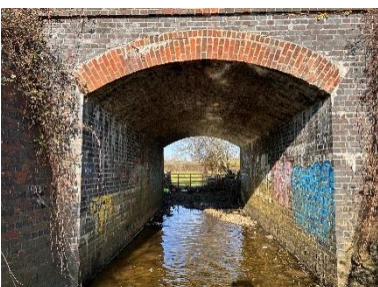
Figure 2-8: Culvert 2, Mason Arch Culvert
