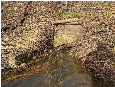
Figure 2-6: Culvert 1, Mason Arch Culvert
