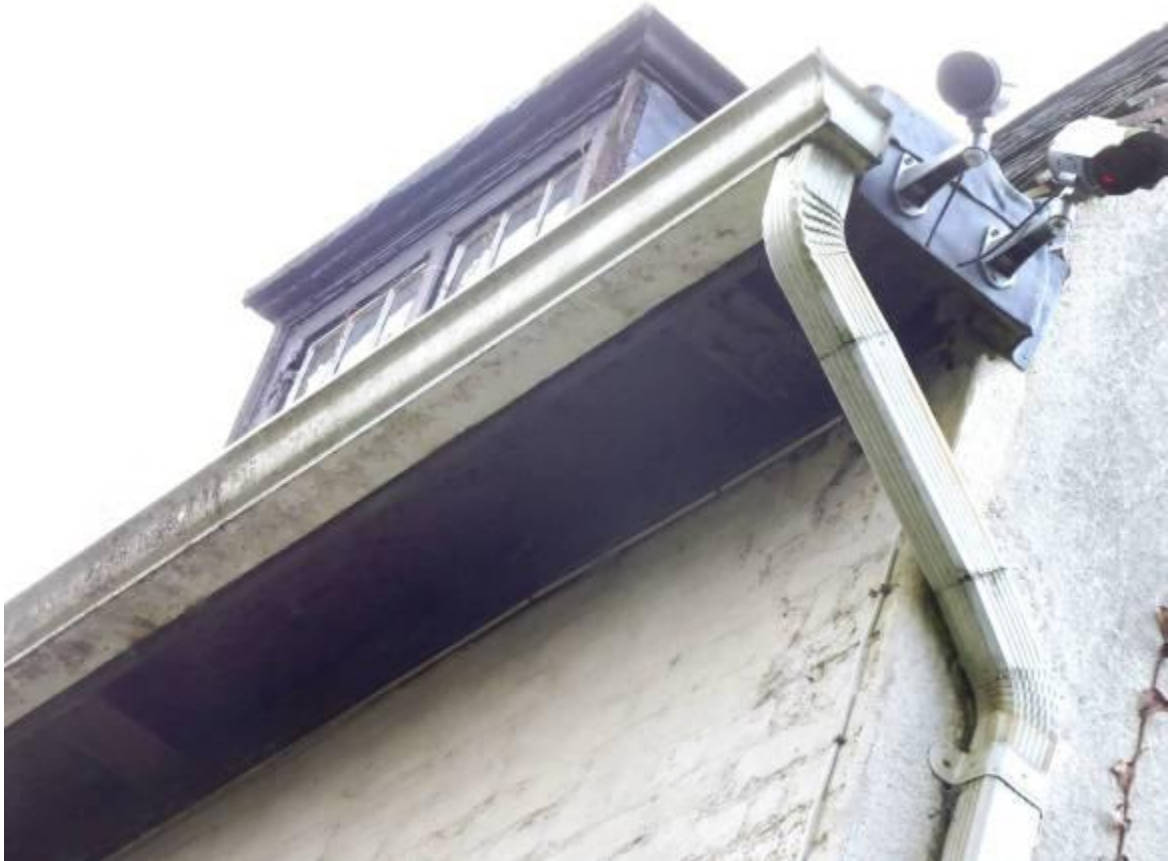
Fig 3.4.1: Main eaves structure
