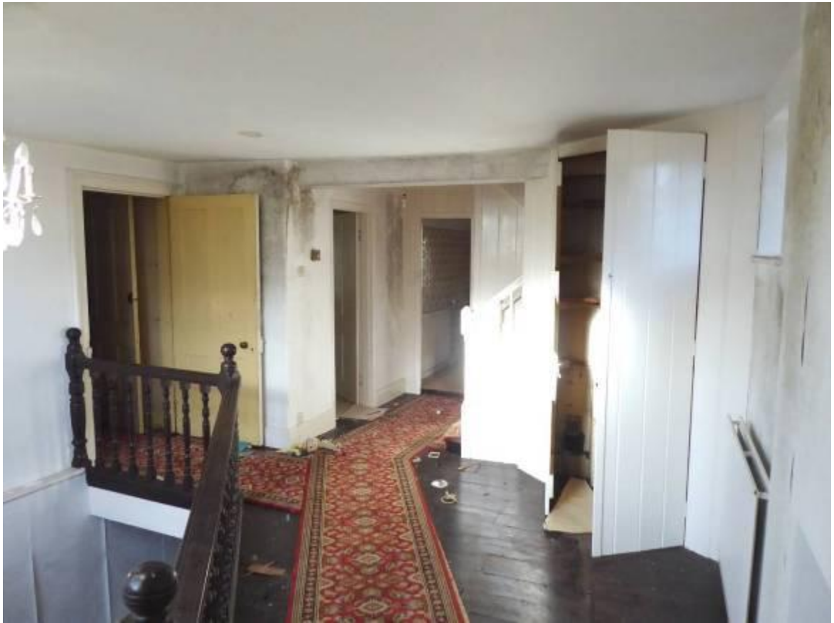
Fig 4.15: First floor landing
