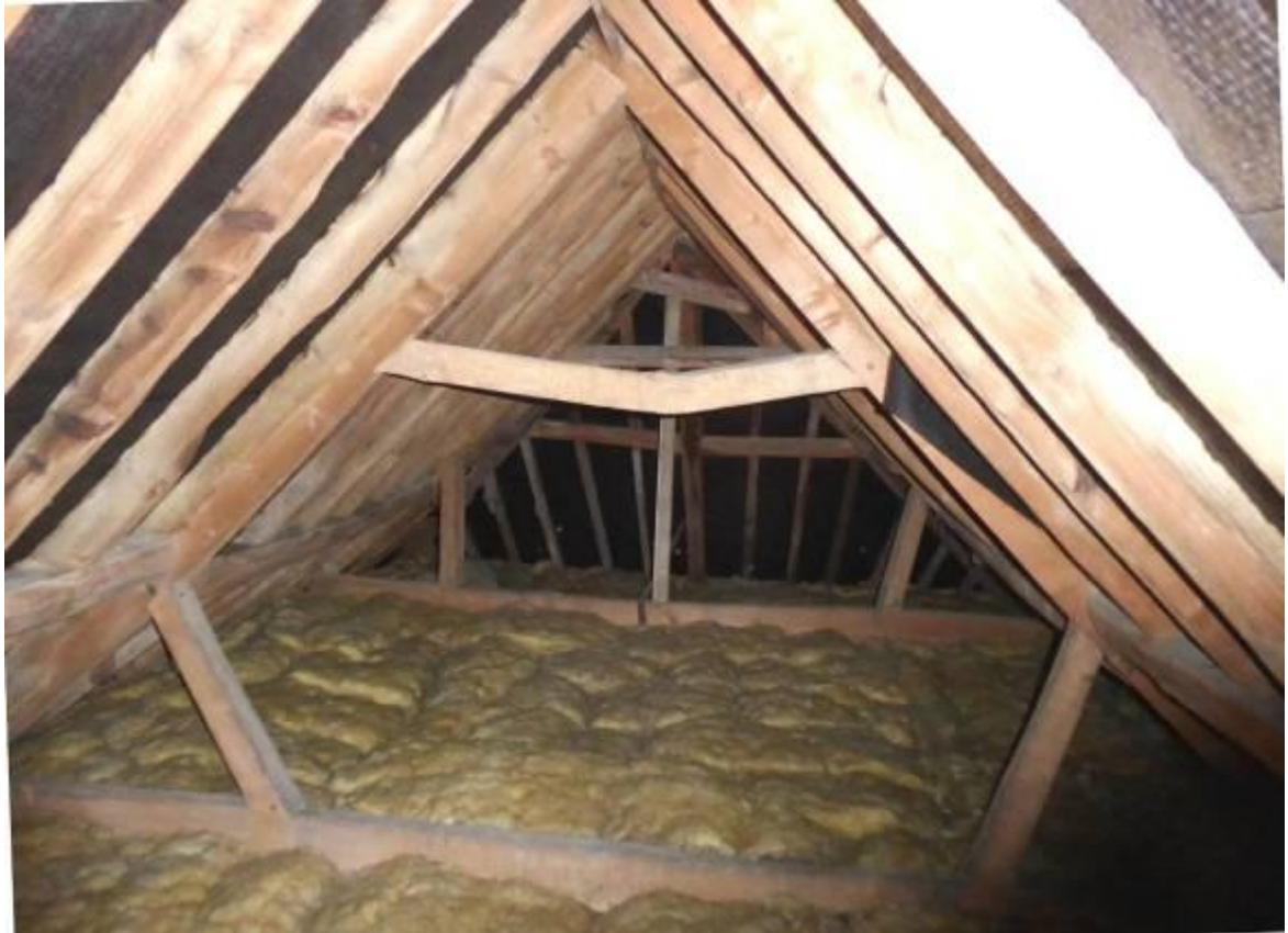
Fig 4.33: Two storey roof
