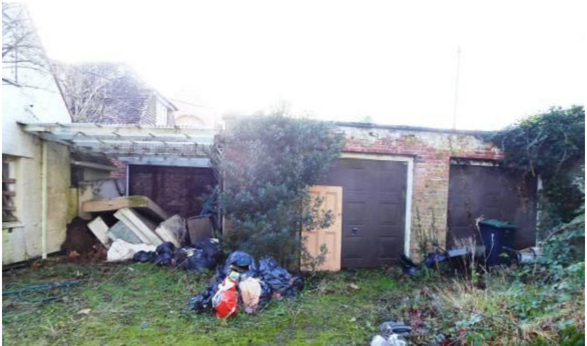
Fig 2.2.3: Garage block in southwest corner of site
