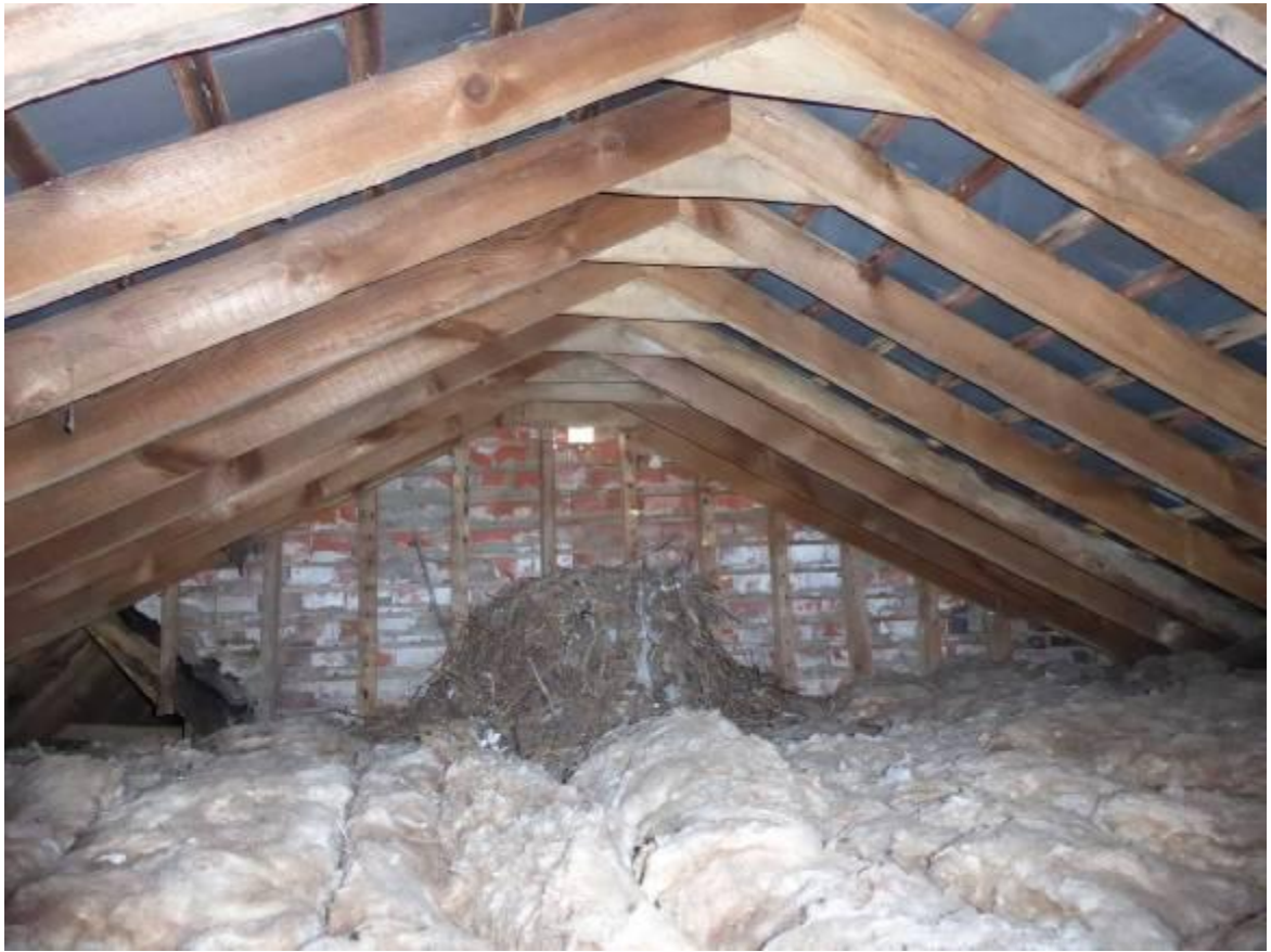
Fig 4.32: Three storey roof looking to east gable
