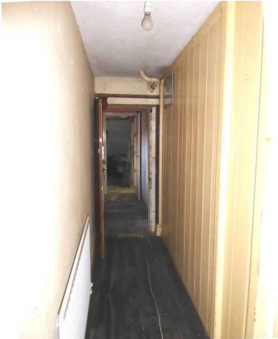
Fig 4.16: Service block first floor access corridor
