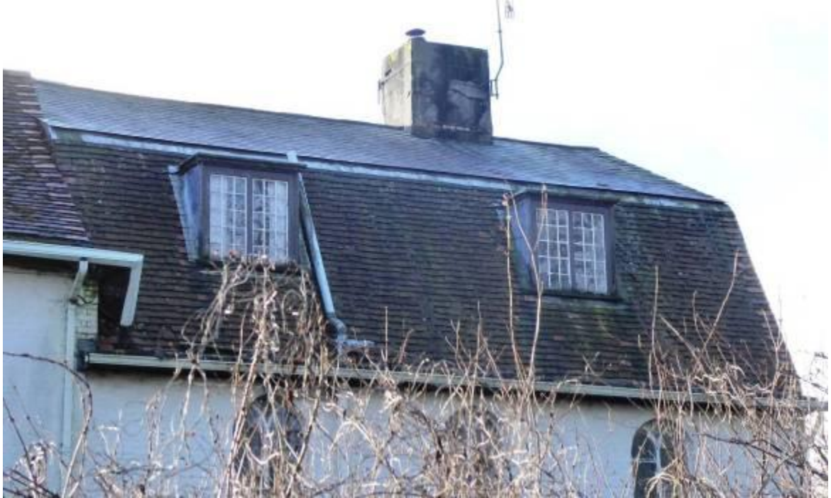
Fig 3.1.1: Mansard roof north side
