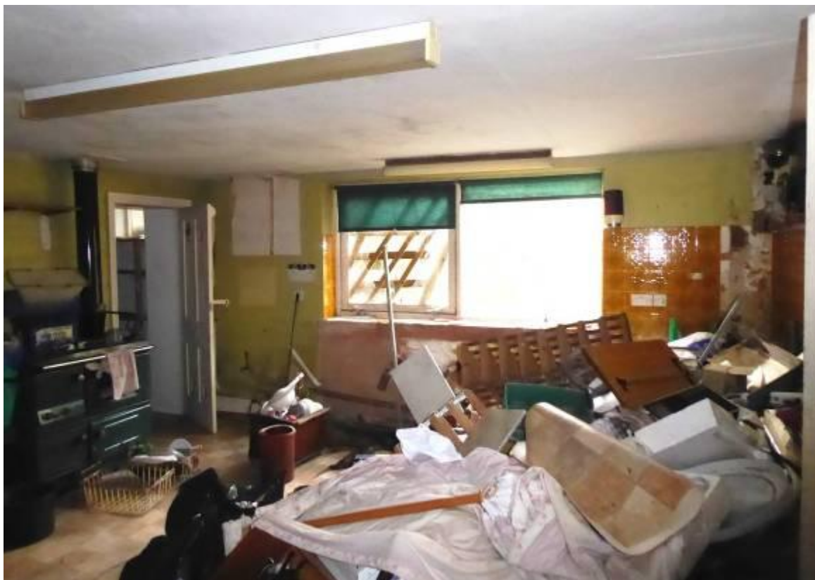
Fig 4.12: Service block ground floor west room
