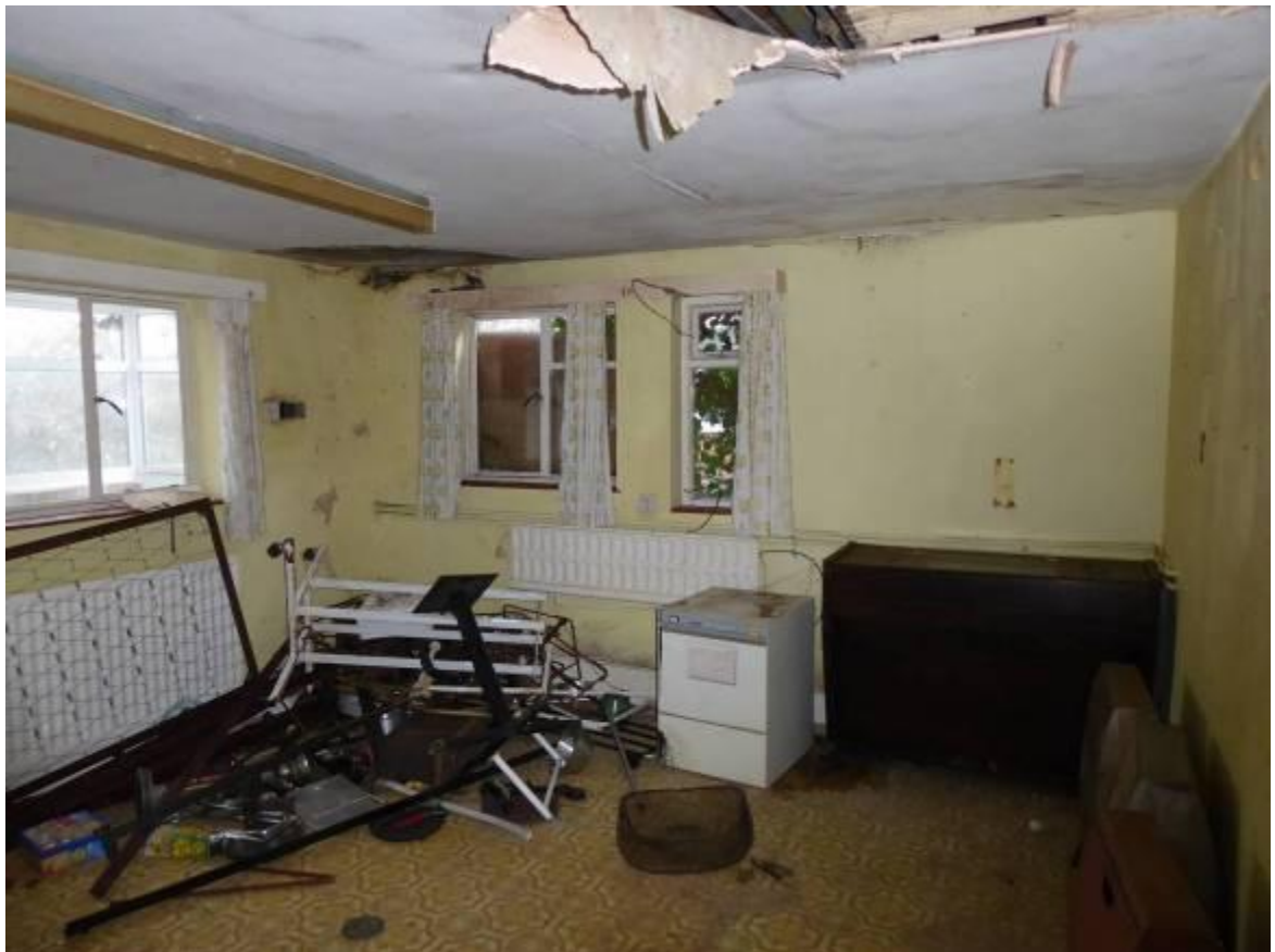
Fig 4.11: Service block ground floor east room
