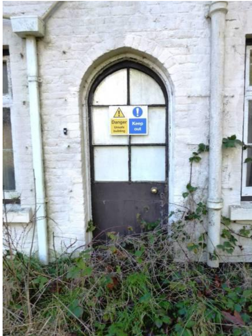
Fig 3.7.3: Entrance hall door
