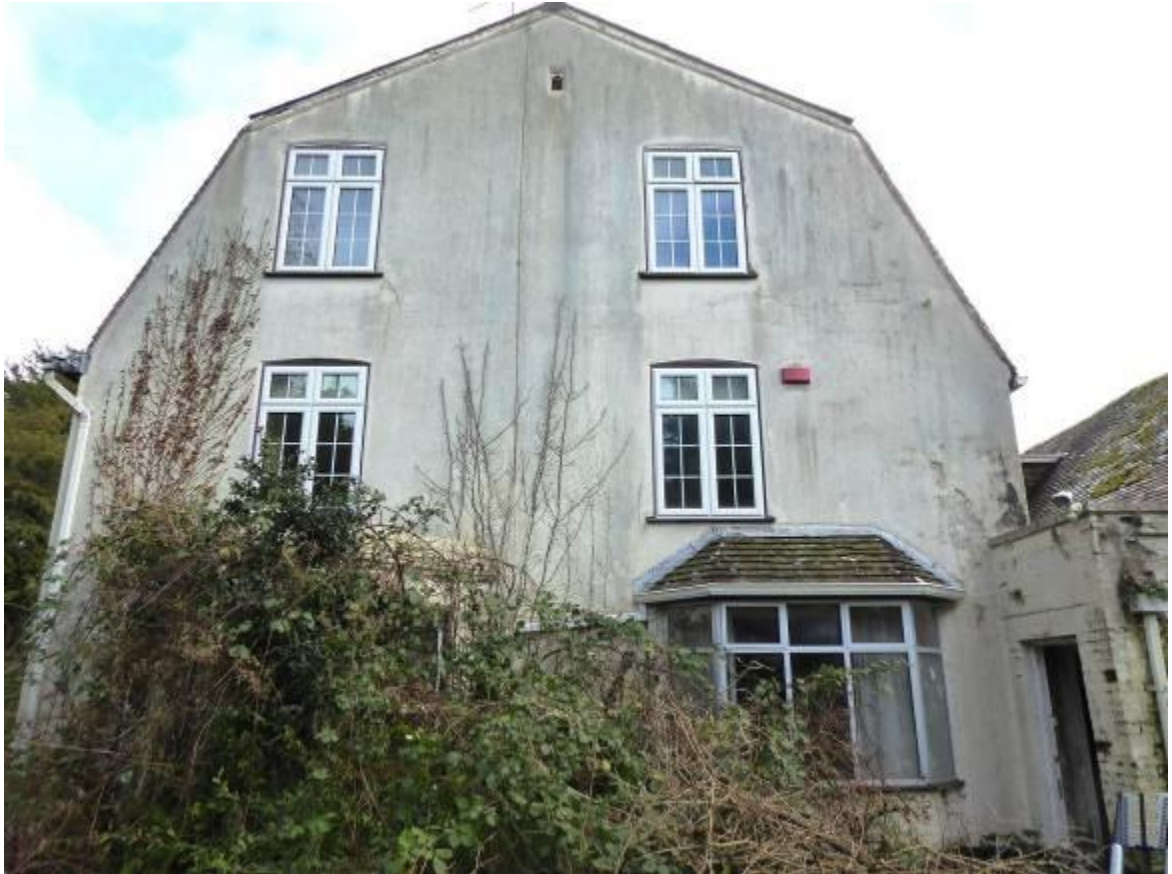
Fig 3.5.1: West elevation of main house
