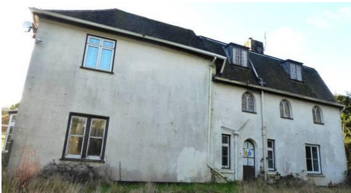
Fig 3.6.5: North side east and west windows
