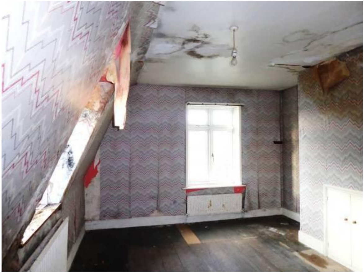
Fig 4.29: Second floor southwest bedroom
