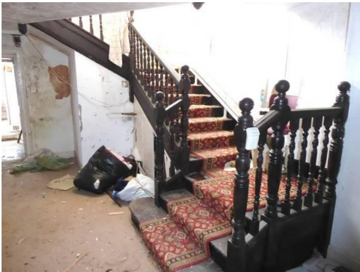
Fig 4.14: Stairs from ground to first floor
