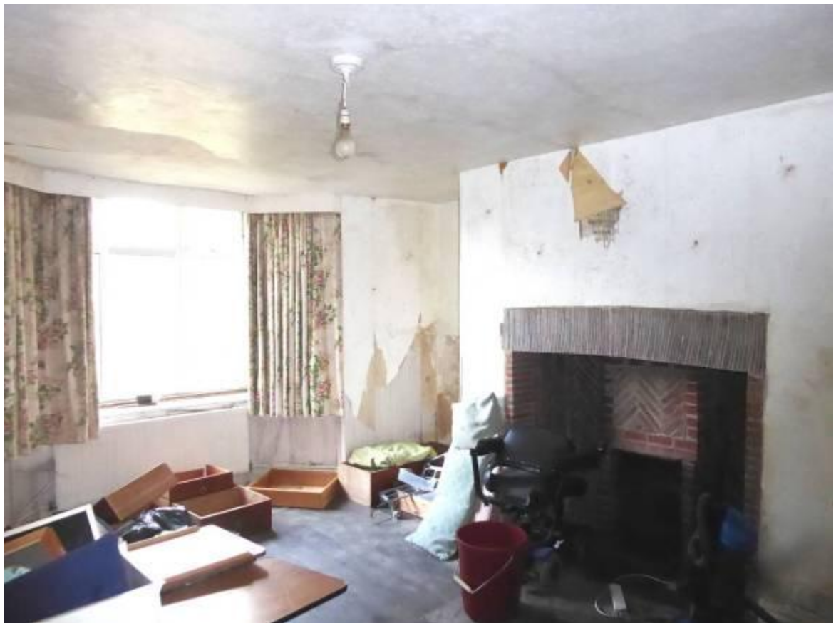
Fig 4.7: Ground floor southwest room
