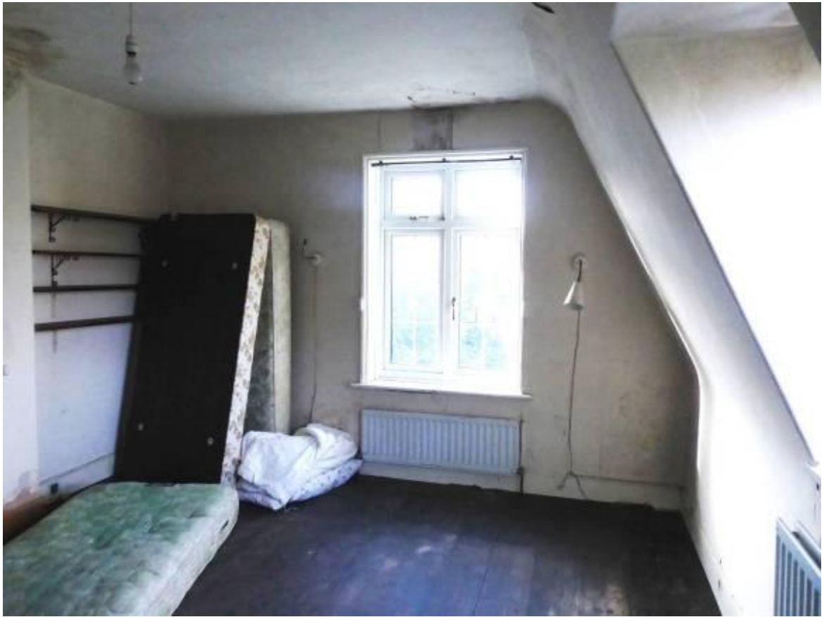
Fig 4.30: Second floor northwest room
