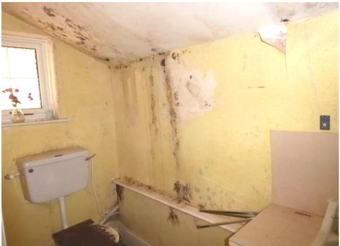
Fig 4.6: Ground floor cloakroom
