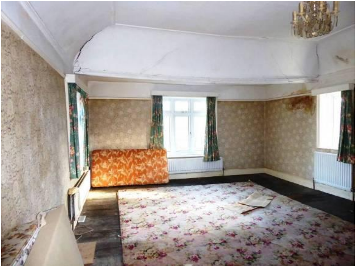
Fig 4.21: First floor east bedroom
