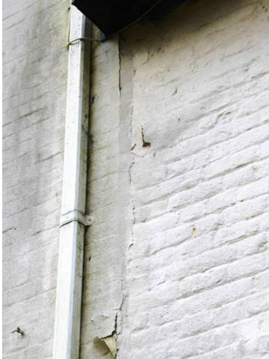
Fig 3.5.6: North wall construction joint between west and east parts
