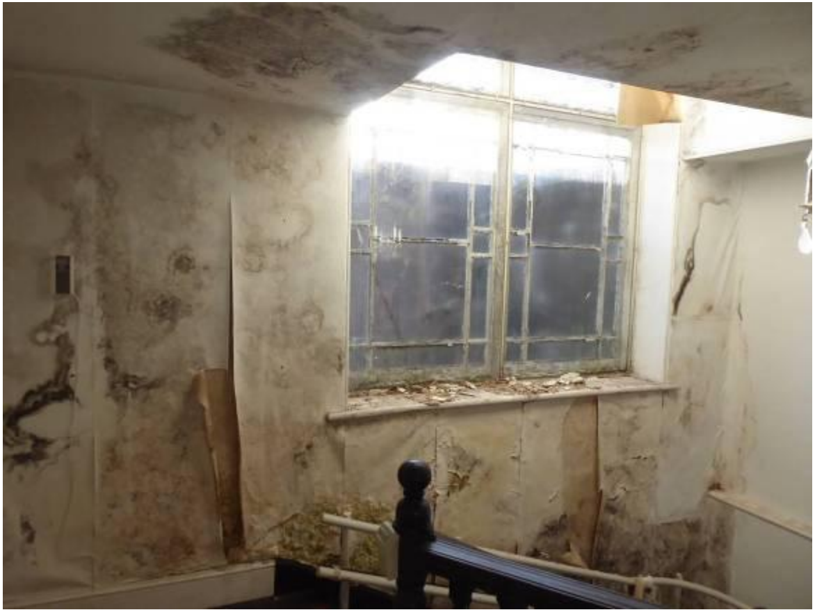
Fig 4.14.3: First floor landing south wall
