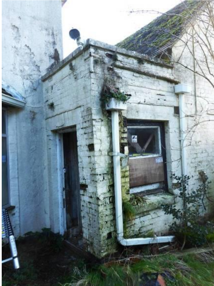
Fig 3.5.14: Northwest corner of service block
