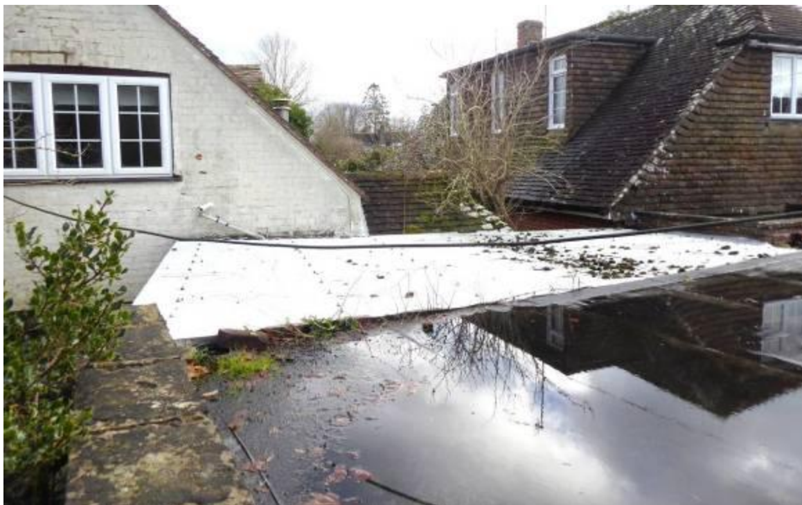
Fig 3.2.1: Garage and car port roof
