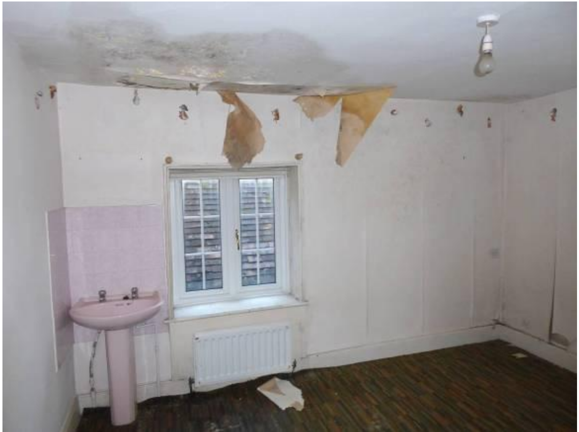
Fig 4.17: First floor southwest room
