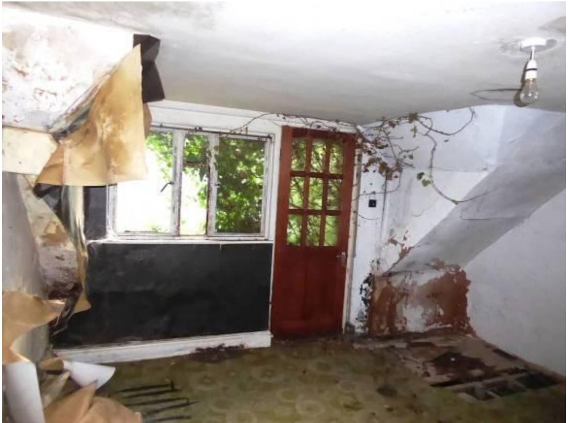
Fig 4.23: Service block first floor east room
