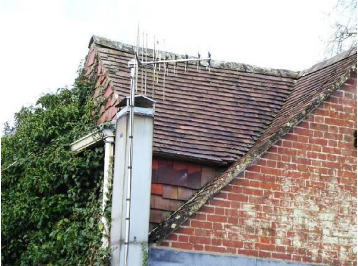
Fig 3.1.9: Service block roof
