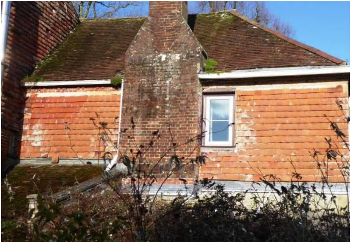
Fig 3.5.11: East wall of two storey part
