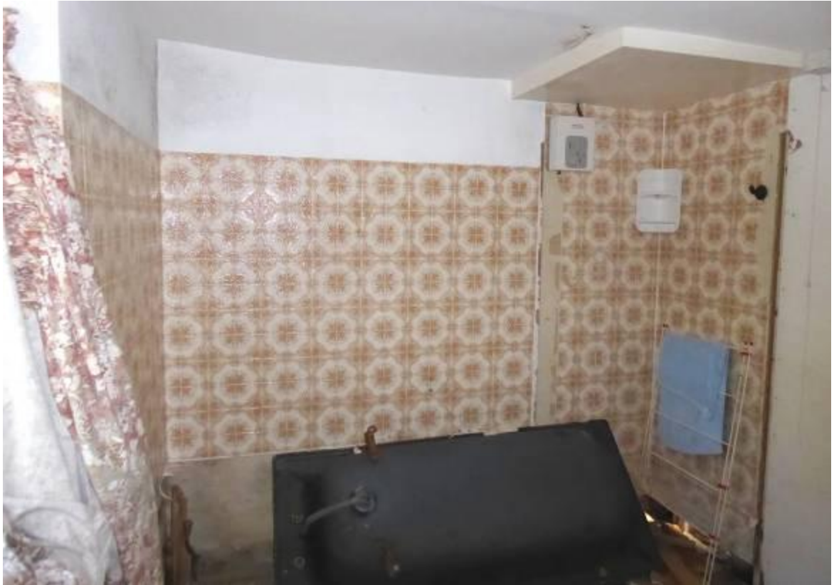
Fig 4.19: First floor Bathroom
