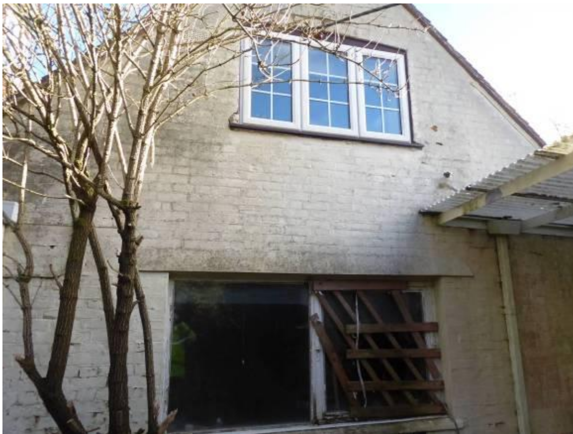
Fig 3.5.14: Service block west windows
