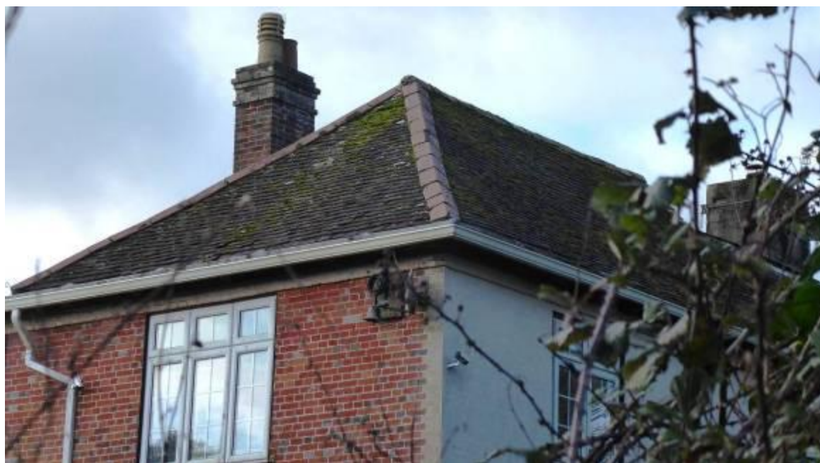
Fig 3.1.6: East two storey roof
