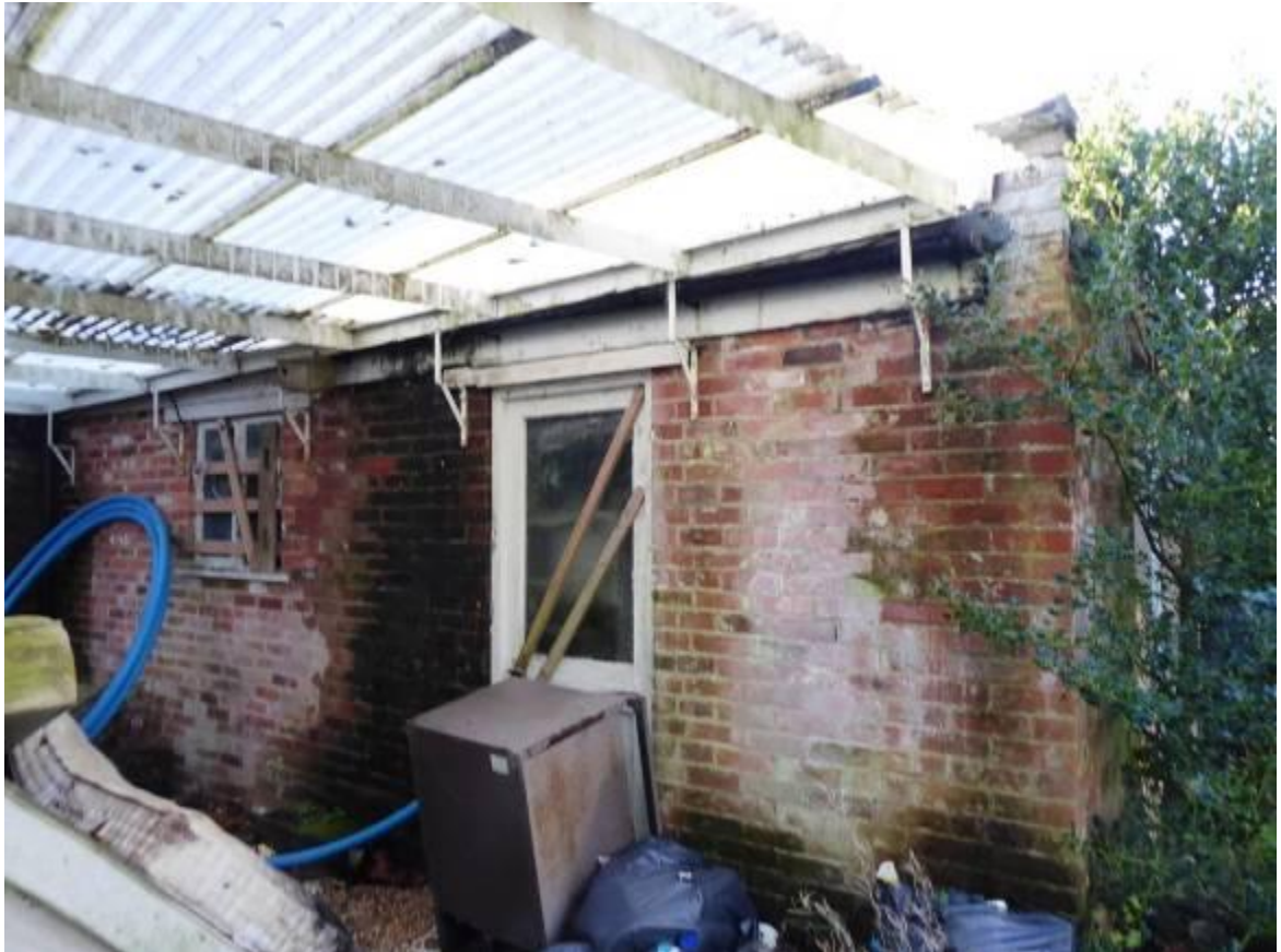
Fig 3.5.16: East wall of garage
