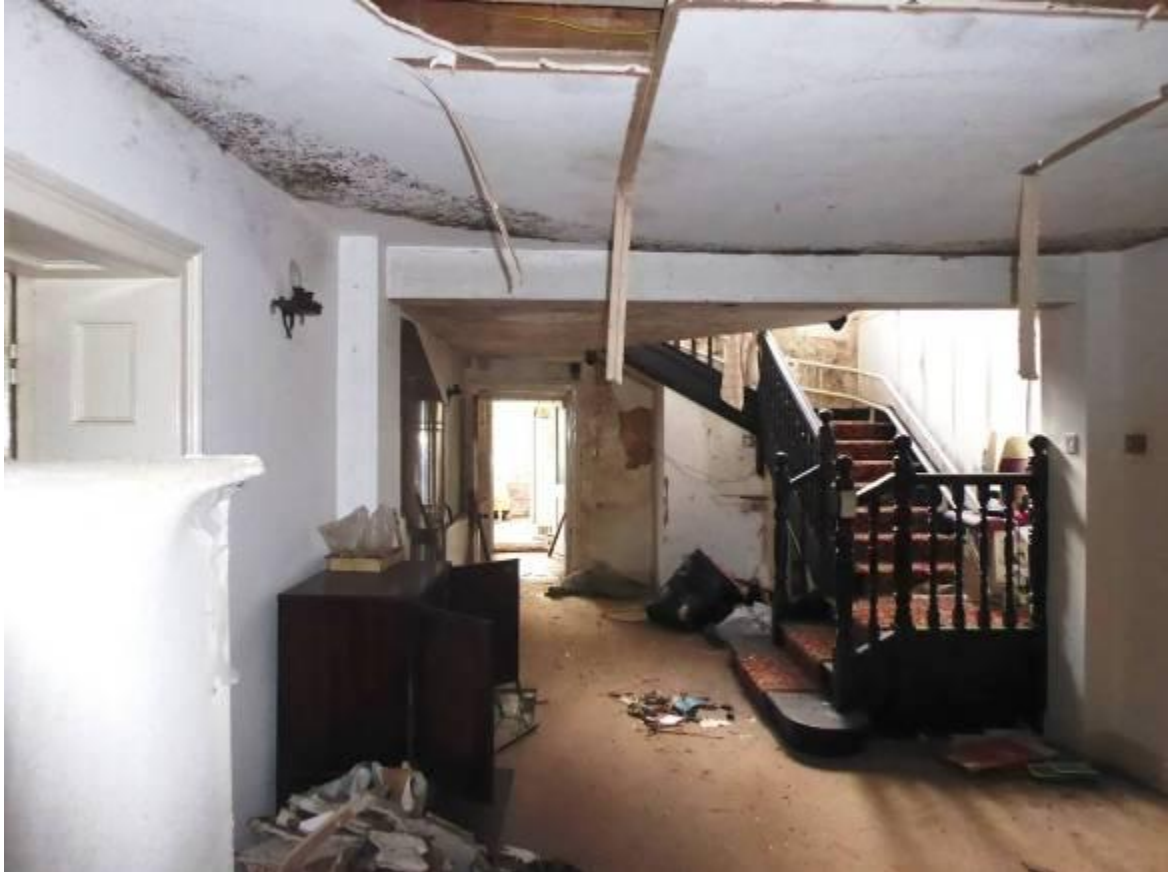
Fig 4.1: Entrance Hall, looking to rear
