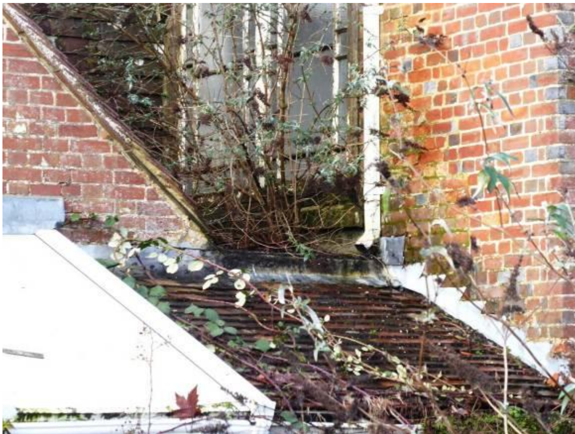
Fig 3.1.13: Failed roof
