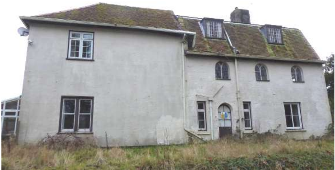
Fig 7.2.6: Old vicarage from the north
