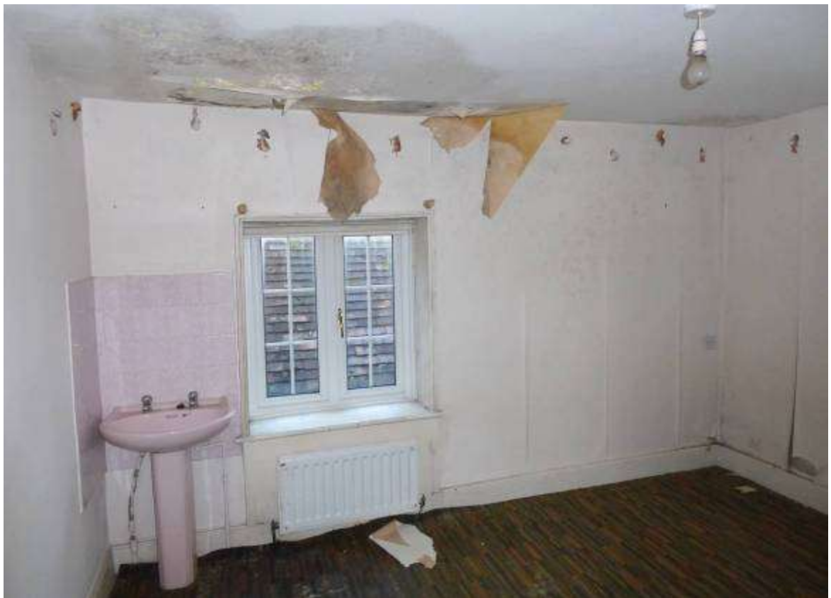
Fig 4.16: First floor southwest room
