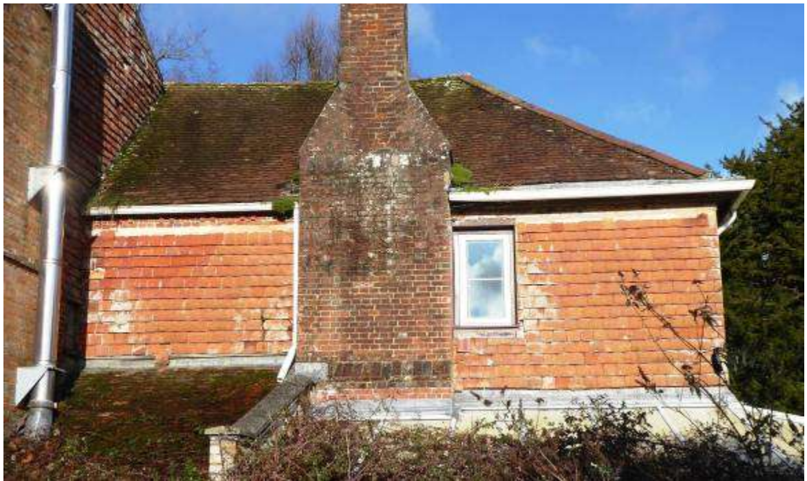
Fig 3.5.7: South side of east block
