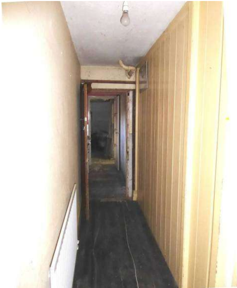
Fig 4.15: Service block first floor access corridor
