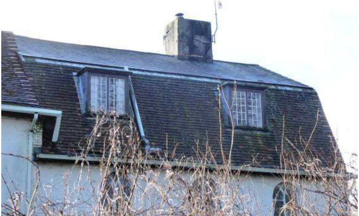
Fig 3.1.1: Mansard roof north side with dormer windows
