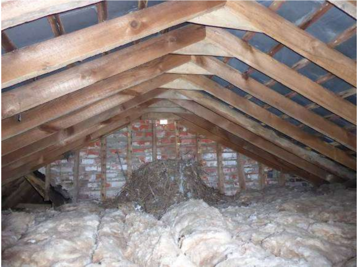
Fig 4.32: Three storey roof looking to east gable
