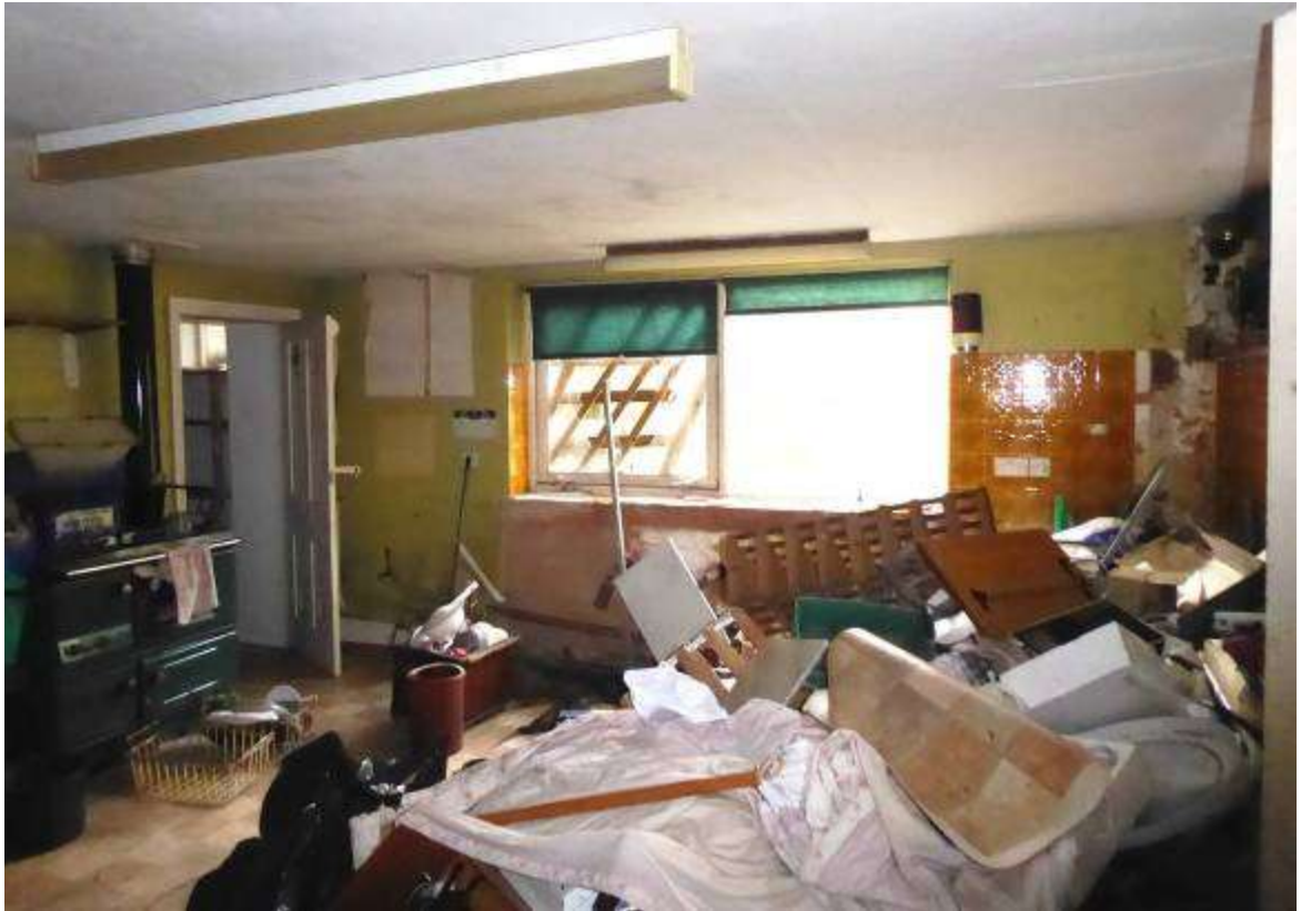
Fig 4.11: Service block ground floor west room
