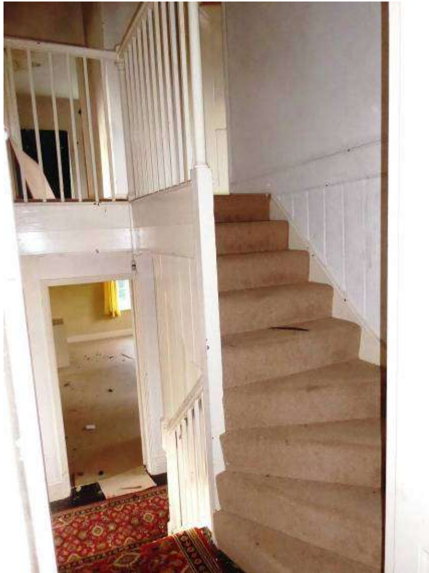
Fig 4.25: Stairs from first to second floor
