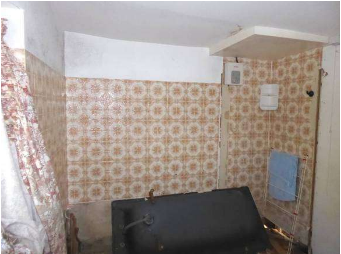
Fig 4.18: First floor bathroom
