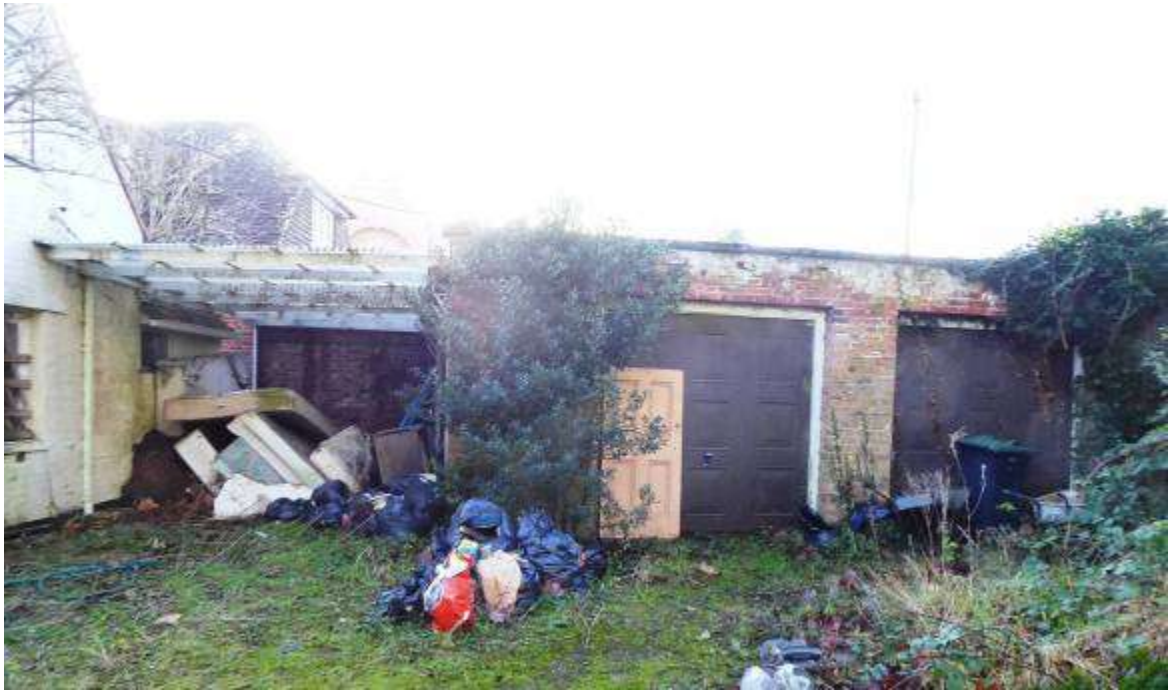
Fig 2.2.3: Garage block in southwest corner of site
