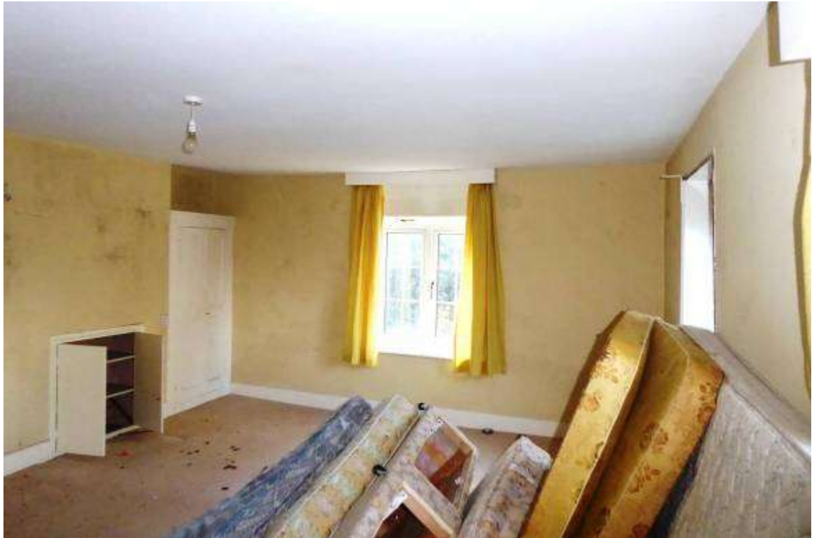
Fig 4.17: First floor northwest room
