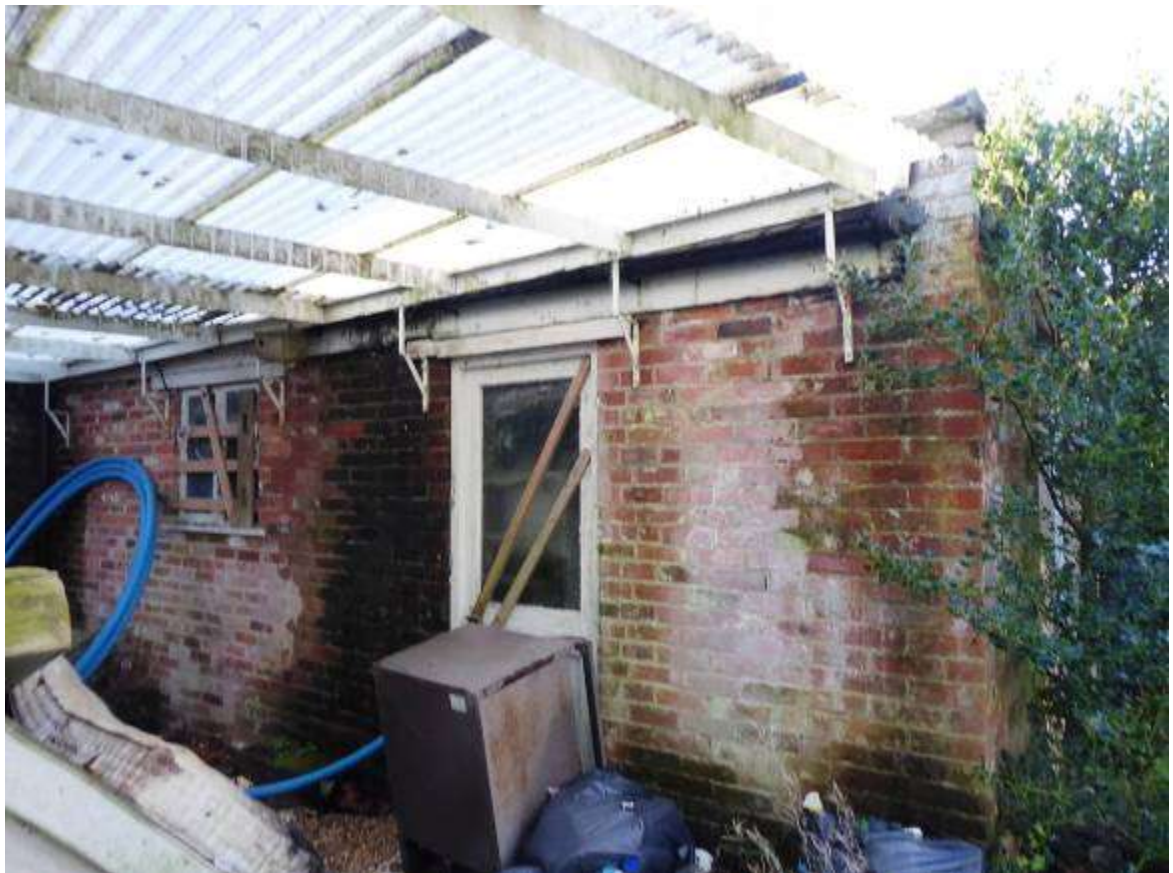
Fig 3.5.16: East wall of garage
