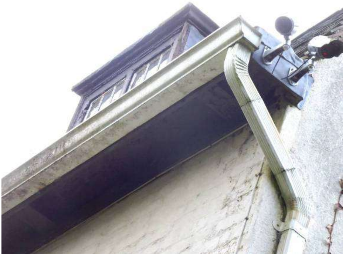
Fig 3.4.1: Main eaves structure
