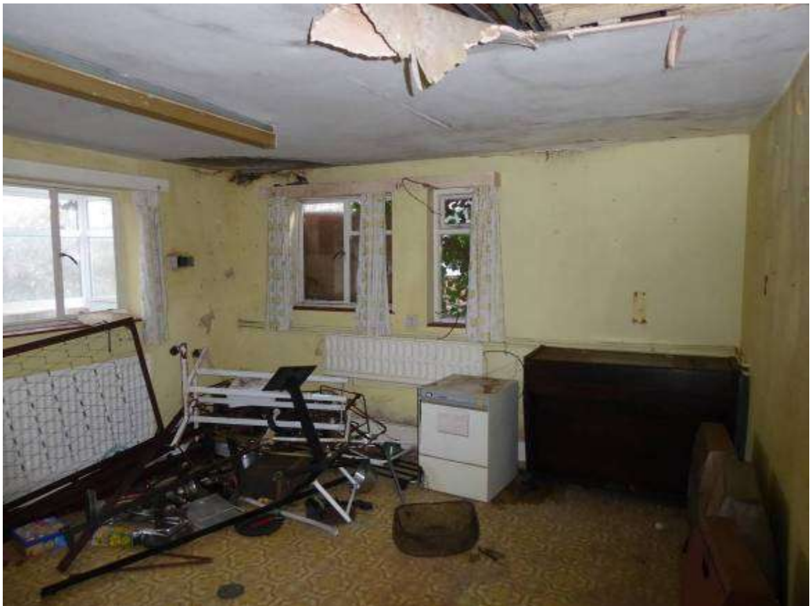
Fig 4.10: Service block ground floor east room
