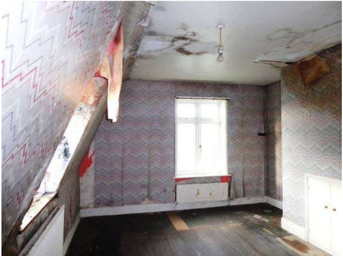
Fig 4.28: Second floor southwest bedroom
