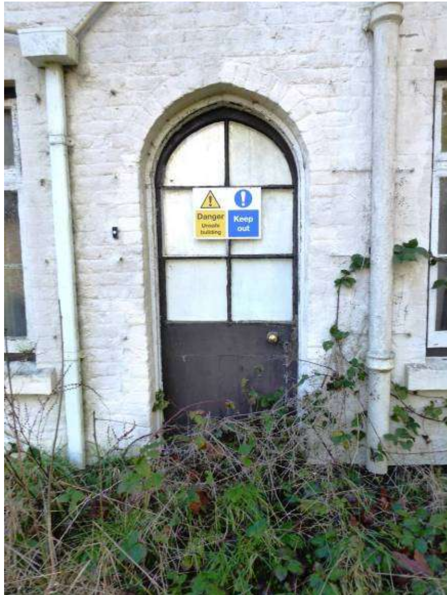
Fig 3.7.3: Entrance hall door
