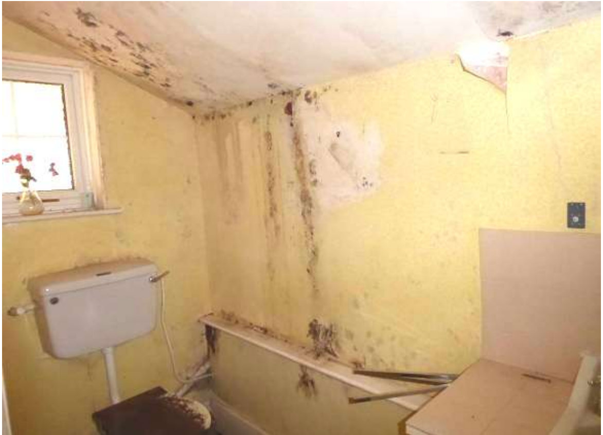
Fig 4.6: Ground floor cloakroom
