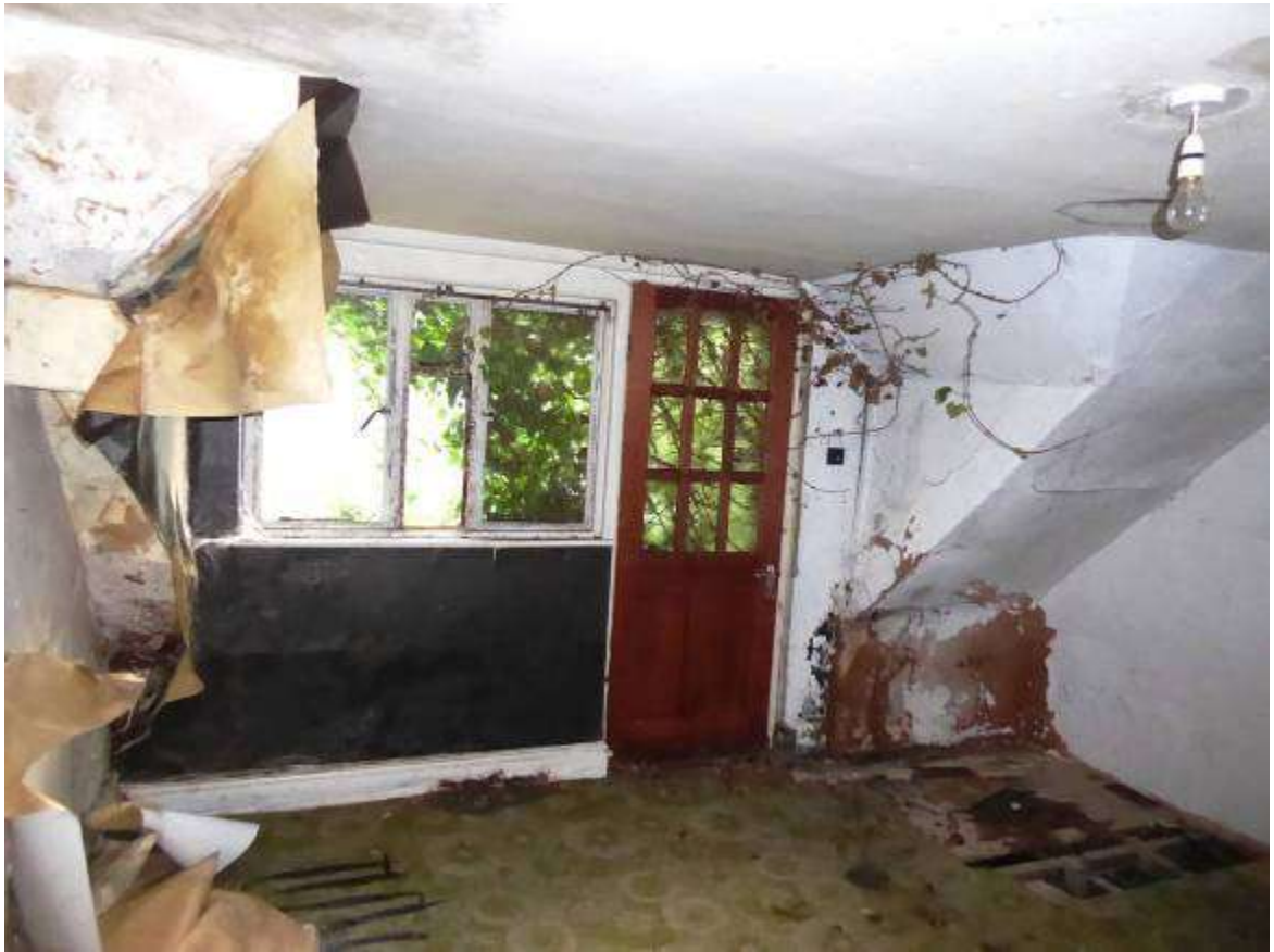
Fig 4.22: Service block first floor east room
