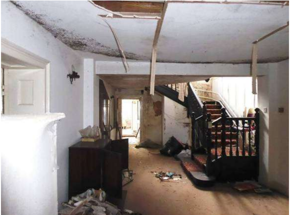
Fig 4.1: Entrance Hall, looking to rear
