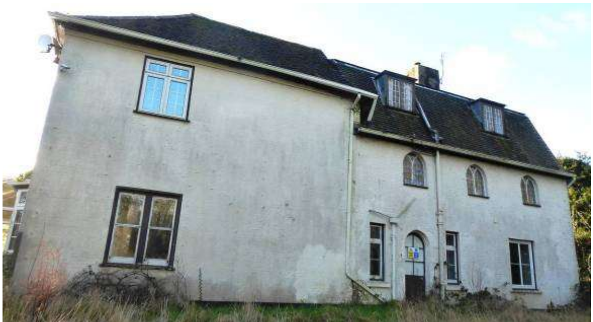
Fig 3.6.2: North side windows
