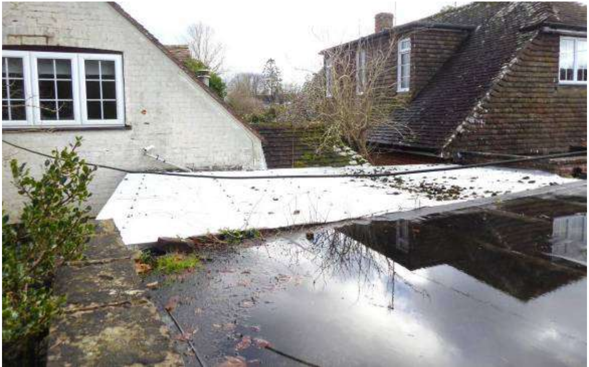
Fig 3.2.1: Garage and car port roof
