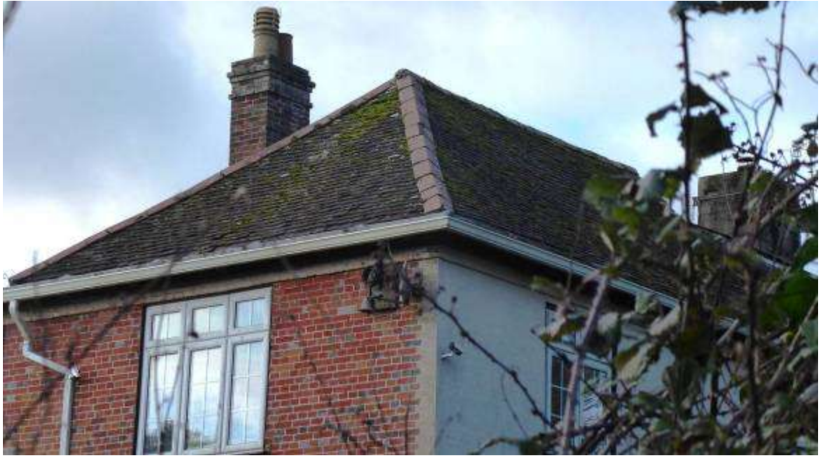
Fig 3.1.5: East two storey roof
