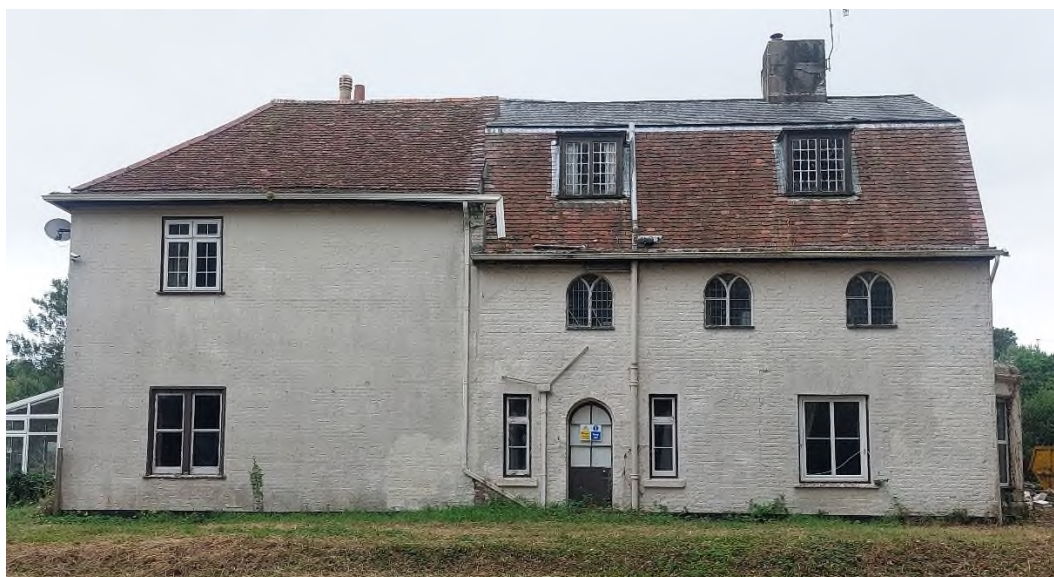
Figure 1 North elevation of The Old Vicarage showing the c.1800 three-bay house to the right, the 19 th century addition to the left and the c.1900 mansard roof over the earlier phase of the house.
