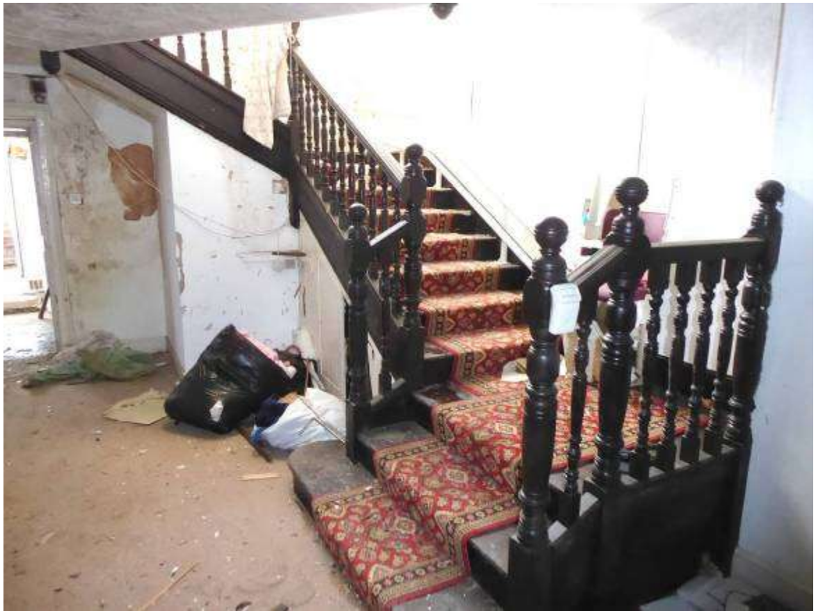
Fig 4.13: Stairs from ground to first floor
