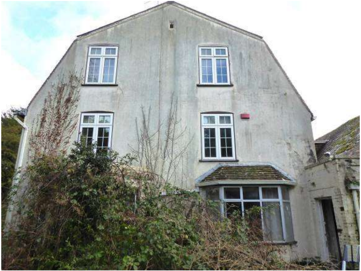
Fig 3.5.1: West elevation of main house
